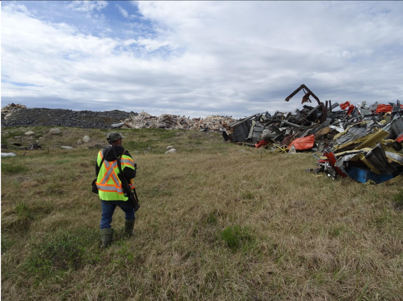
Description: Temporary Storage of Demolished Debris – View 5
