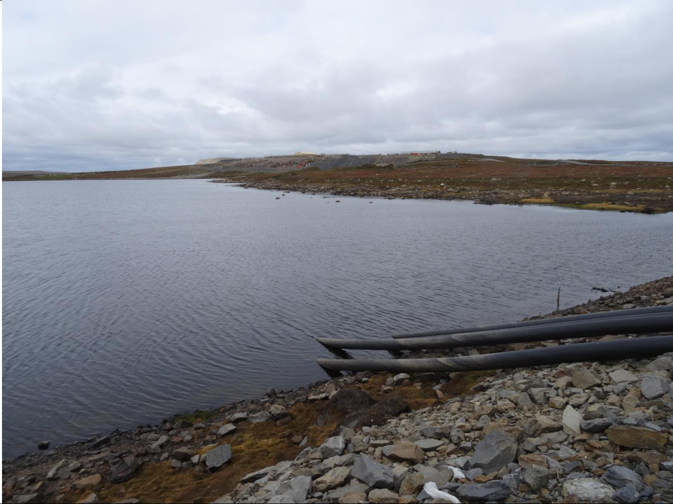
Description: Lower Sewage Lagoon
