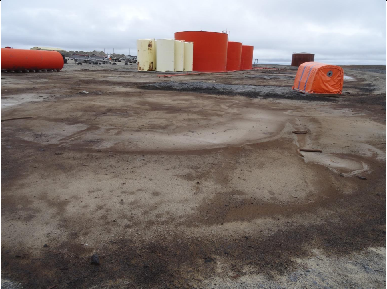
Description: Main Tank Farm – View 1
