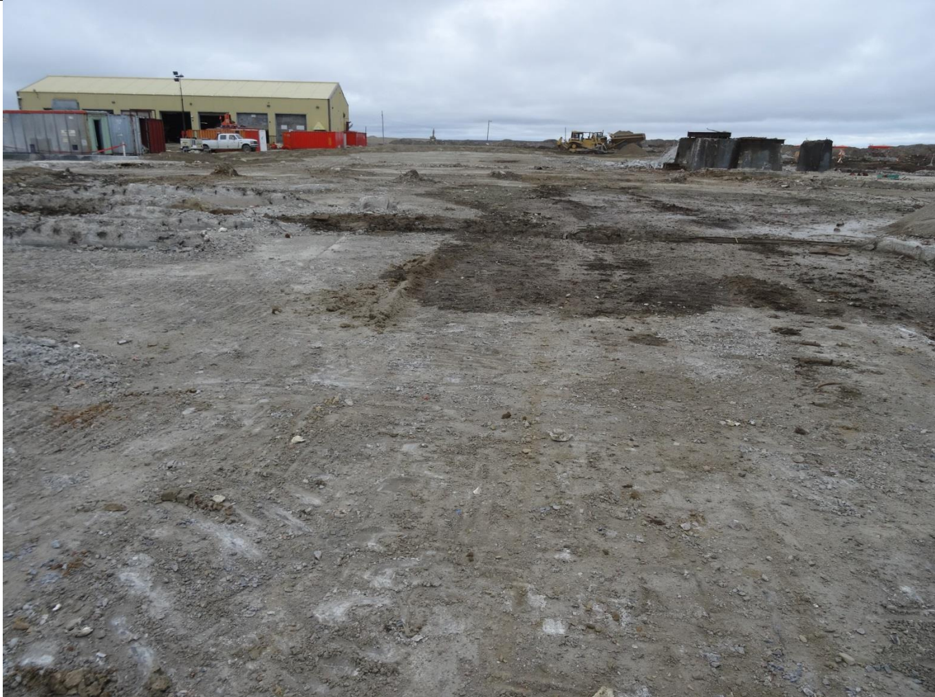
Description: #11 Mill, View 1 – Large Concrete Blocks in Top Right of Photo to be Removed – All other Debris Removed into Land Fill
