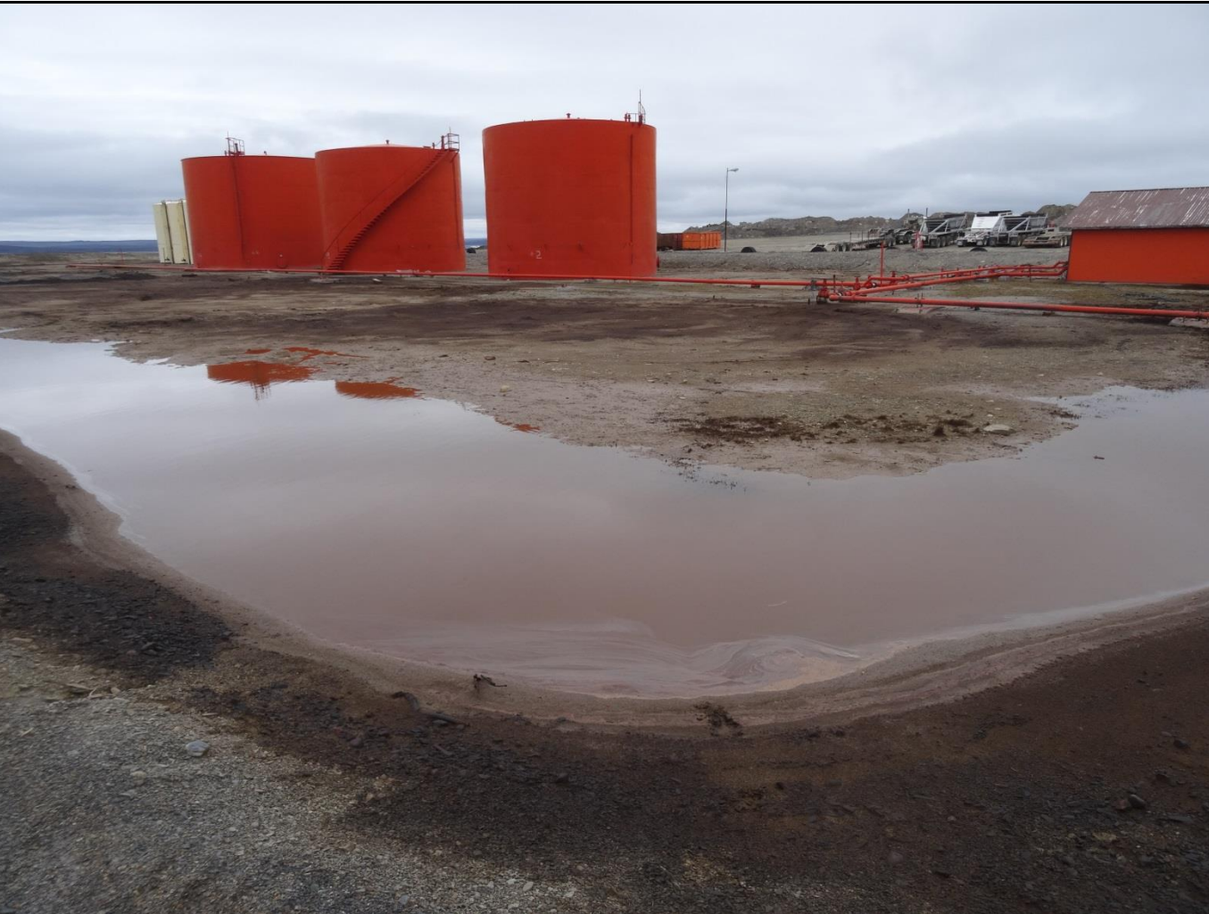
Description: Main Tank Farm – View 2
