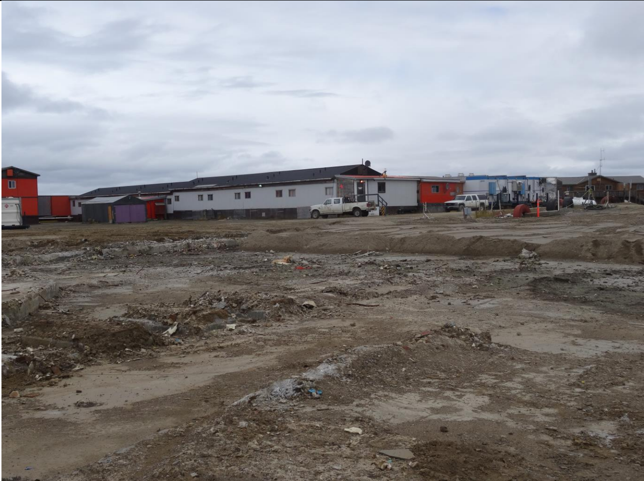
Description: 1300 Dorm Complex – White Building
