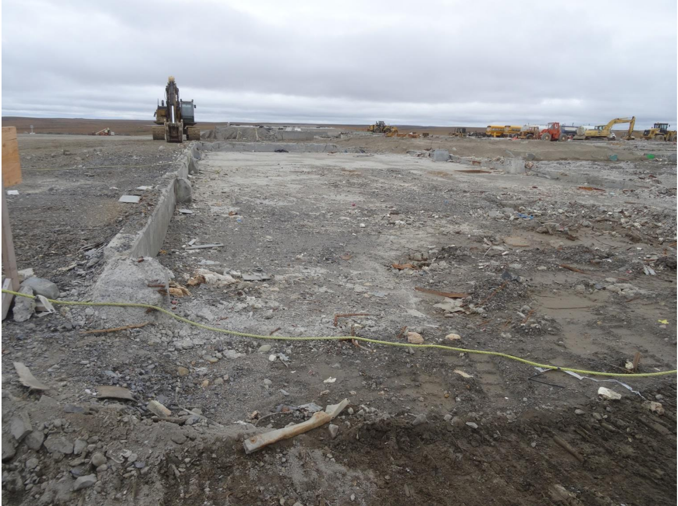
Description: #19 Batch Plant, aka Paste Plant – Concrete Foundation Remains – All Debris Removed and Placed into the Land Fill
