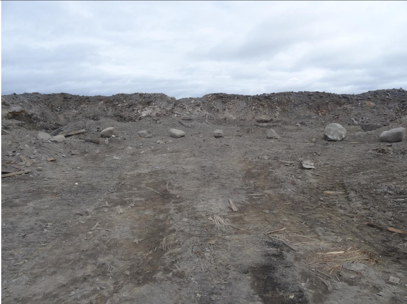
Description: Burn Pit Area – Entire Area yet to be Excavated, Capped and Covered
