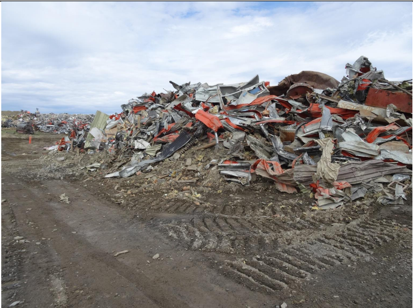
Description: Temporary Storage of Demolished Debris – View 1
