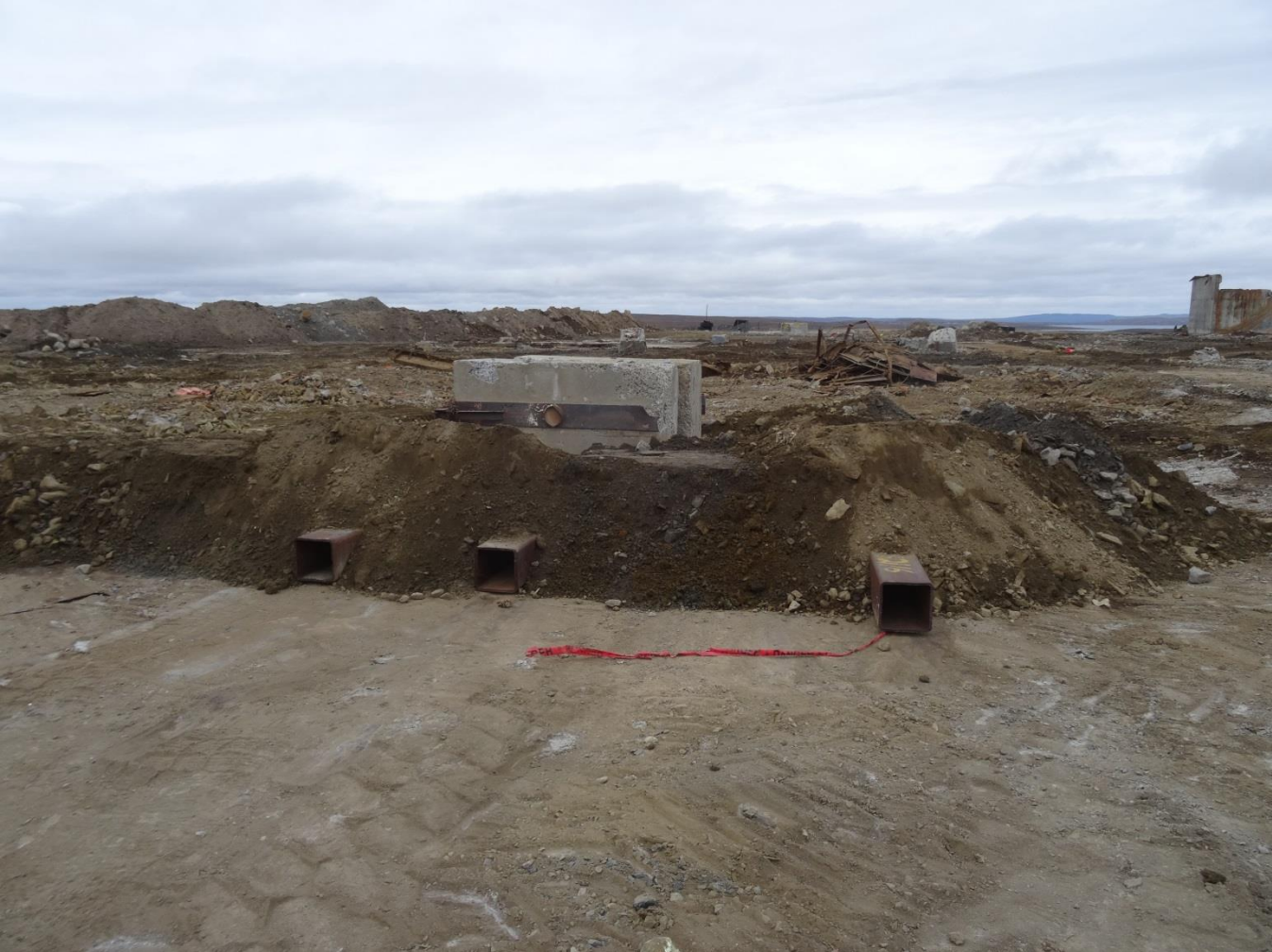
Description: Shaft Hole – All Debris Removed and Placed into the Land Fill
