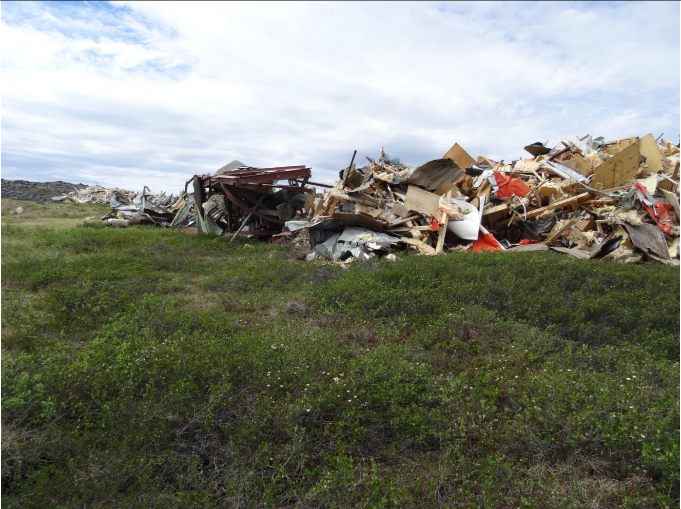
Description: Temporary Storage of Demolished Debris – View 4
