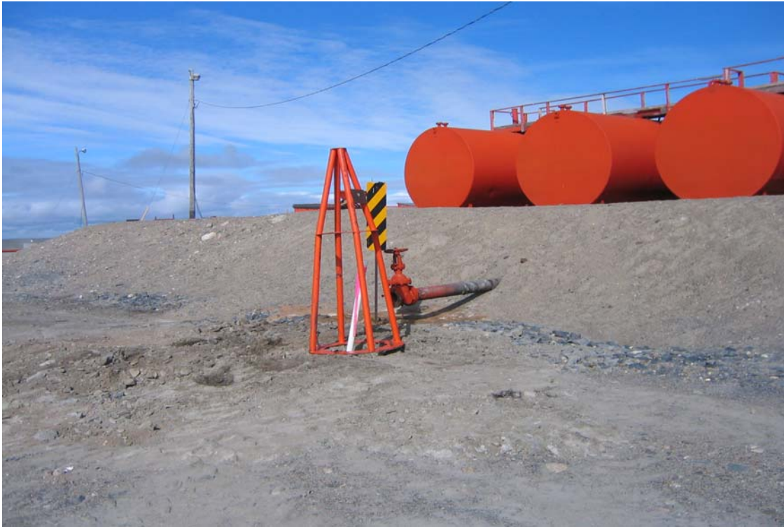
Photograph 45: Typical completed monitoring well (05-28), with "Quadra pod" placed for protection, July 2005 (APEC 3a).
