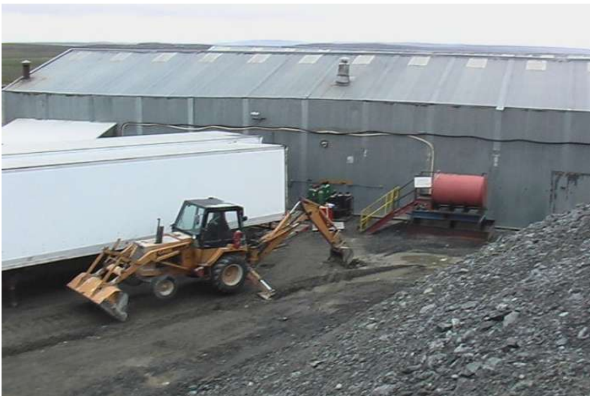
Photograph 32: Test pit 05-44 being excavated south of the RTL Shop, July 2005 (APEC 5a).
