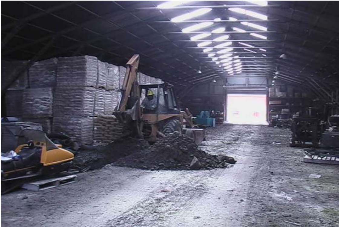
Photograph 27: Excavating test pit 05-18 inside of the Cold Storage building, July 2005 (APEC 4b).
