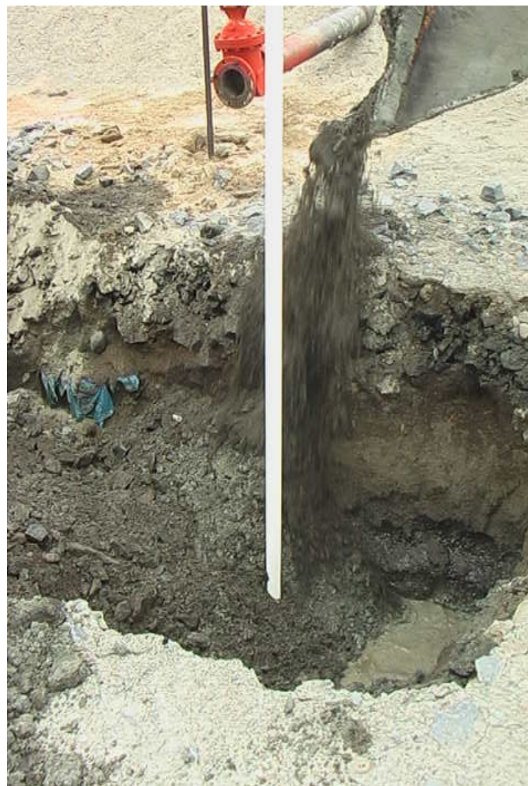
Photograph 44: Showing a typical installation of a monitoring well in a test pit, well 05-28, July 2005 (APEC 3a).
