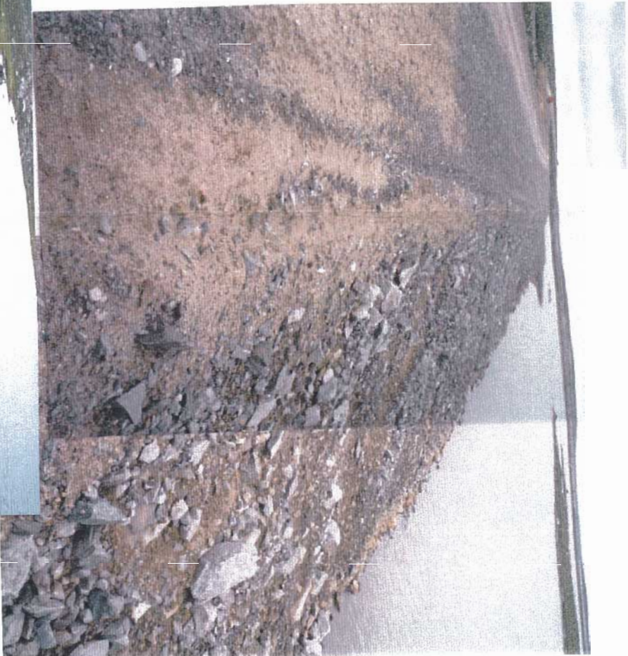
Two shot panoramic of some of the disturbances on the upstream side riprap of Dam #4. This disturbance has been noted in previous inspections.
