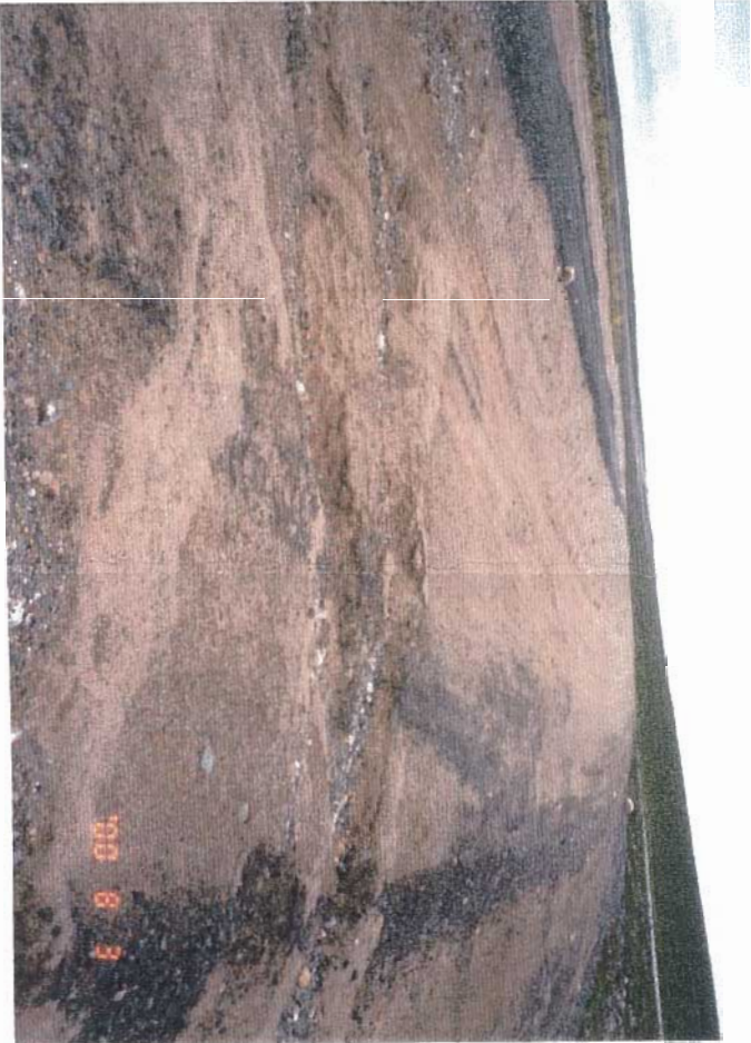
View of another erosional gully which is formed right across the crest of Dam #3. This one is located approximately 20 meters south of the bend in the dam. Again, this small erosional gully should be graded over and/or back filled to prevent any further concentration of run off water and further erosion.
