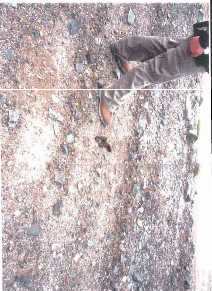
View of a small sink hole located in the downstream third of the crest of the dam. This small sink hole is approximately 8 to 10 inches long.
