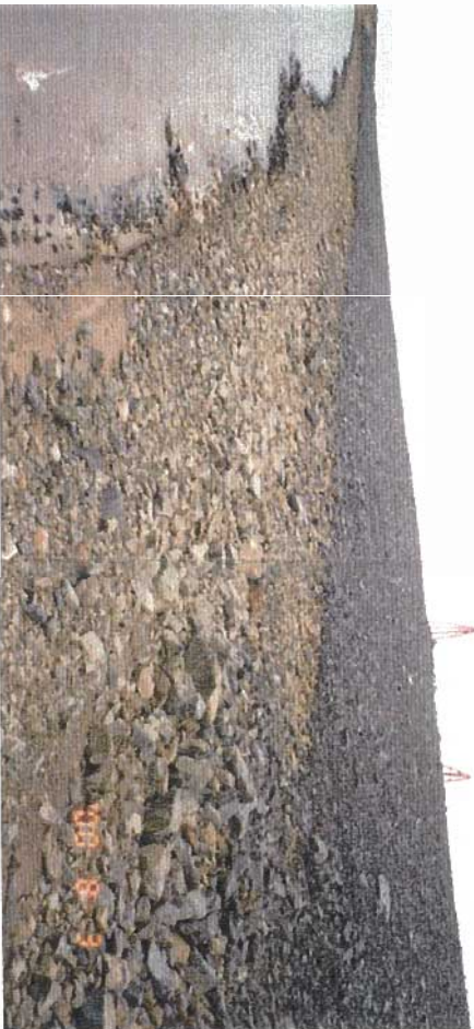
View of the riprap on the upstream side. There is a marked change in colour in the riprap from the dark grey material on the upper portion to the light tan colour on the lower third of the slope. There is a slight scarp formed where the water has been lapping, approximately at the contact of the dark grey to the light tan riprap.
