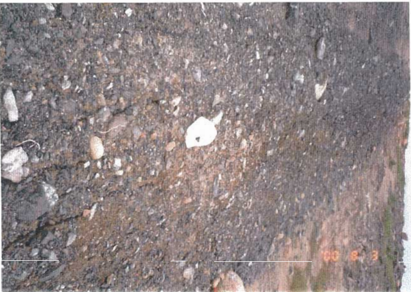
View of 2 to 3 parallel tension cracks found at the toe of Dam #3. This is on the steep northwest portion of the dam. Cracks at this location had been noted in previous inspections.
