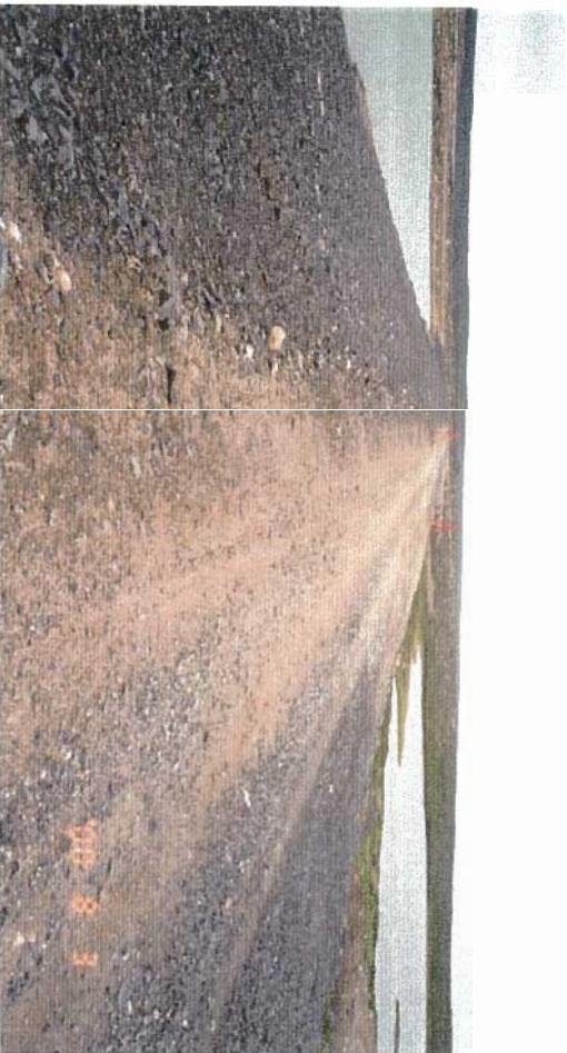
View of the crest of Dam #2, which appears to be in generally good condition and is graded smooth.
