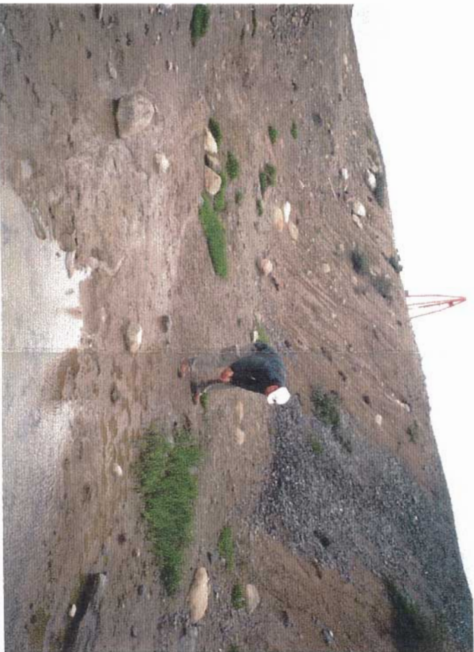
View of the riprap on the upstream side. There is a marked change in colour in the riprap from the dark grey material on the upper portion to the light tan colour on the lower third of the slope. There is a slight scarp formed where the water has been lapping, approximately at the contact of the dark grey to the light tan riprap.
