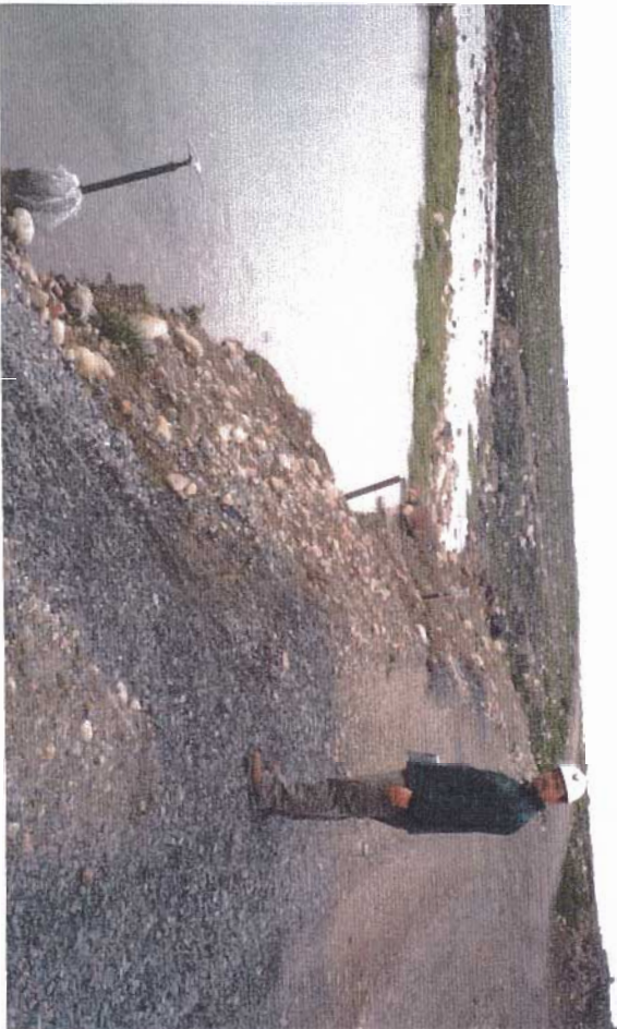
View of the downstream side of the access road berm at the toe of the dam. Dark grey angular blast material has been previously placed in a number of the small erosional scarps. A number of these scarps are continuing to erode back into the access road, probably because the blast material was installed too steep.
