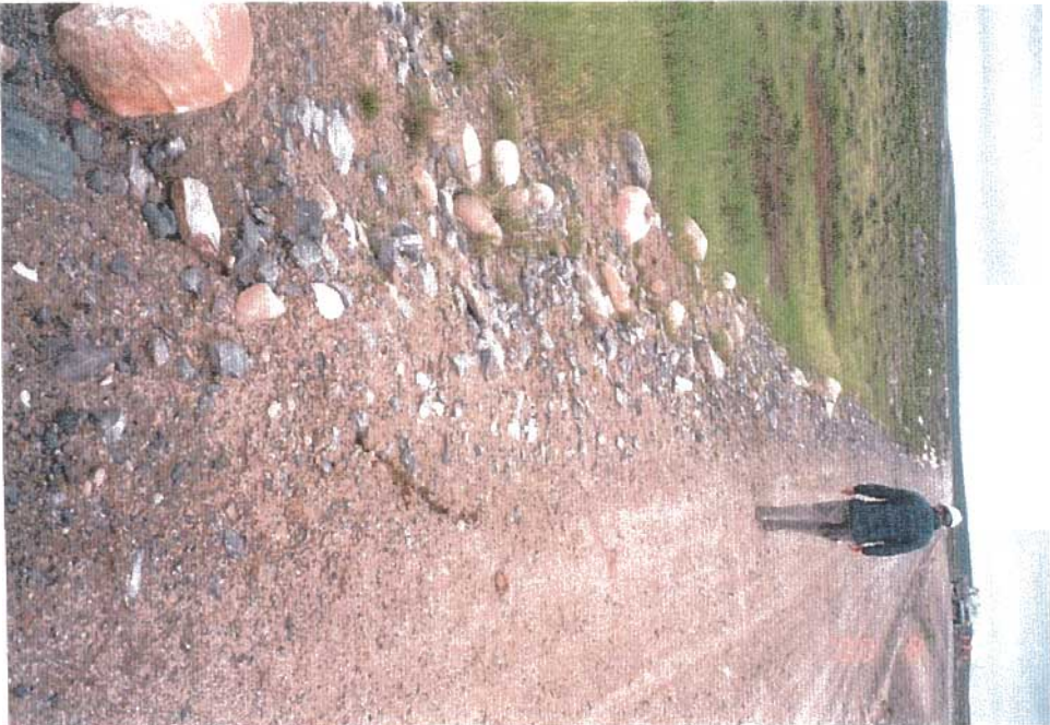
View of a minor settlement trough and cracking at the downstream side of the access road toe berm.
