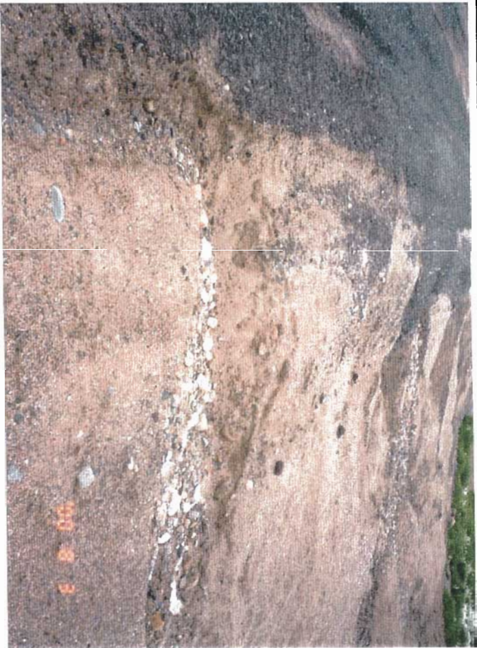
View of one small erosional gully located at the toe of Dam #3. This erosional gully is approximately 3 meters long by 1 meter wide and is armoured with some cobbles and boulders. In the background, the remnants of two previous erosional gullies can be seen.
