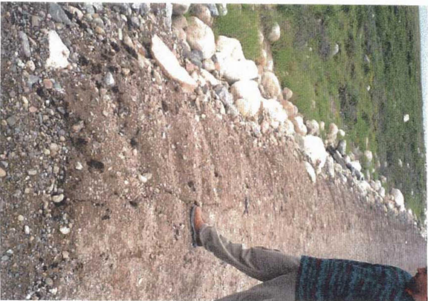
View of a thin longitudinal crack located right at the downstream edge of the berm on the downstream toe of Dam #2. This crack has a trace distance of approximately 15 to 18 meters along the toe. Some small associated settlement troughs are located adjacent to this crack.
