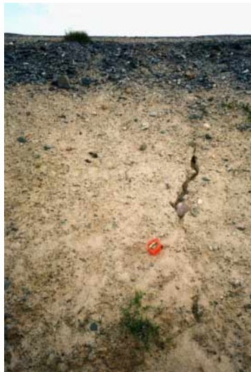
View of a thin erosional gully located on the downstream side of Dam 1B. This erosional gully is located about 30 meters south of the north abutment of this dam. The erosional gully is some 3 centimetres wide.
