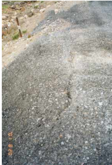
View of some cracking near the toe..
