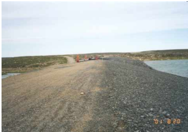
View of the crest on the upstream of Dam #1A looking north. There are no signs of cracking, deformation, or erosion except for one minor sinkhole.
