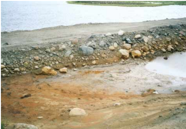
Shows a close up of the area where the seepage discharge is incoming from the downstream side.
