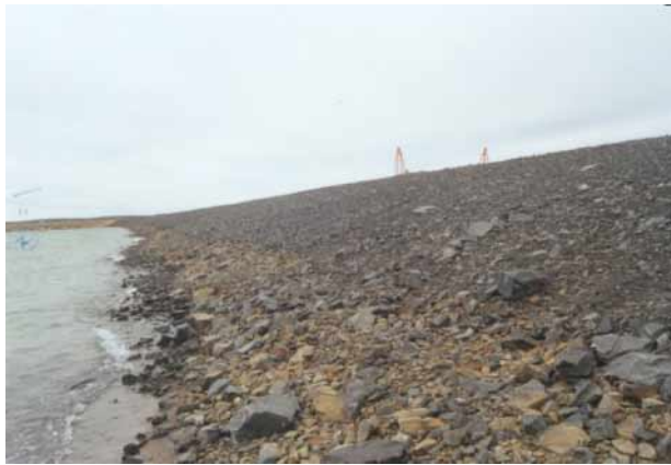
View of the upstream side of this dam. As previously noted, there is a small scarp formed at the contact of the light brown to the grey material.
