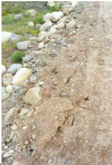
View of some minor crest edge cracking located along the downstream edge of the access berm.
