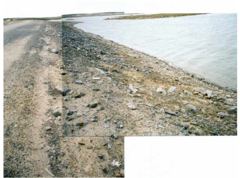
View of the disturbed area on the upstream side of the Dam 4. As can be seen, some of the light brown sandy material is sticking through where the dark grey riprap has been disturbed.
