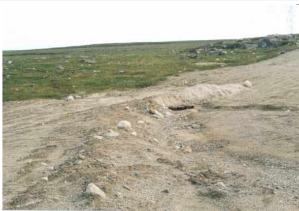
Shows four small diameter pipes that have been placed in a previously noted erosional gully. A properly constructed swale should be located here instead.
