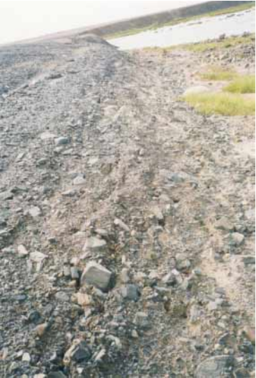
Shows some cracking located at the toe which runs in a discontinuous manner for perhaps 20 to 30 metres.
