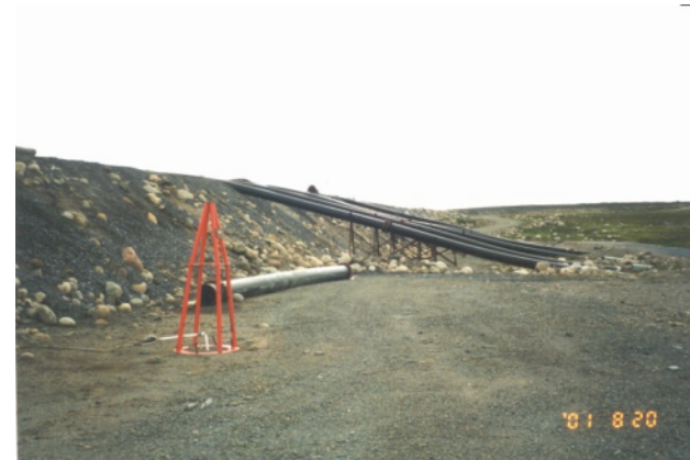
View looking back along the toe and the backslope of Dam 1A. No signs of seepage, settlement or erosional concerns other the minor cracking were noted.
