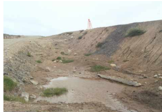
Shows the small pond and seepage discharge which is occurring over towards the north abutment of Dam #2. There has been a seep going on here for the last few years.
