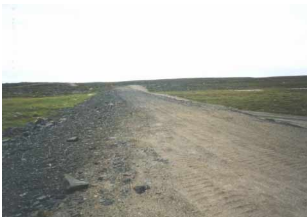
View of the crest on the upstream side of this dam. The crest is somewhat well travelled with the tire marks still visible. As previously noted, the upstream side is somewhat undulating.
