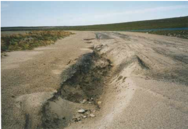
Shows a depression formed approximately 8 metres back from the crest edge for Dam 3. This depression is approximately 1 to 1.2 metres wide and extends over a distance of some probably 20 metres. This erosional gully should be back filled.
