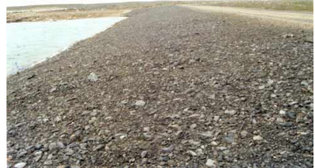
Another view of the riprap on the upstream side of the dam.
