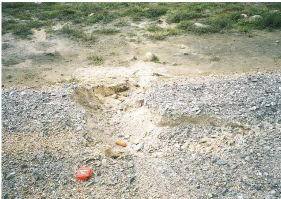
Shows an erosional gully situated at the toe of Dam 6. This gully is located approximately some 20 metres south of the north abutment. This gully is approximately 1 metre wide by approximately 0.5 metres deep.
