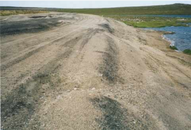
Shows an erosional gully approximately 1 metre wide by perhaps 0.4 metres deep in the foreground of this photo.
