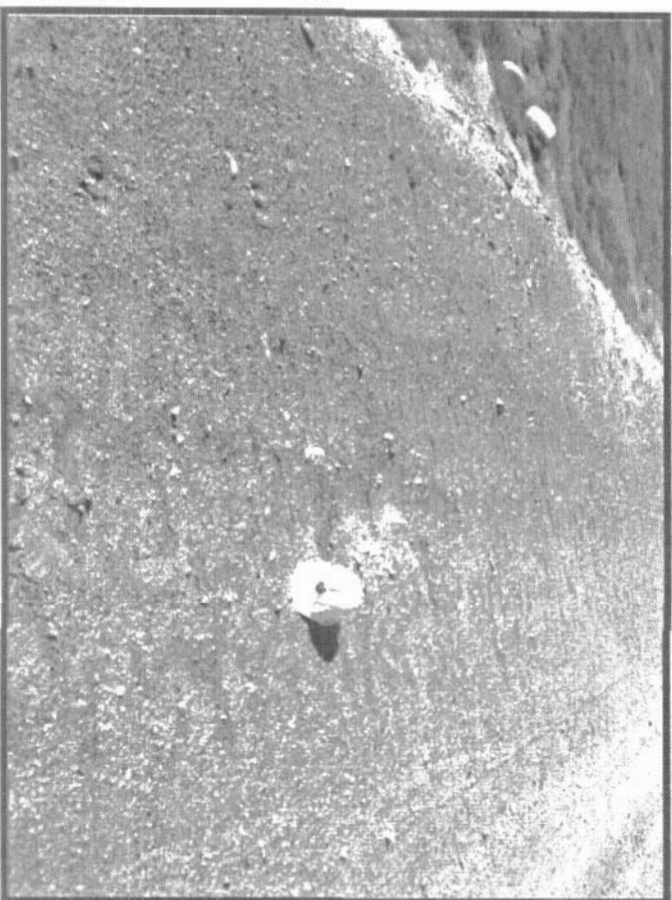
Photo 99 shows one minor sinkhole located near the downstream side of the crest. This sinkhole is located some 50 m north of the south abutment.
