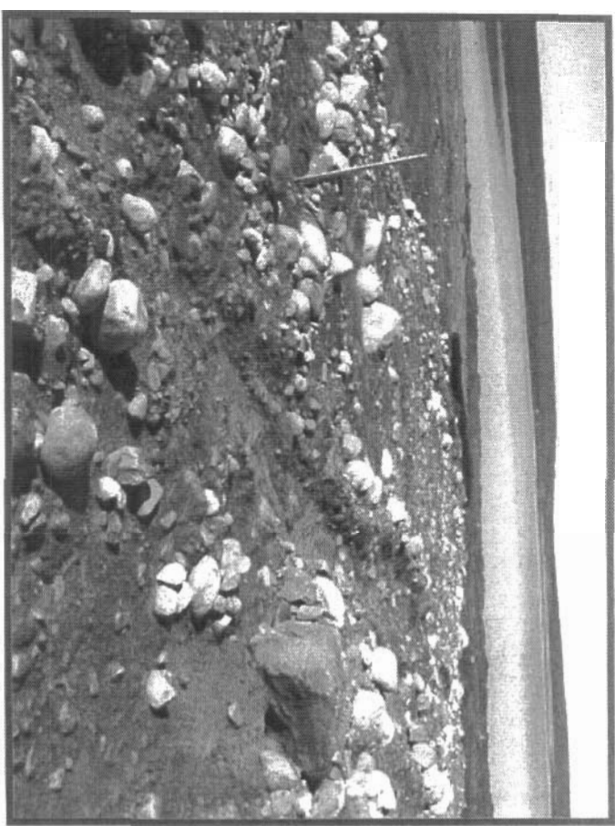
Photo 137 Shows some boulders and cobbles that appear to have been placed in a low swale area. At the current time, the swale work is very disturbed and would likely be ineffective in transmitting any water. The material should be excavated and a proper swale should be laid out.
