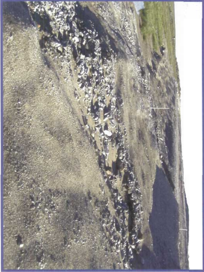
Photo 141 Shows a remnant erosional gully located at the toe.
