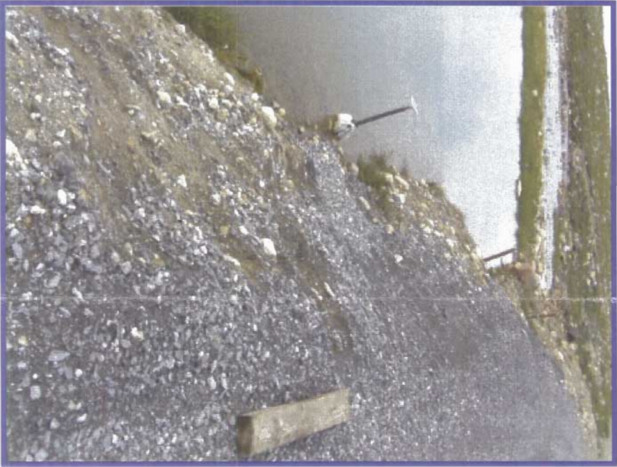
Photo 70 shows the little scarps formed by the retrogression of the material right at the toe of the access road berm.
