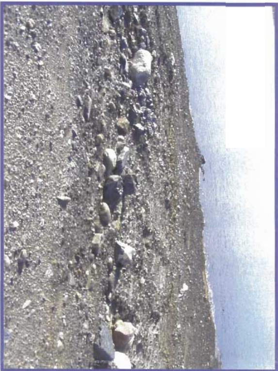
Photo 115 shows some of the disturbed area on the upstream side riprap. It appears that additional material has been placed on the crest and was graded over, perhaps to correct some of the earlier rutting caused by construction activity. The large number of boulders that have segregated out on the side of the fill to confirm appears that assumption.
