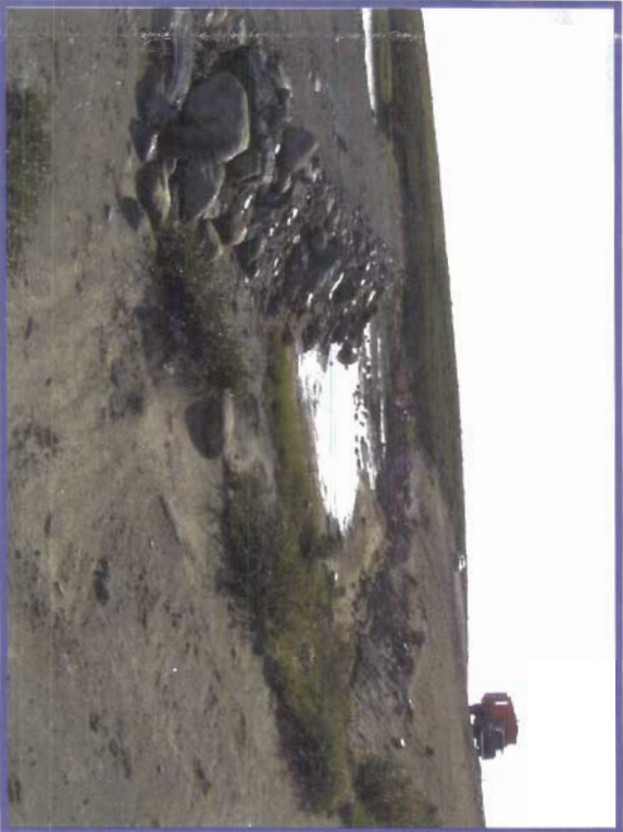
Photo 130 Shows the small pond which is located between the toe of Dam 4 and the small berm on the left of the photo. This area is pumped dry for the following two reasons; 1.) allow inspection of the downstream toe and 2.) to confirm the origin of the water in the pond.
