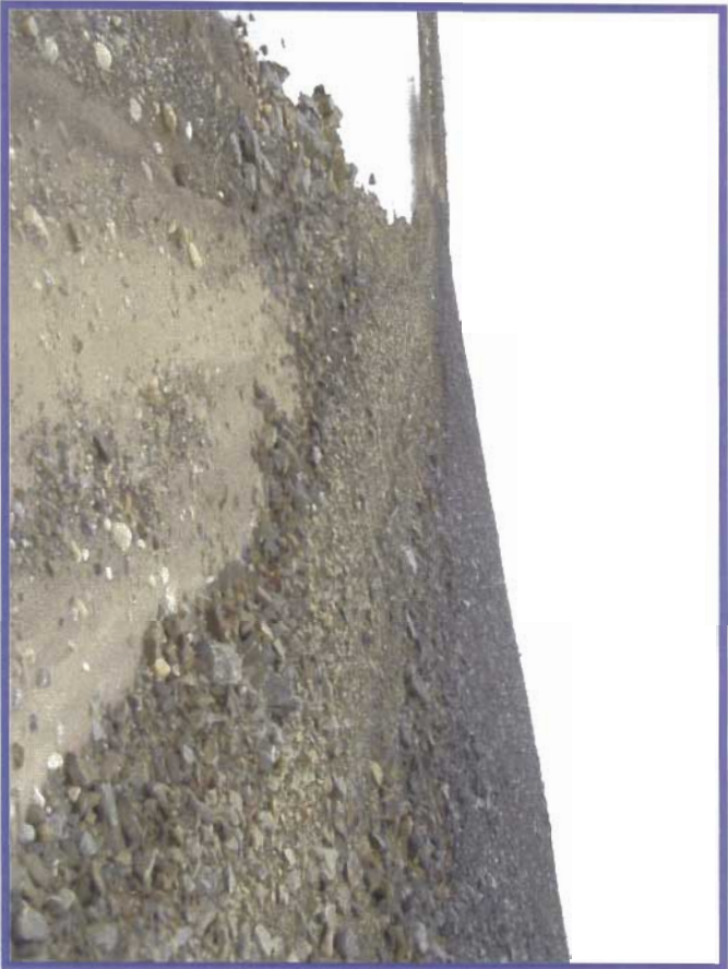
Photo 44 shows a view of the upstream side, taken from waterline perspective. As can be seen and has previously been noted, there are some small scarps at the transition from the light brown to the gray material.
