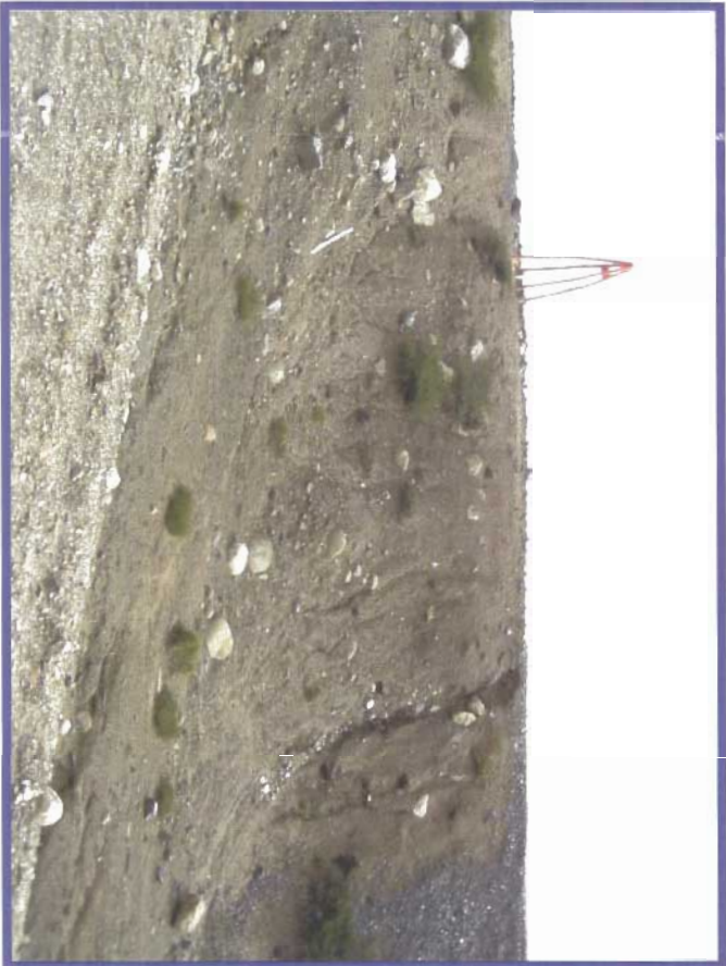
Photo 59 shows one significant erosional gully located on the downstream face at the north abutment.
