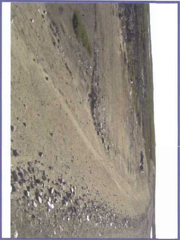
Photo 121 shows a view of the relatively steep toe of this dam, followed by the flat graded area below the toe. No signs of sloughing or significant erosion are noted from this vantage point.
