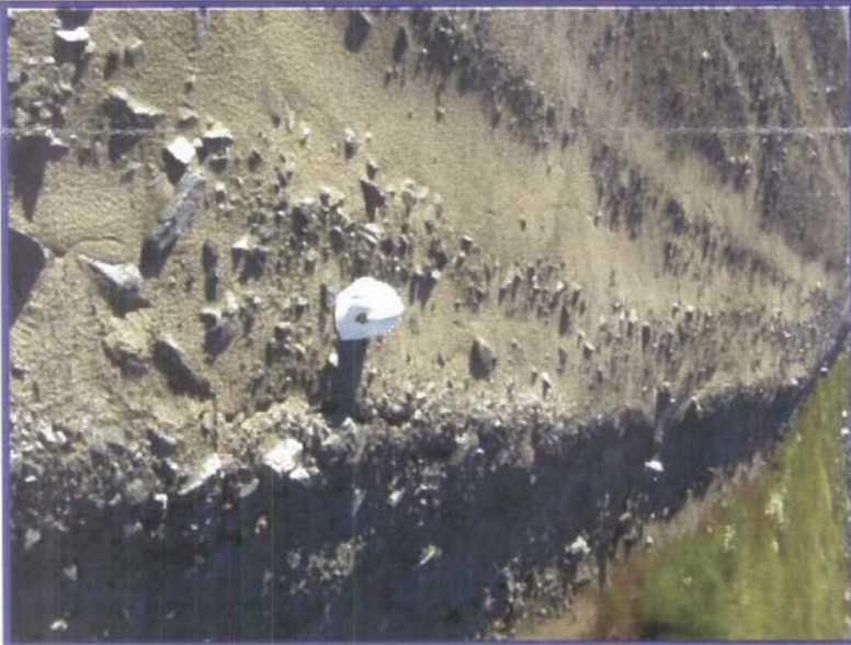
Photo 142 Shows a number of tension cracks within this toe area. The cracks are discontinuous but can generally be observed over a distance of some 10 to 15 m.
