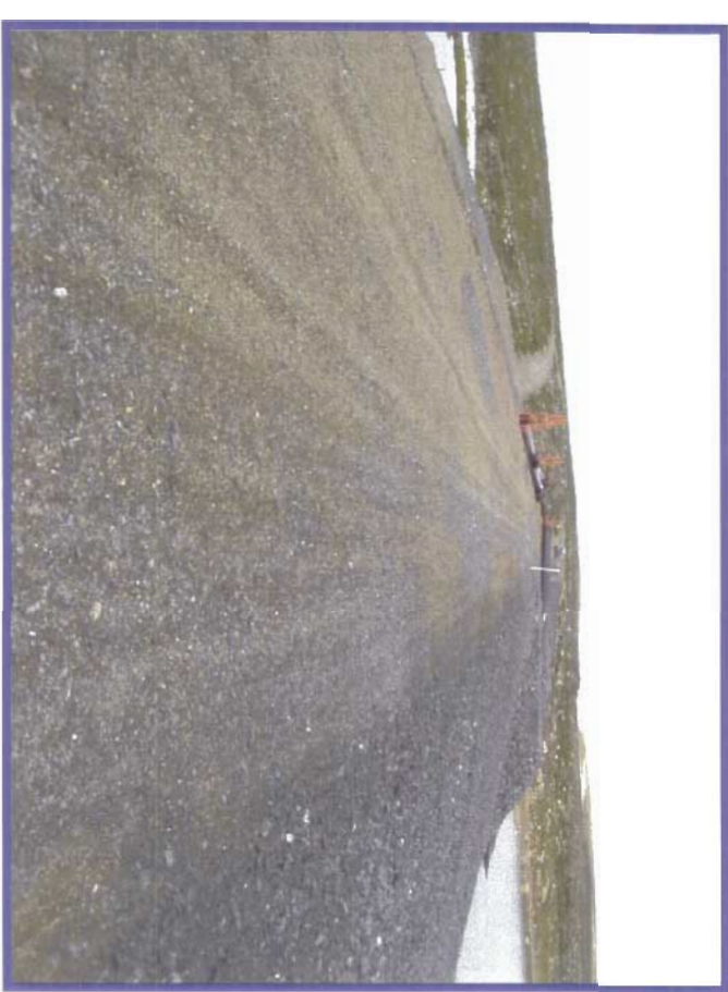
Photo 67 shows a view of the crest looking towards the north abutment. No signs of settlement, deformation or cracking noted on the crest.
