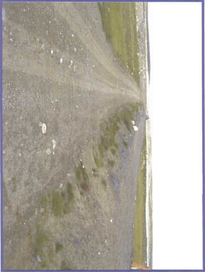
Photo 79 shows the downstream side and the crest of the dam looking towards north. Some minor vegetation is catching onto the slope.
