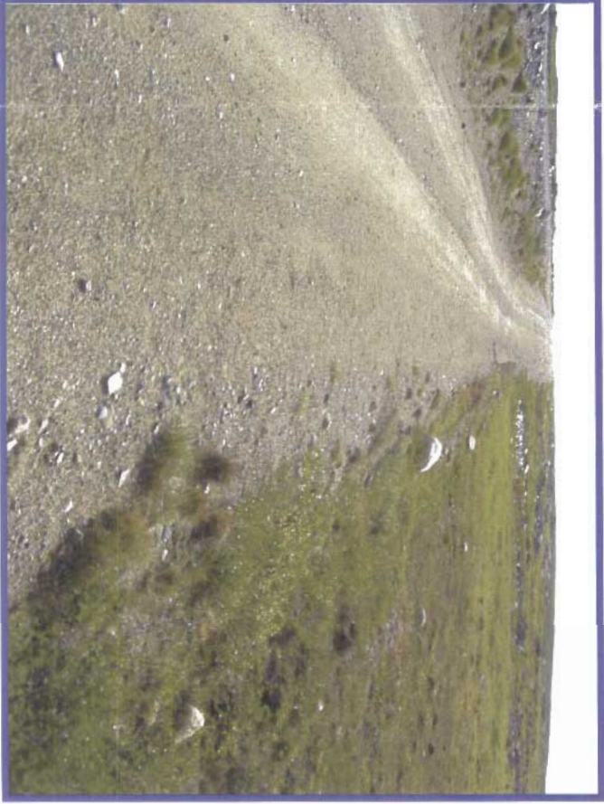
Photo 80 is a view along the downstream toe. No signs of seeping water were noted.
