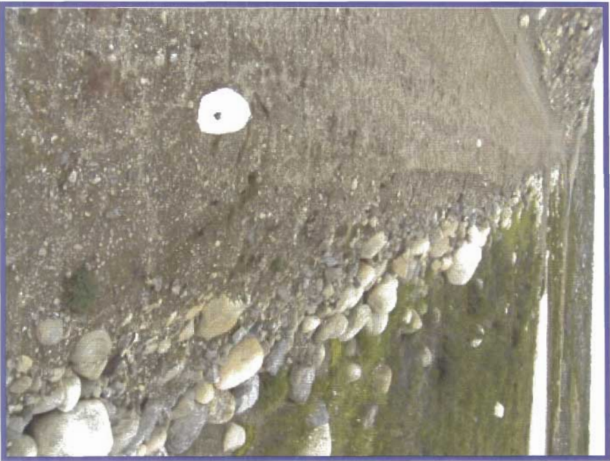
Photo 51 shows some minor cracking along the downstream toe. This cracking has been previously noted.
