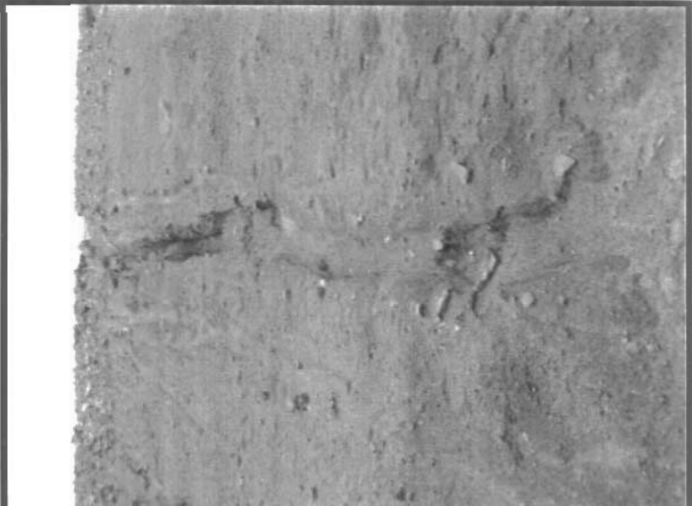
Photo 67 shows a narrow erosional gully which should be backfilled.
