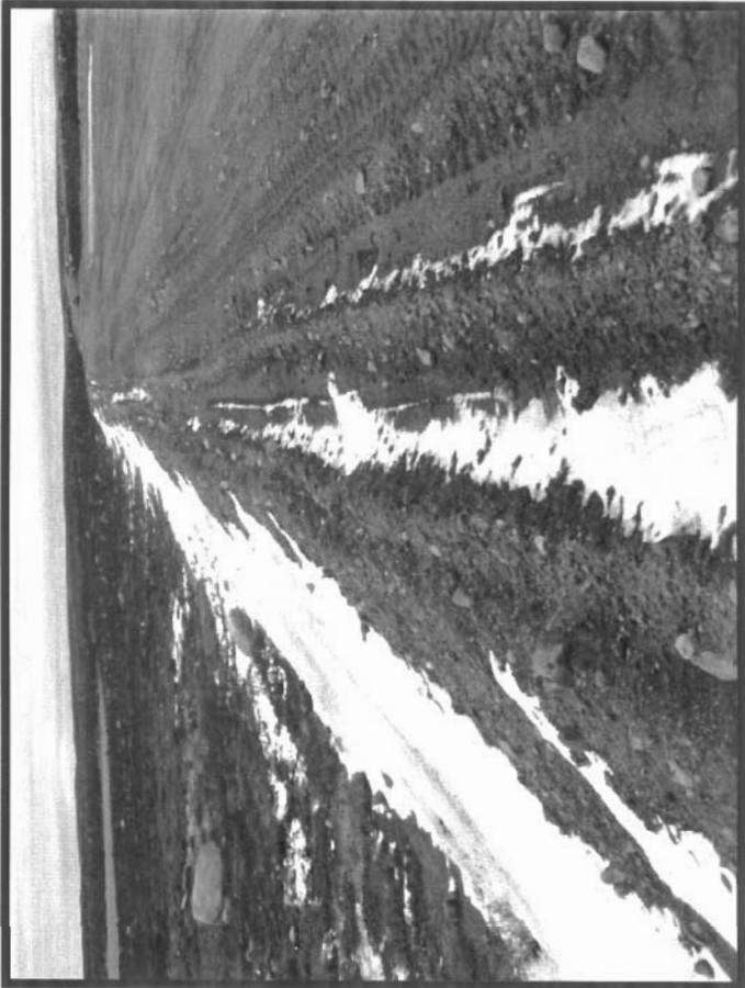
Photo 47 shows a view of the downstream toe looking towards the north. Construction traffic has caused a number of ruts and pushed up some windrows on the toe crest.
