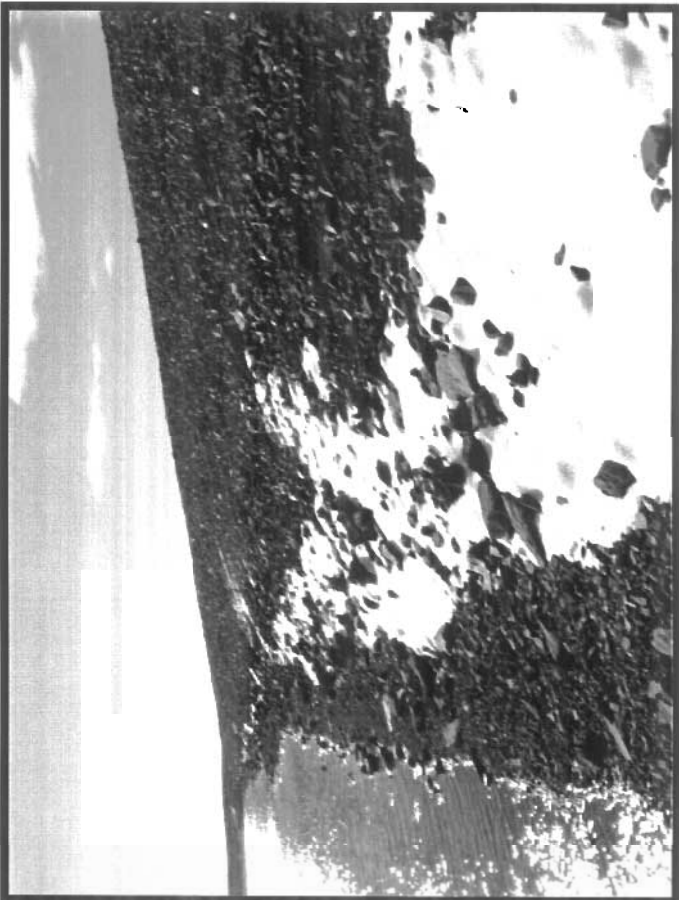
Photo 4 is a view of the upstream side. The distance from the current pond level to the crest is approximately 3.5 metres. Occasional small scarp form at the water level.
