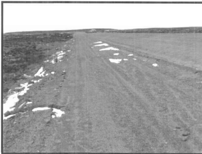
Photo 38 is a view along the access road toe berm. The downstream side has no signs of deformation or cracking from this perspective.
