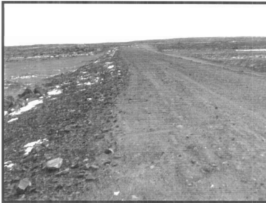
Photo 29 is a view of the crest on the upstream side. As previously noted, the riprap on the upstream side is relatively undulating. This dam does not currently retain any water.
