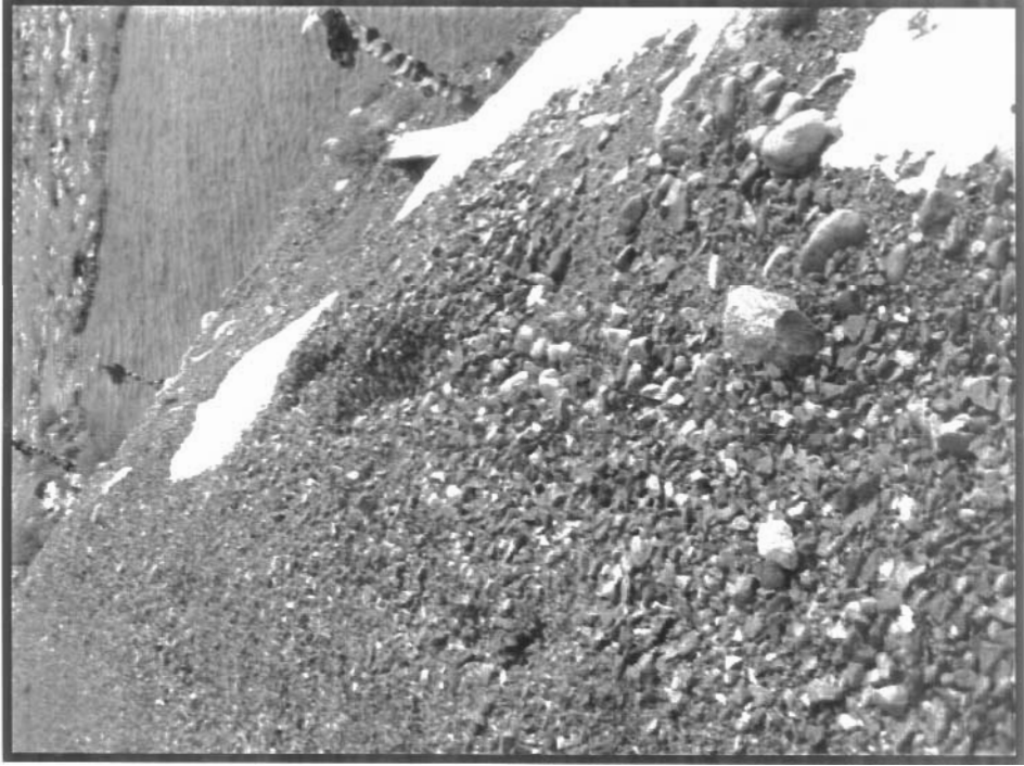
Photo 27 shows some longitudinal cracks formed in the angular rock fill. These cracks were previously noted proximal to the valve locations.
