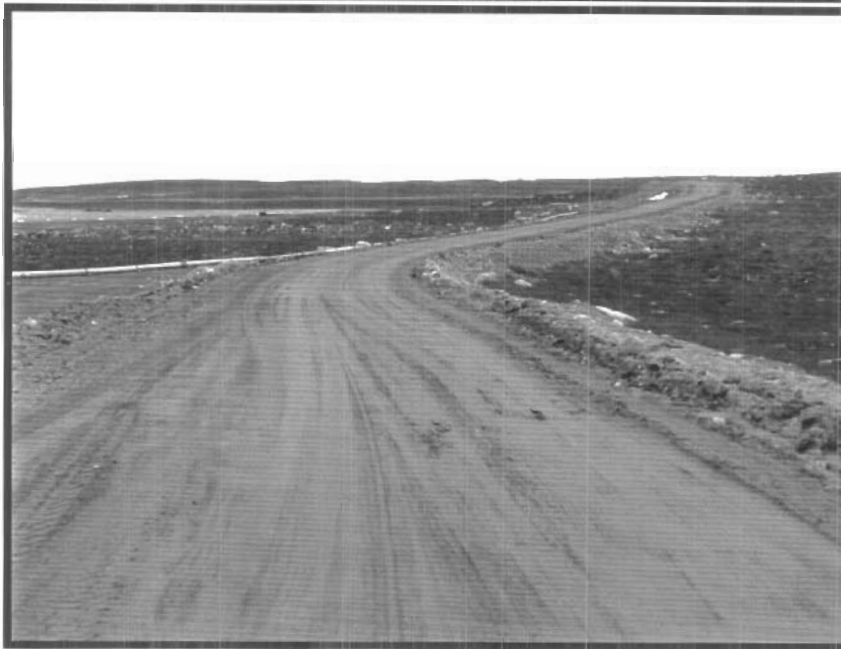
Photo 54 shows the crest of this dam and the downstream side. Windrows have been formed by recent grading activity for vehicle access.
