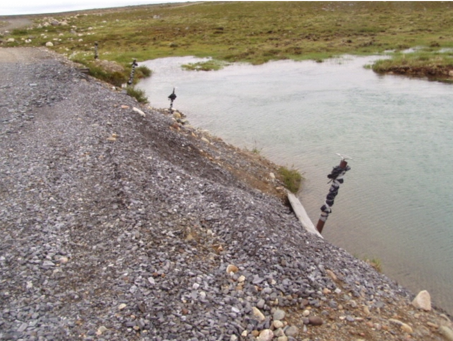
Photo shows the steep face overlooking the valves which come from the discharge pipes. The rockfill slope is oversteepened and there are some longitudinal cracks.
