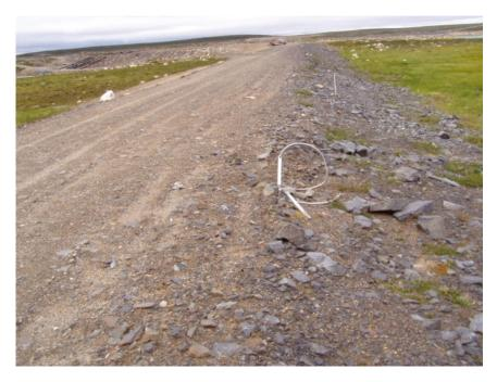
Photo shows the upstream side. No observations of settlement or cracking were noted.
