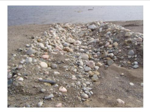
Photo shows the armouring in the swale which then runs down towards Boomerang Lake. Portions of the armouring are somewhat disturbed due to settlement, but overall, it performs its function.
