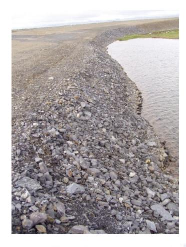
Photo shows the armouring where the end of Dam 3 comes in contact with Boomerang Lake. This riprap and armouring all appear in good condition.
