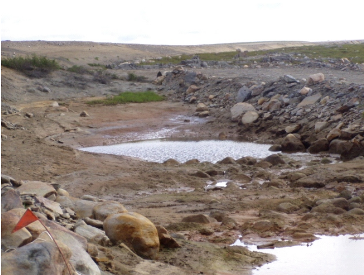
Photo shows the small remnant pond near the east end of the dewatered area. Seepage is coming in from the lake side located on the downstream side of the pond.
