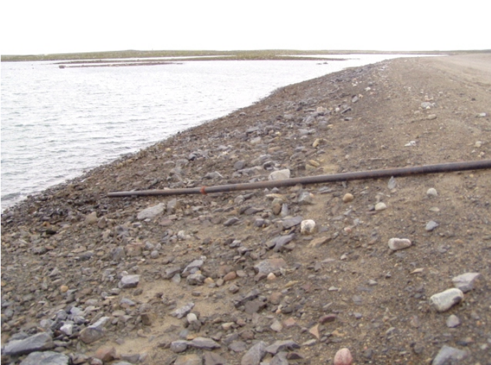
Photo shows the position of the riprap on the upstream side. It is rather undulating as previously noted.
