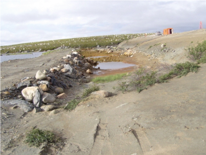
Photo shows the cofferdam area at the toe and the small remnant ponds which remain after pumping.
