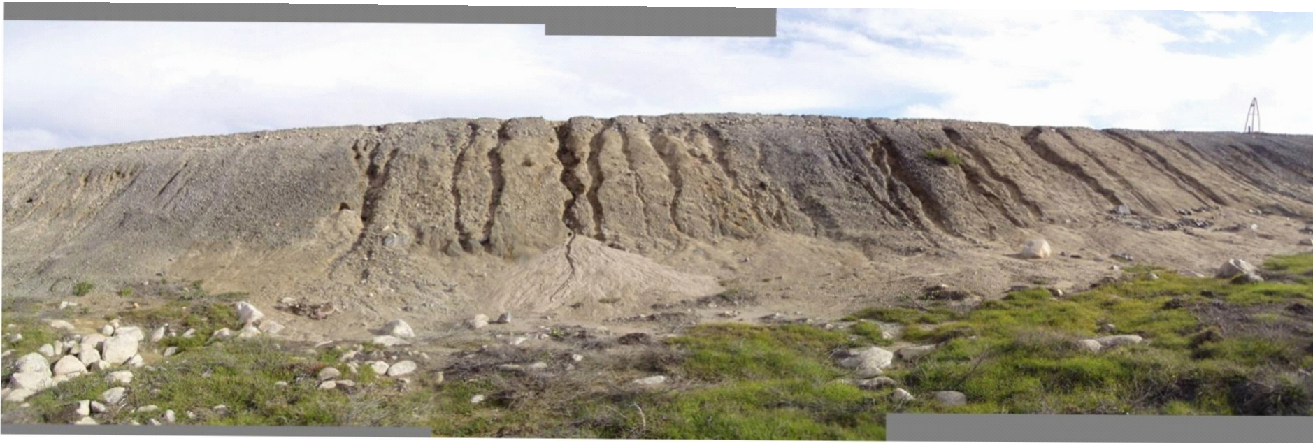
Photo shows a number of erosional gullies located on the downstream face over towards the east abutment. These gullies should all be properly backfilled to prevent further erosion.
