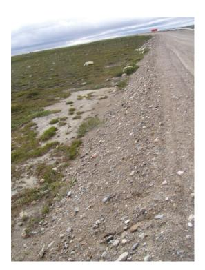
Photo shows the downstream slope of this dam. No signs of erosion or seepage noted from this perspective.
