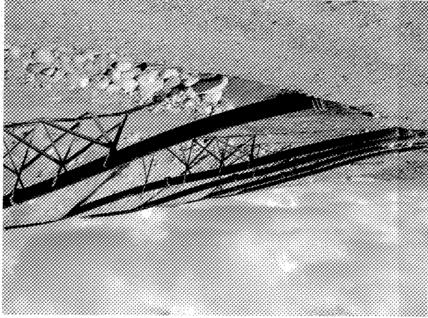
View of the five decant siphons on the downstream side some which have been partially dismantled.
