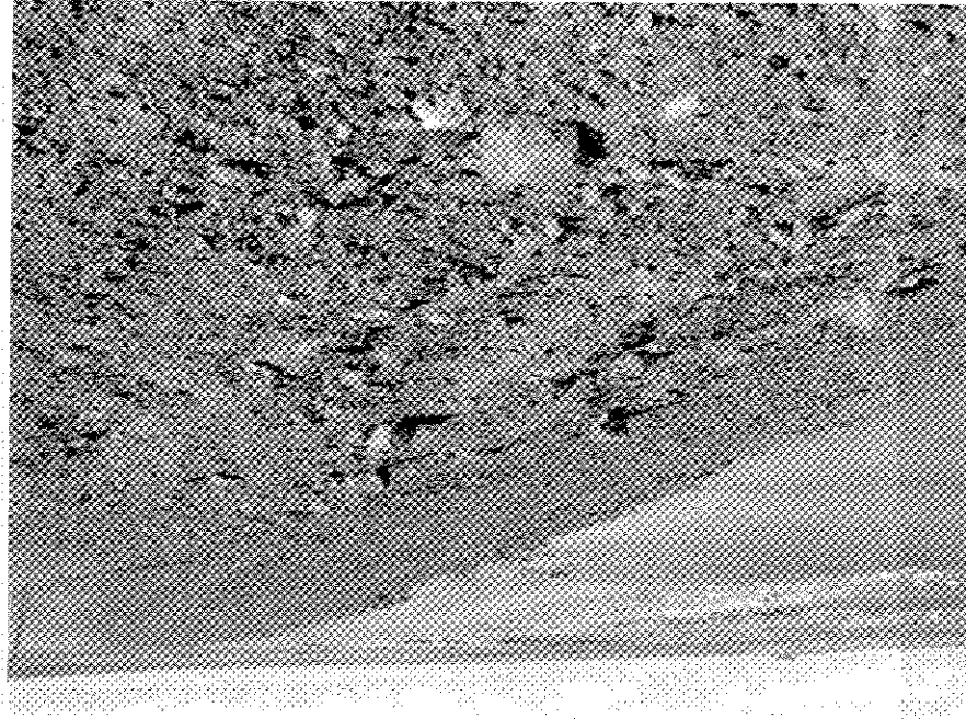
Shows the previously noted disturbed area on the upstream side. There doesn't appear to be any new cracking or deformation associated with this area.
