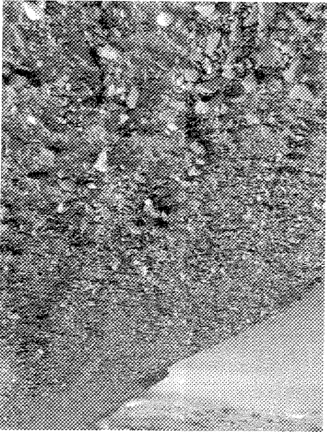
Shows some longitudinal cracks in the riprap on the upstream side.
