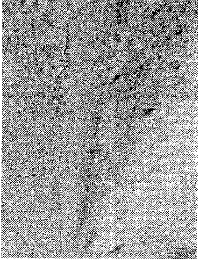
Shows longitudinal cracks located at the downstream toe of the fill.
