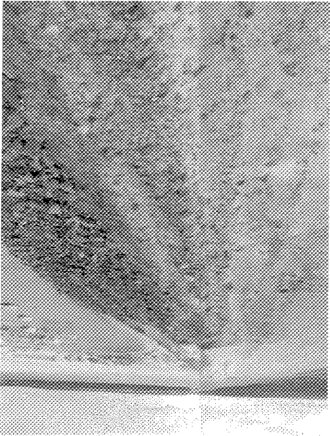
Shows some longitudinal cracks within the fill material located in the berm.
