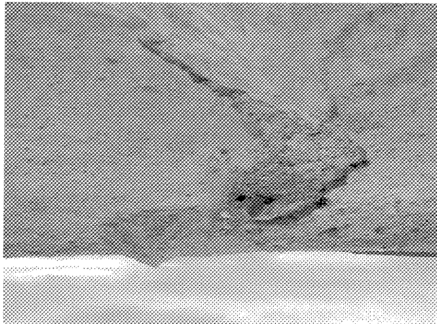
Shows an erosional gully right at the west abutment of this dam. This gully tends to stem from an uphill ditch which focuses the erosional forces of water from the slope above.
