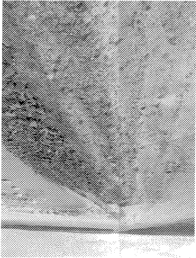
Shows some longitudinal cracks within the fill material located in the berm.
