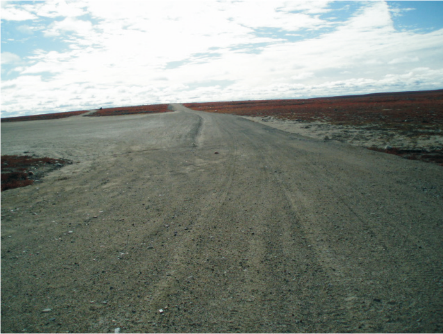
Shows a view of Dam 6 looking towards its south abutment. This area is completely reclaimed and there is no pond retained.
