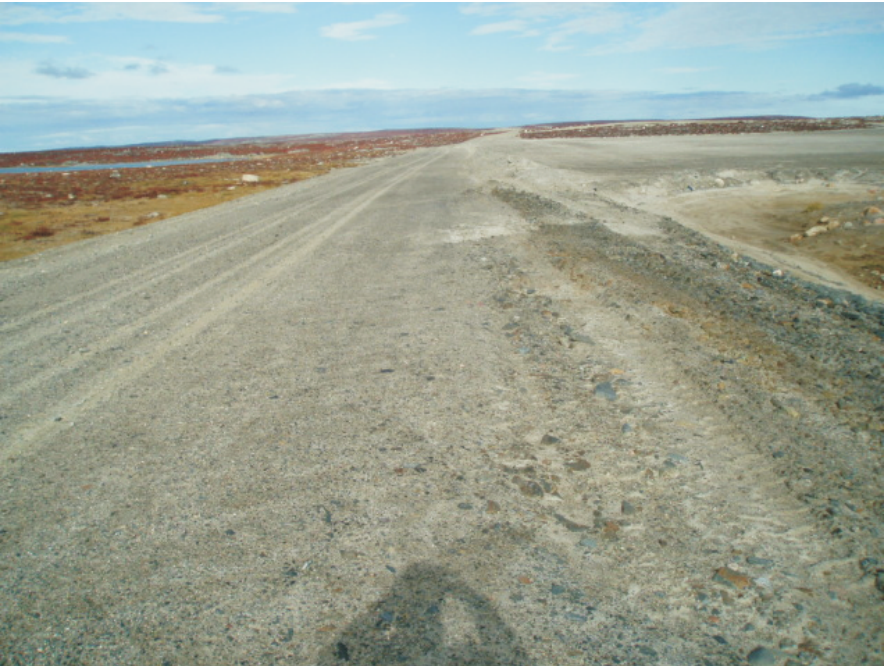
View of the crest looking towards the north abutment. We can see the reclaimed cover sand on the upstream side being .75 m higher than the dam crest.
