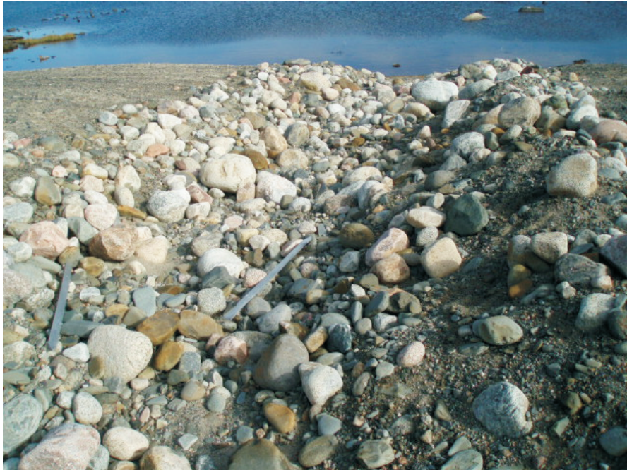
Shows the armoured channel which conveys ditch water across the crest, which appears in satisfactory condition
