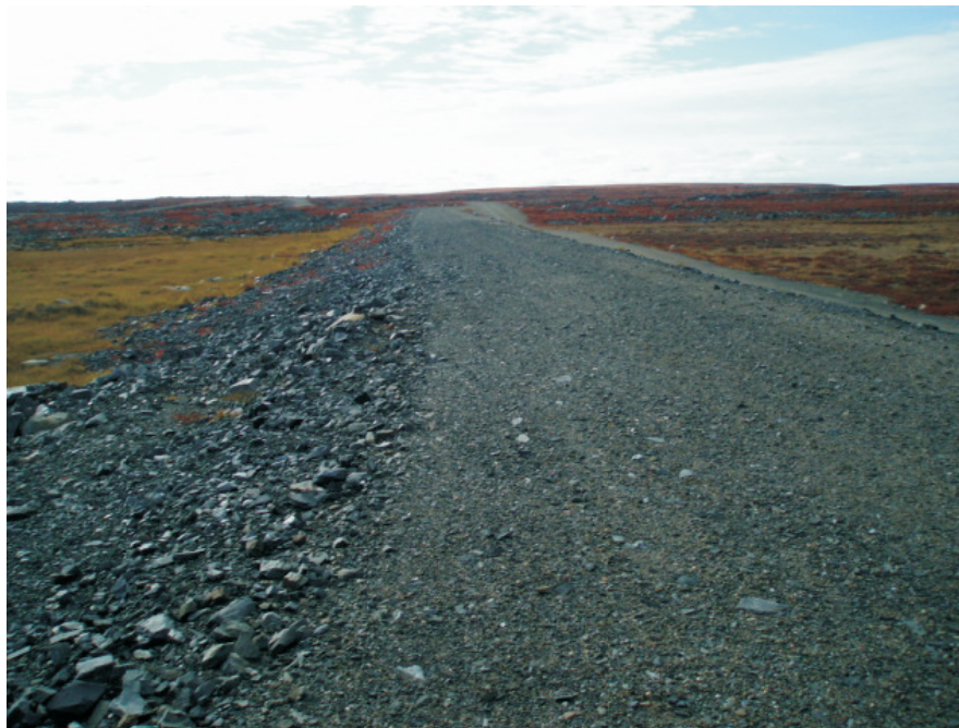
Shows the crest and upstream side of Dam 1B with no signs of deformation or settlement.
