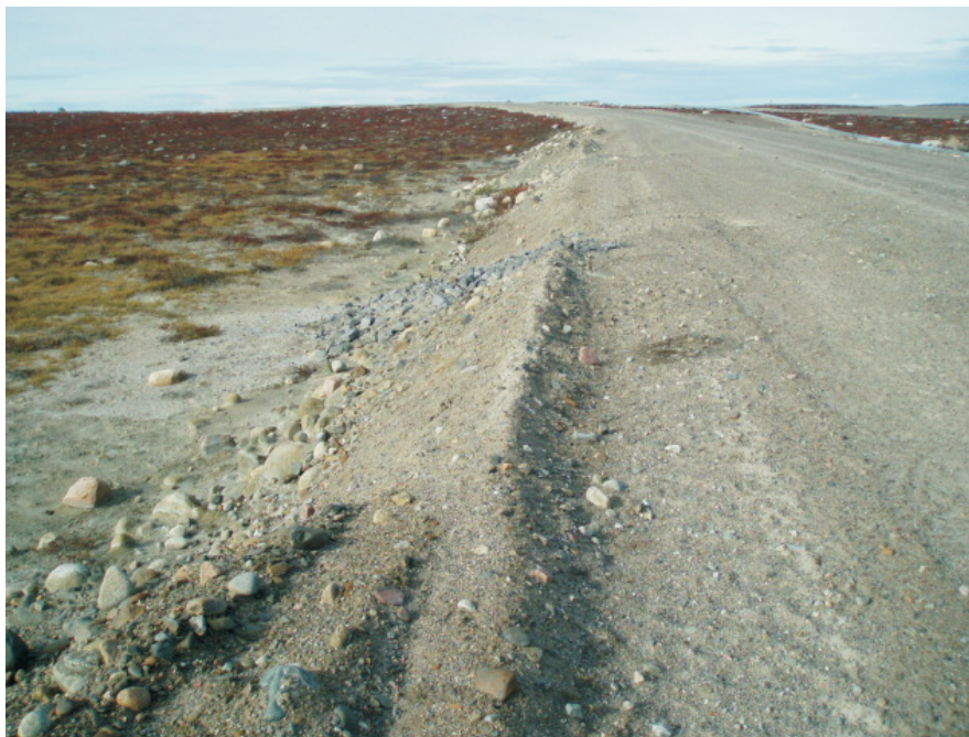
Shows some angular riprap that was previously placed in erosional gullies located at the toe.
