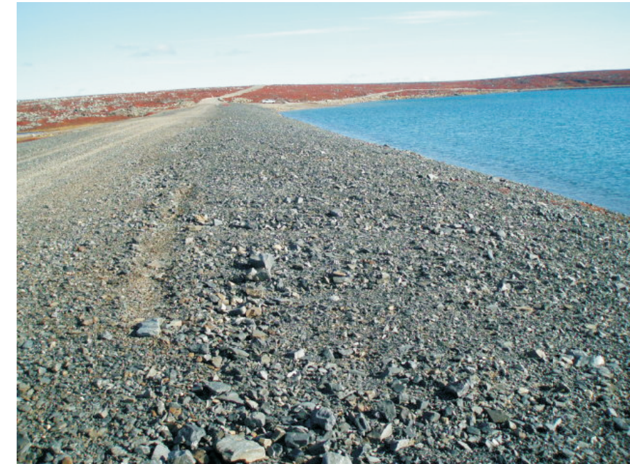
View of the crest and upstream slope looking towards the north abutment. There are no signs of deformation or erosion.
