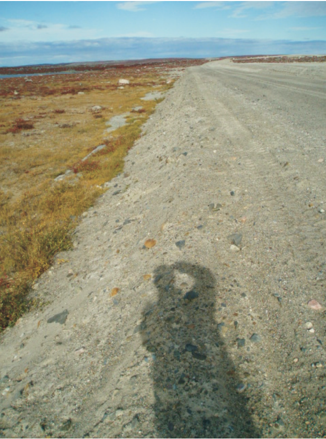
View of the downstream toe where we see some accumulation of wind blown sand in the grasses beyond the toe. No signs of seepage or significant erosion are noted at the toe.
