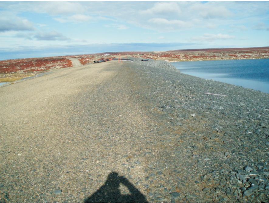
View of the crest and upstream side looking towards the north abutment. No real signs of deformation or settlement noted.
