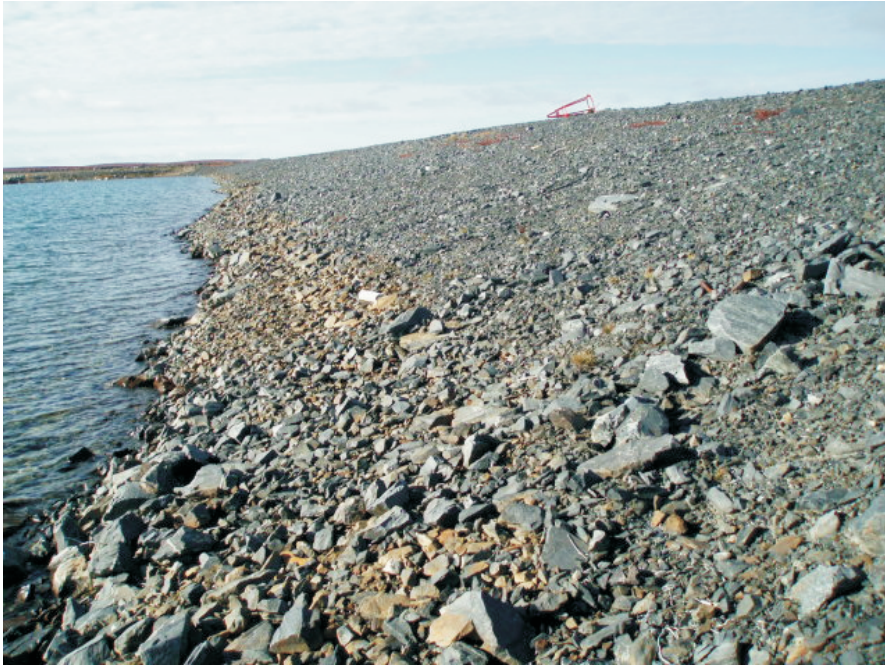
Shows the two colours that appear on the riprap on the upstream side and the small scarp which has formed at the water line.
