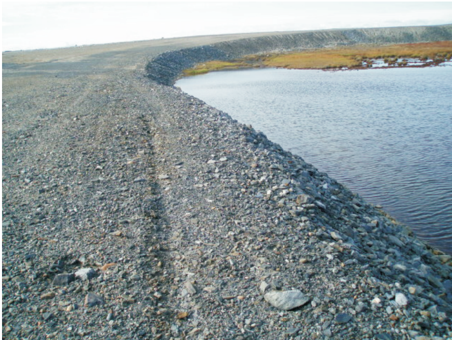
Shows the section of the toe of Dam 3 looking at its confluence with the main haul road. No signs of seepage, significant deformation or erosion were noted.
