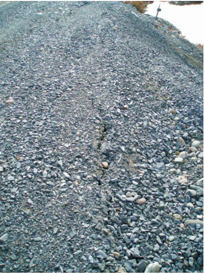
Shows some longitudinal cracking and a small scarp located along this berm edge along the toe.
