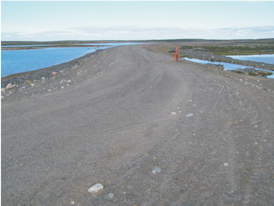
The crest of Dam 4 as seen from the right abutment. The crest is in good condition.
