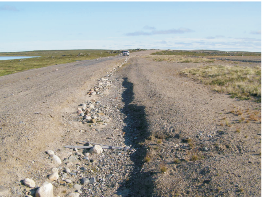
An armoured ditch which collects the run-off coming off the covered tailings area. This ditch is eroding in some sections and needs maintenance.
