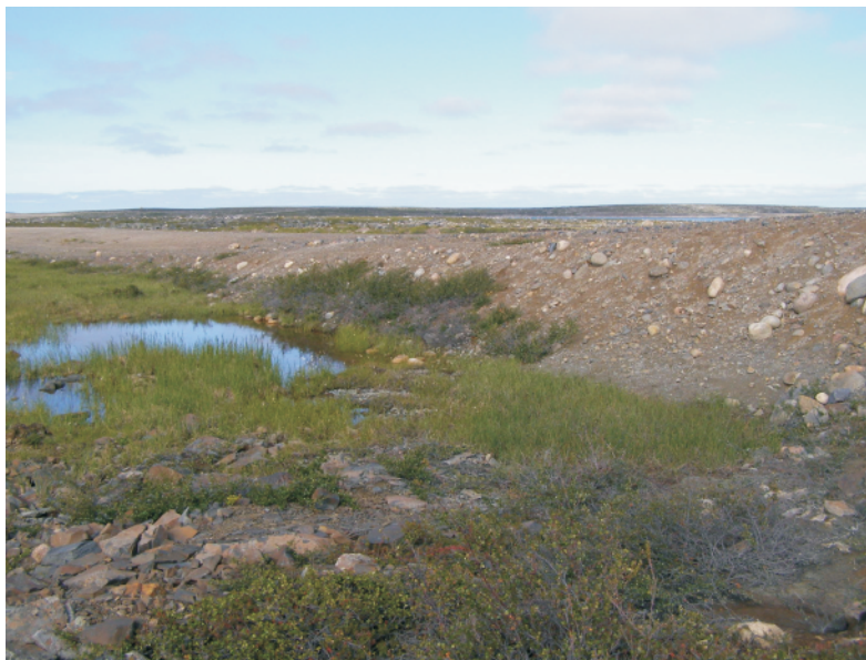
A view of the downstream face of the Dam 1C with a small pond of water adjacent to it, near the left abutment.
