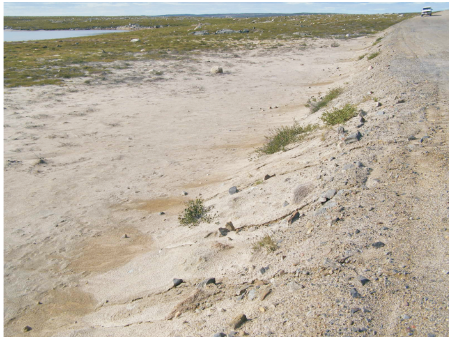
The downstream edge of Dam 6 with some minor erosion gullys Note the sand deposited along the face of the dam after being blown over the crest from the tailings cover.
