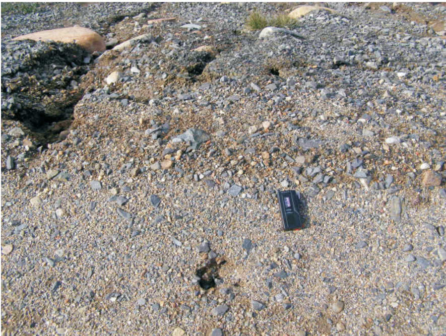
The crest of Dam 2 where a small sinkhole was noted directly above an erosion zone.
