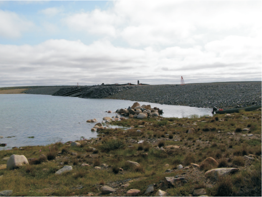
An overview of the upstream face of Dam 1A. There is currently about 3 m of freeboard and the upstream face shows no signs of distress.
