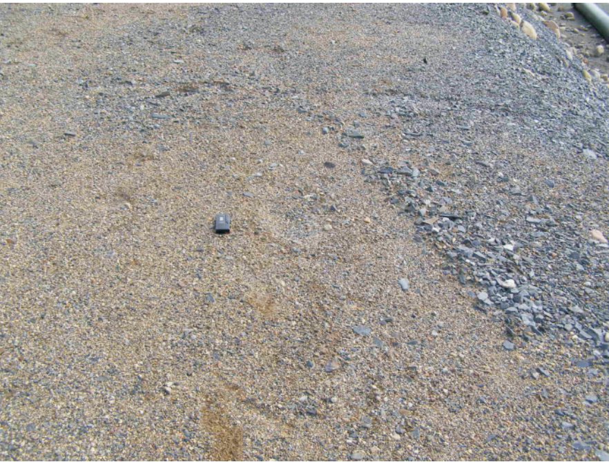
A view of a settlement spot that was noted during the 2007 inspection. It does not appear that any further movement has occurred in this area.
