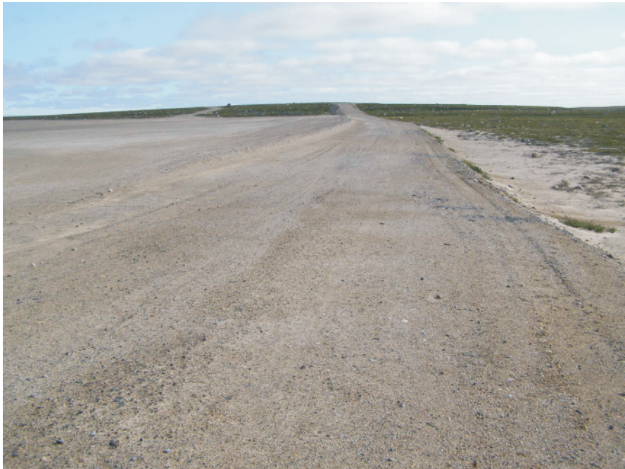
The crest of Dam 6 as seen from the right abutment. Note that the left side of the photo shows covered tailings and on the right some wind blown sand from the cover.
