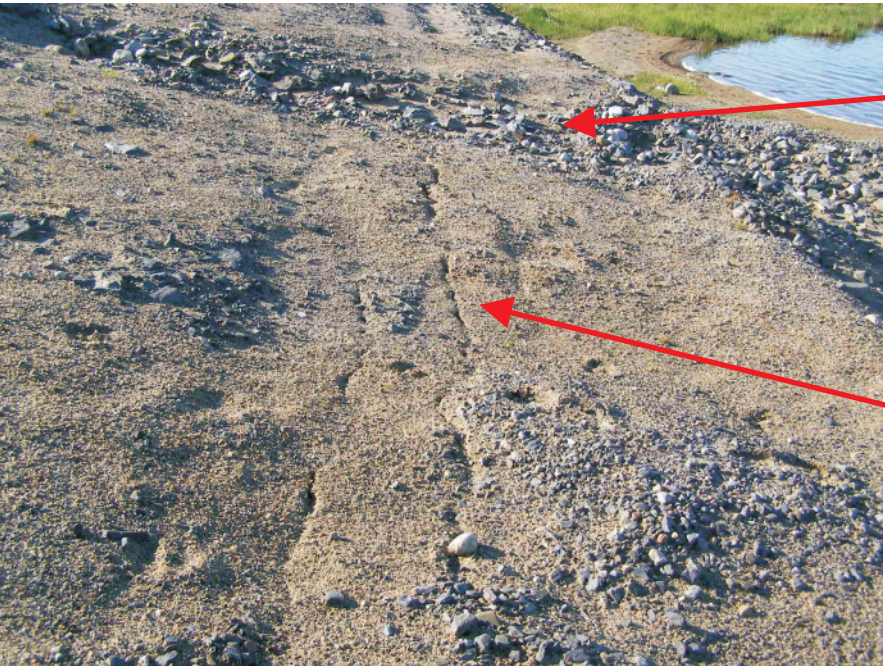
Tension cracks in the toe of Dam 3 near Boomerang Lake. These cracks are located directly adjacent to the erosion gully that can be seen towards the top of the photo.
