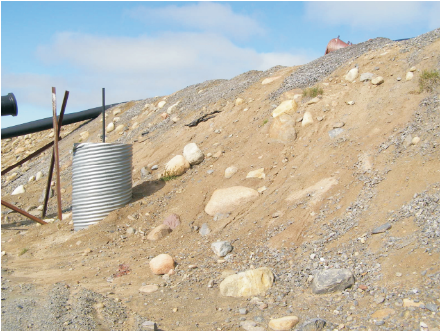
A close-up of the downstream face in the siphon area. Note the steep face and some minor erosion that is occurring on the face.
