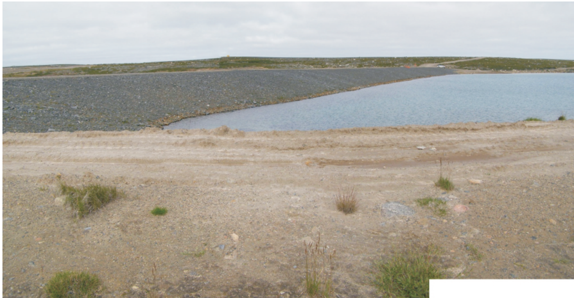
An overview of the upstream face of Dam 2 as seen from the left abutment. Note that the crest and upstream face are in good shape. A small wave erosion scarp is evident near the edge of the water.
