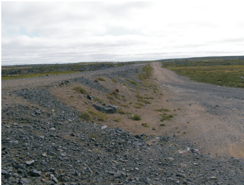
A view of the downstream face of Dam 1B taken from the right abutment. Note the vegetation that is beginning to take hold on the downstream face the dam. A number of animal burrows are evident on the downstream face.
