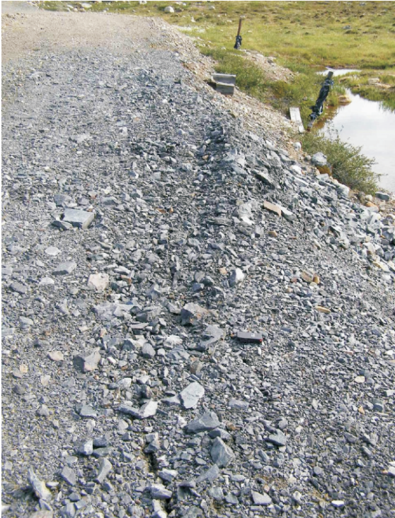
A view of a crack forming on the downstream side of the lower road. The outside shoulder is approximately 1.5 m to 2 m long and is softened from slumping due to erosion of the toe of the road.
