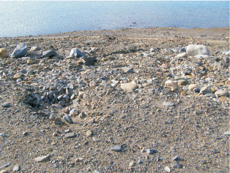
An area of erosion on the upstream face of Dam 4.
