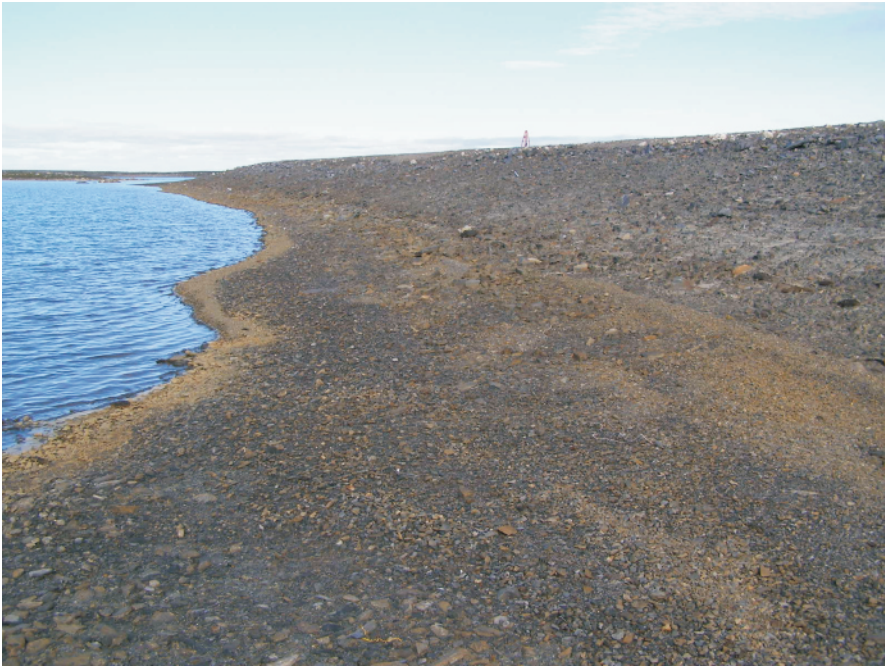
A view of the pond and dam interface on the upstream side of Dam 4. Note that the water level here appears to be about 0.5 m lower than seen in previous years, as evidenced by discolouration of the rock on the face of the dam.
