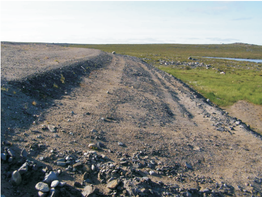
The downstream face of Dam 3. Generally the downstream face is in good condition.
