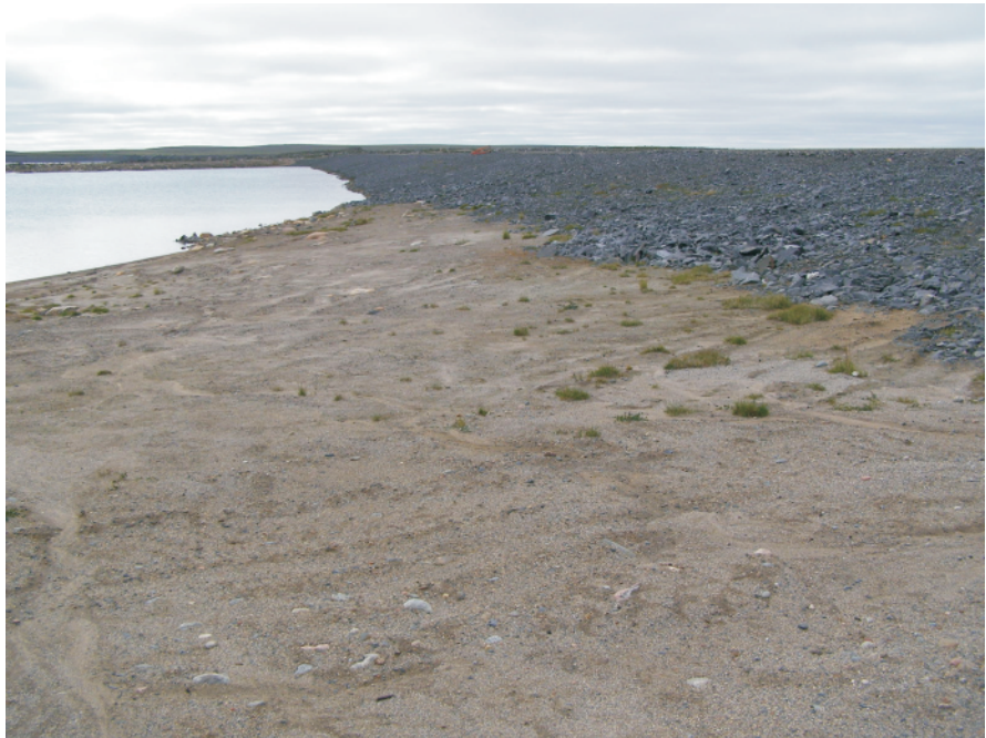
The upstream face of Dam 2 showing the grey riprap on the face of the dam.
