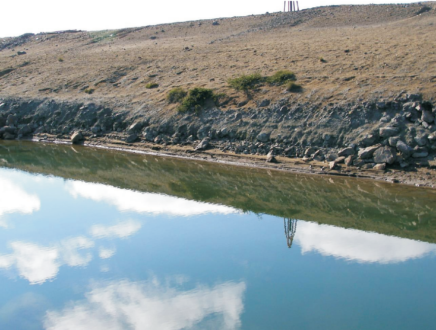
Wave erosion of the toe of Dam 4 near the right abutment.
