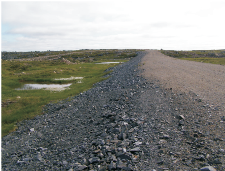
The upstream side and crest of Dam 1C showing the generally good condition and that there is no tailing water retained by this structure.
