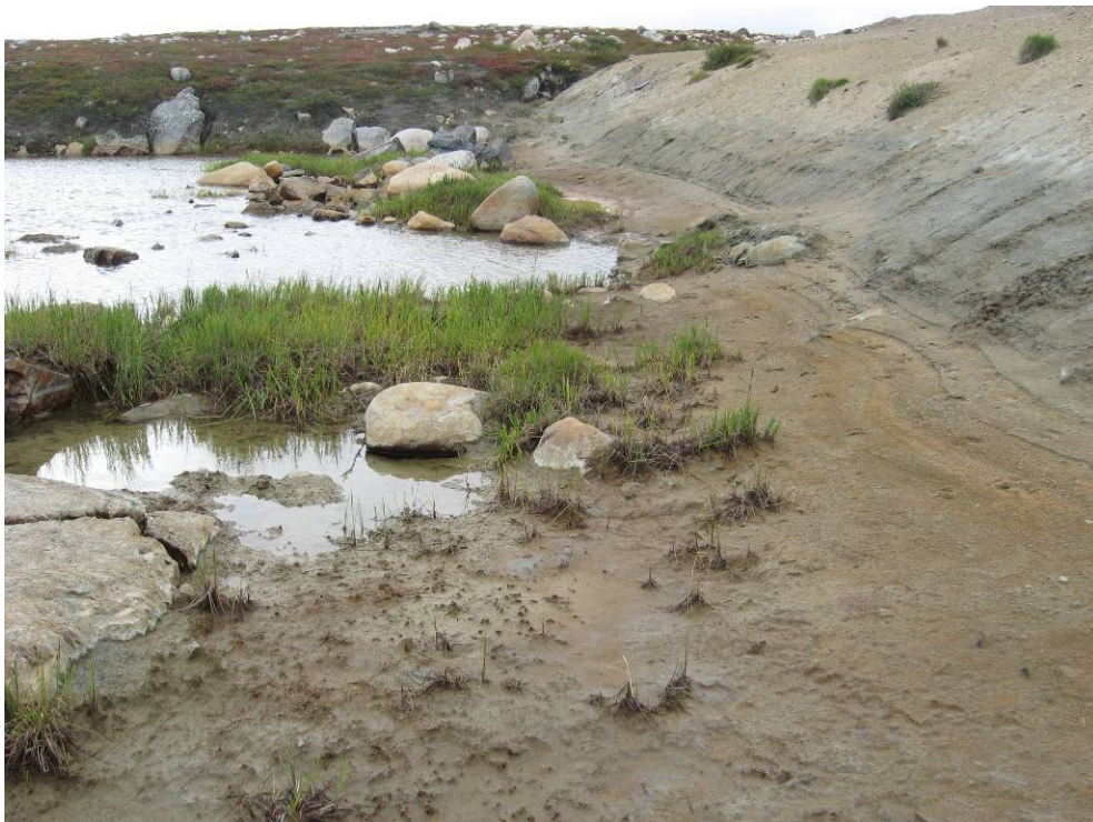
Dam 4: Downstream, note seepage line TBT Engineering Limited
