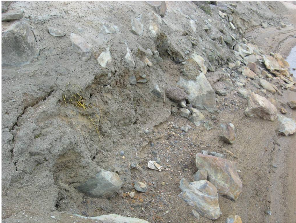
Dam 4: Downstream - sloughing zone
