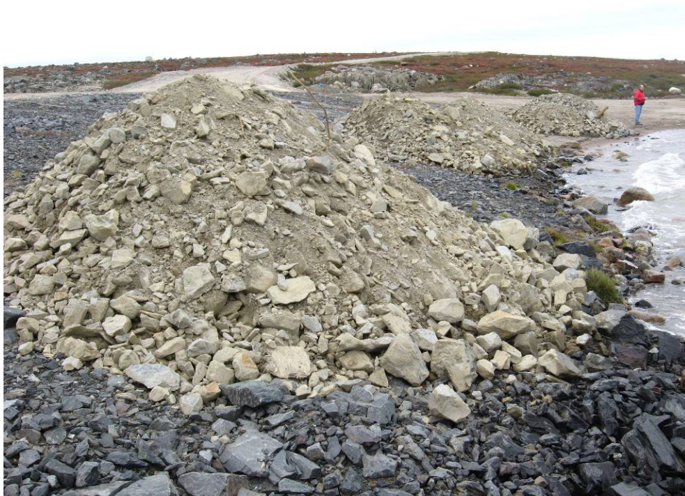
Dam 2: Upstream – New Riprap Material
