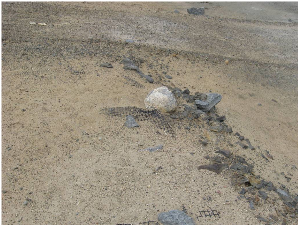
Dam 4: Downstream - exposed geogrid
