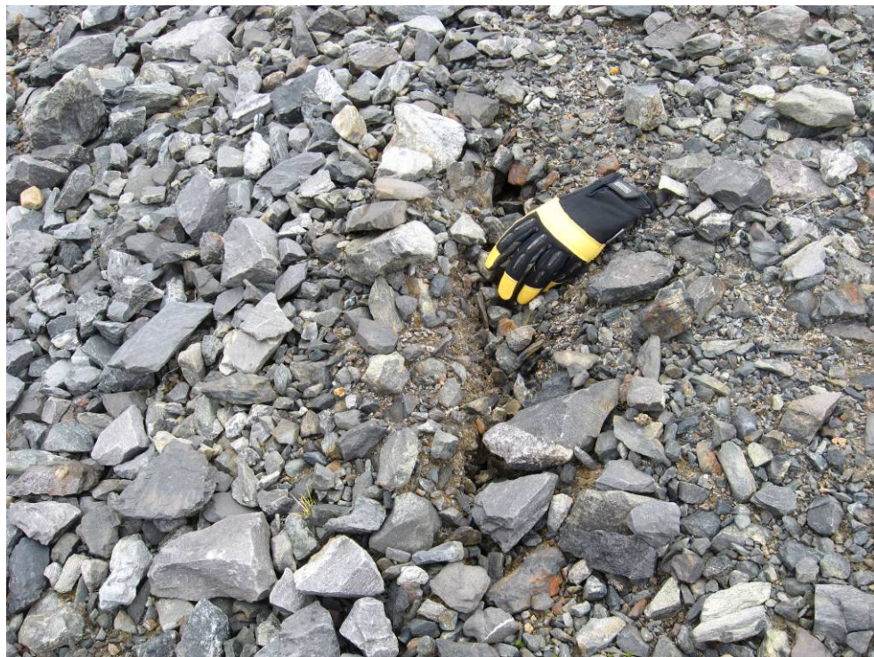
Dam 1C: Upstream-Minor Cracking
