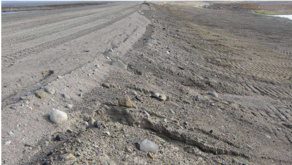
Dam 4: Downstream slope. Loose surface and erosion gullies on new infill between dam and cofferdam.
