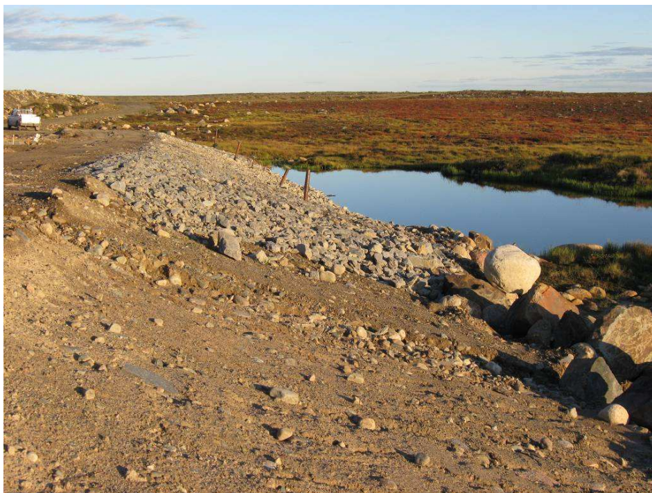
Dam 1A: Downstream Access Road toe Berm Looking South (Note, Downstream Slope Regraded and Covered with Riprap in 2010).
