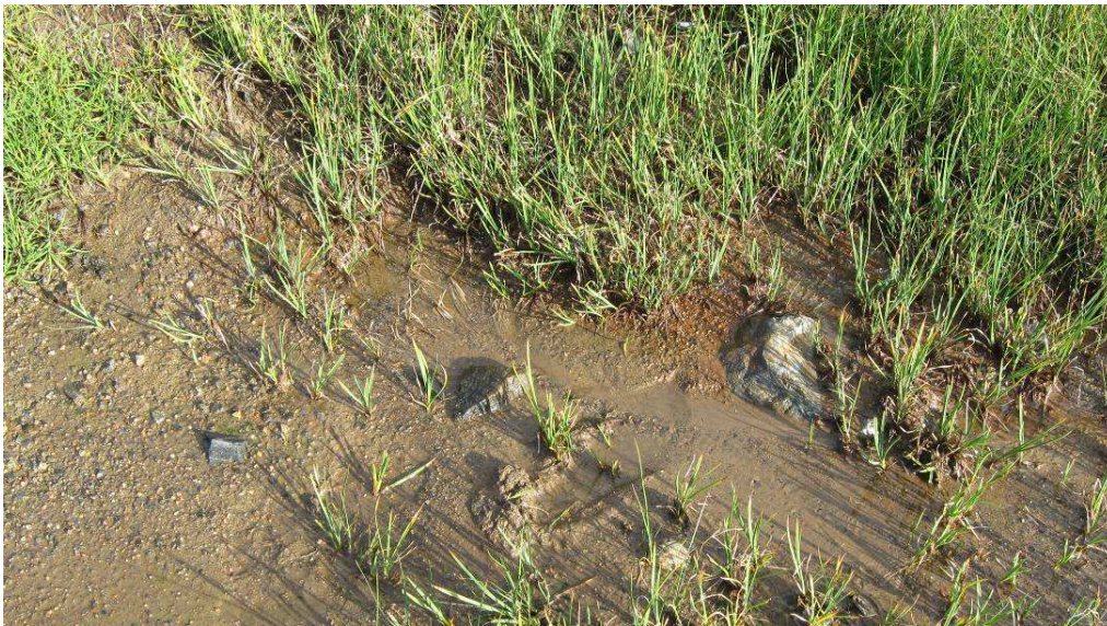
Dam 2: Downstream Toe (approx. 20 m South of D2-00-02) Clear Seepage at a Rate of Approx. 2 liters/min.
