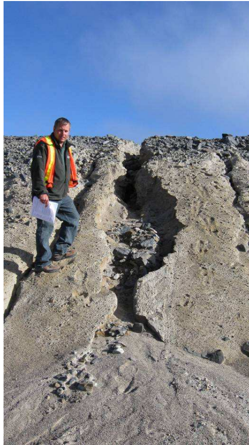
Dam 4: Downstream slope, east of cofferdam. Extensive erosion gullies
