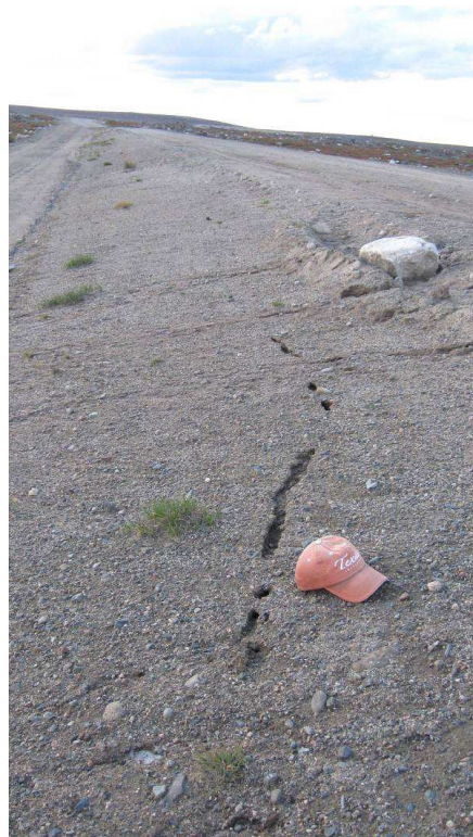
Downstream Slope (12 m long crack, middle of dam, 150 mm deep)
