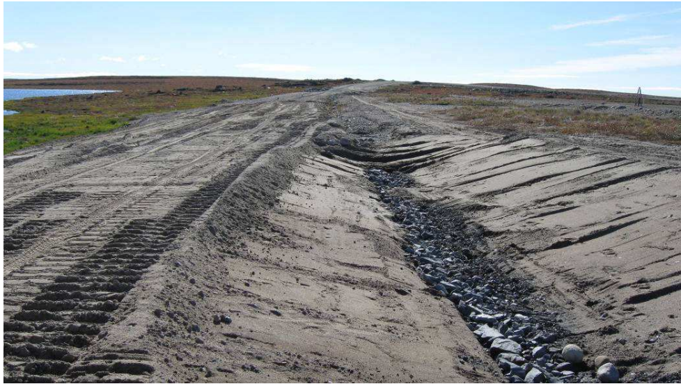
DAM 3: Upstream crest looking southeast. Loose fill on crest. End of ditch regrading. Ditching upstream of ditch regrading treatment contains some sediment.
