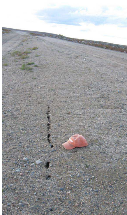
Downstream Slope (7 m long crack, 75 mm deep, north end of dam)
