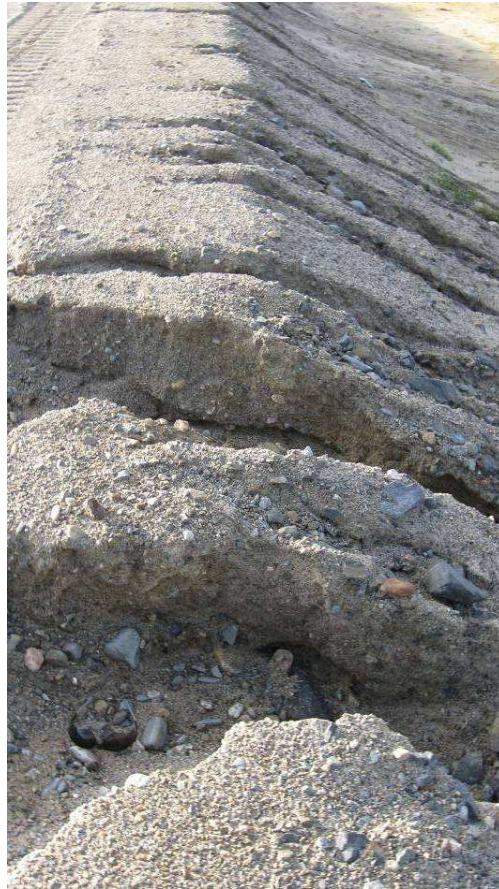
Dam 6: Down stream erosion gullies.
