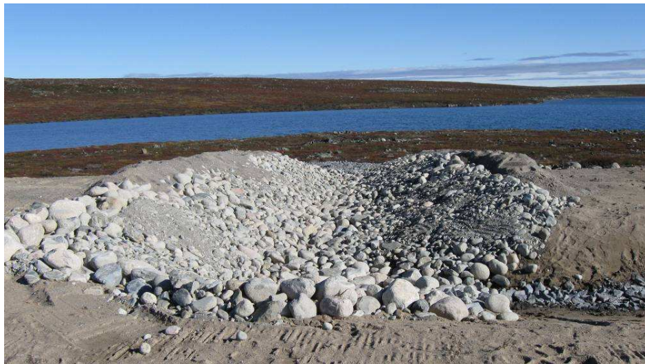
Dam 3: Spillway crossing dam at end of upstream ditch. Recently re-constructed with a grade of about 20H:1V (was specified at 30H:1V through the dam and 7H:1V along downstream slope). Through the dam crest, the new spillway has a channel base width of 2 m, not the specified 4 m. The spillway is lined with riprap and geotextile.
