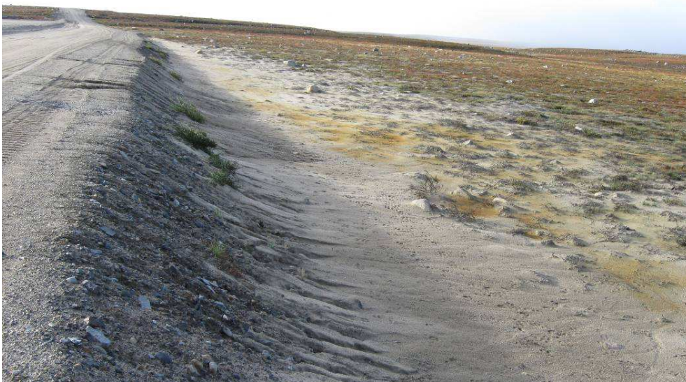
Dam 6: Downstream. Erosion gullies.
