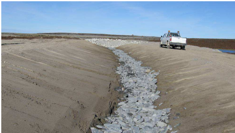
Dam 3: Upstream slope looking northwest at area of recent ditch regrading leading to reconstructed spillway. Ditch invert graded at about 3.5%. Tailings side ditch slope at about 4H:1, lake side ditch slope at about 3H:1V. Ditch invert lined with riprap (no geotextile observed).
