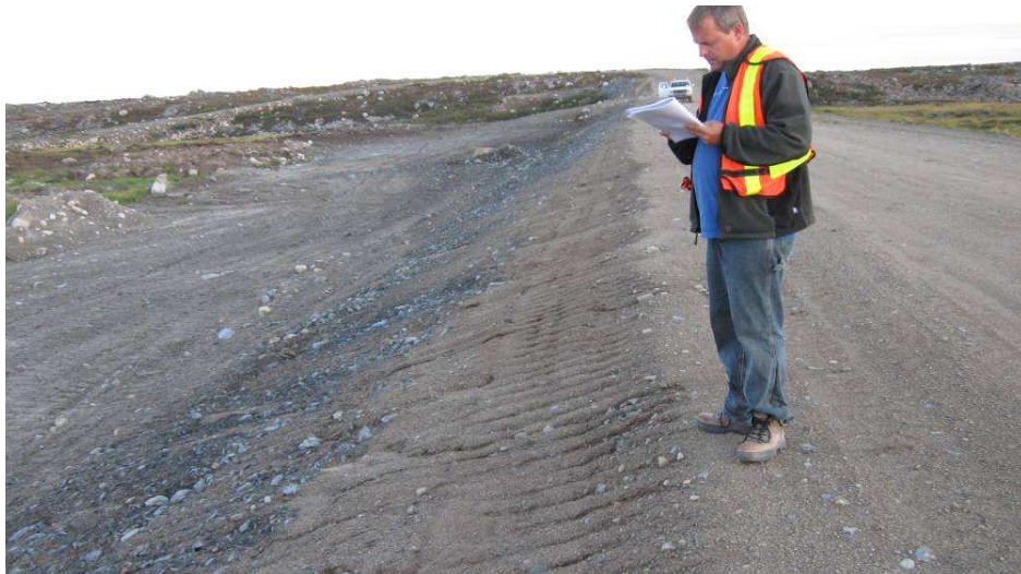
Dam 1C: Upstream (Minor Erosion Gullies on Shoulder of Granular Surfacing) Souther 2/3 of Upstream Slope Has Been Regraded/Extended with a Mixture of Rip Rap and Esker Material
