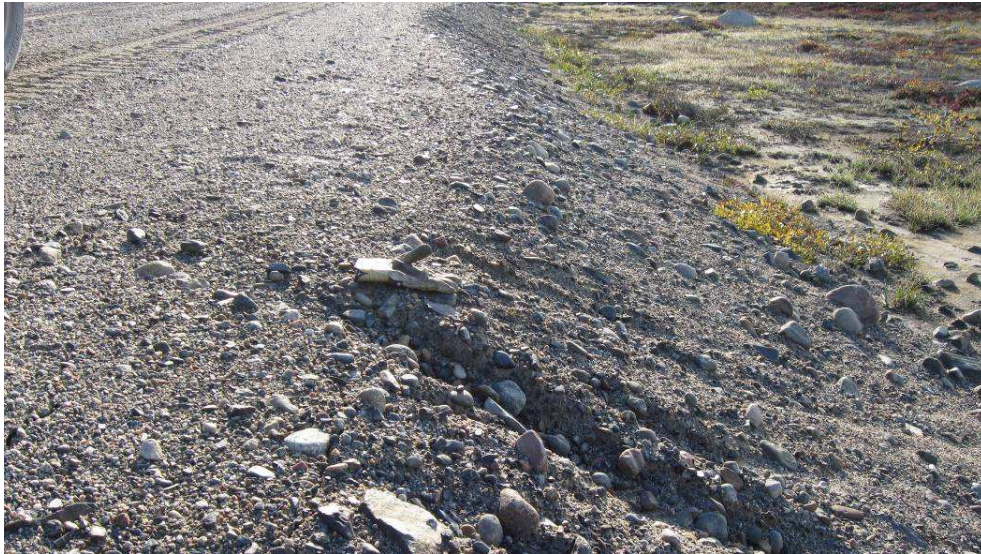
Dam 5: Downstream. Erosion gullies.
