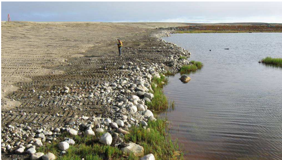
Dam 4: Downstream slope in area of old coffer dam (cobble stone).
