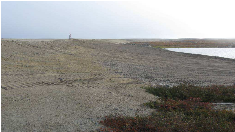
Dam 4: Downstream side, west end of dam. Area between Dam and downstream coffer dam recently infilled with esker material to mitigate seepage conditions note in last years inspection. Base on inspection of completed surface, fill appears to be placed in a loose manner.
