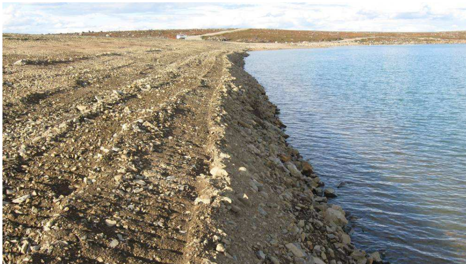
Dam 2: Upstream Slope Looking Northeast, Regraded with Riprap and Esker Material (graded at approx. 4.5H:1V upper portion, and at 1.5H:1V below about el. 483 m to pond level).
