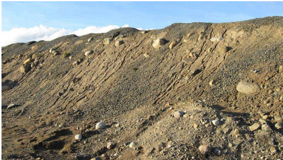
Dam 1A – Downstream Slope (south side of Siphons) Erosion Gullies – 2010
