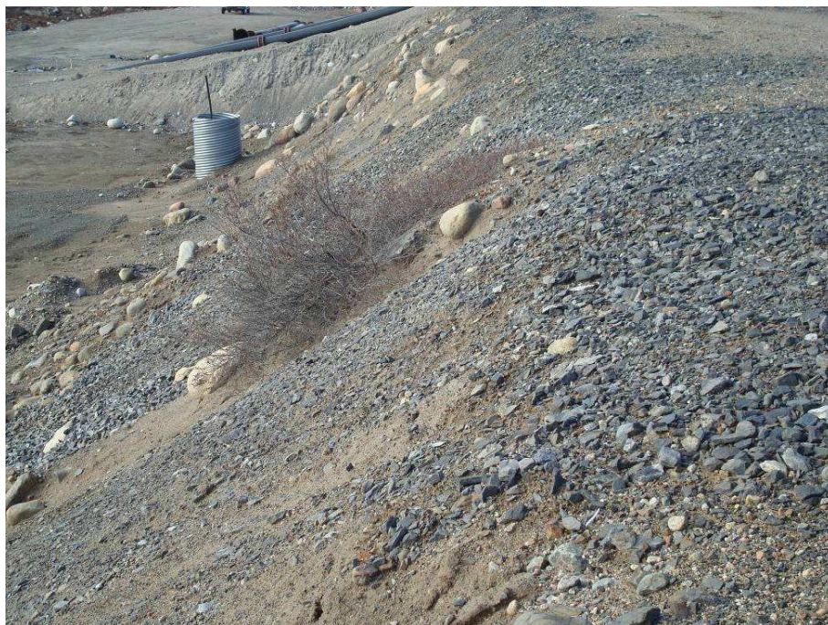
Downstream Crest: 1 m long narrow crack now filled in – 2011
