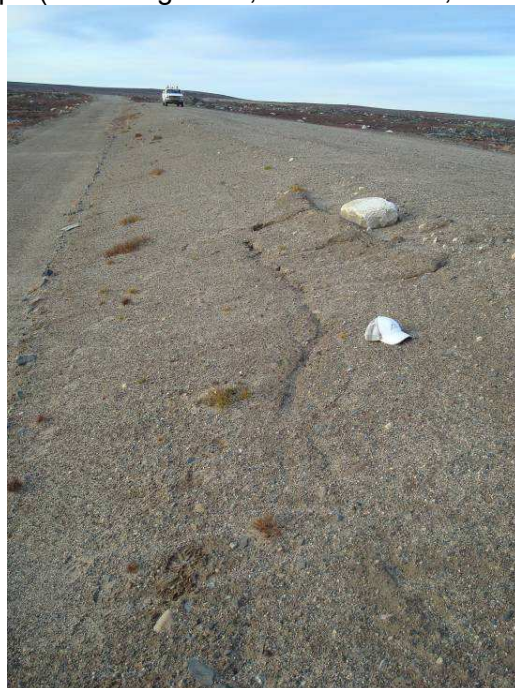
Downstream Slope (crack now partially in-filled) – 2011
