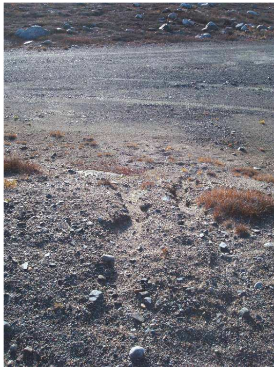
Downstream Slope: Erosion Gullies – 2011
