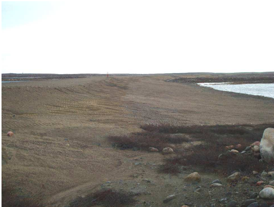
Dam 4: Downstream side, west end of dam. Some erosion gullies evident. Surface material in loose condition. No seepage observed. – 2011
