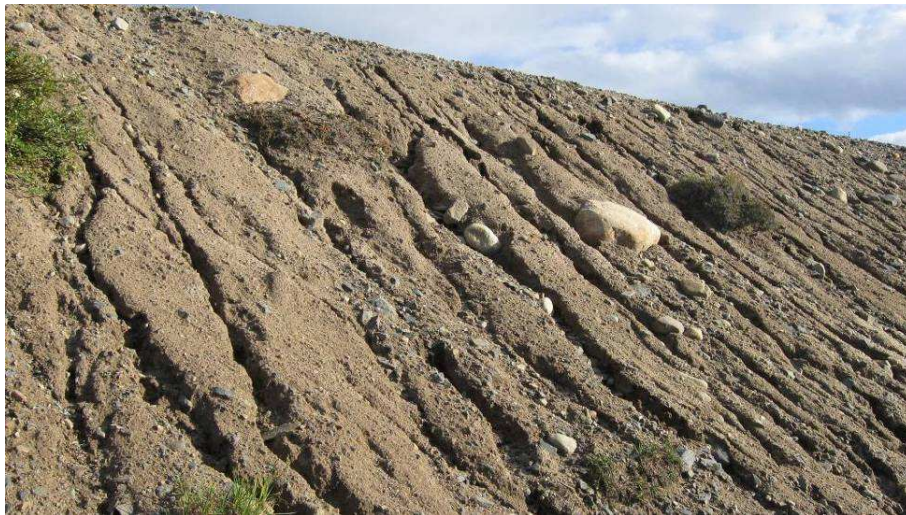
Dam 2: Downstream Slope Erosion Gullies and Rills – 2010
