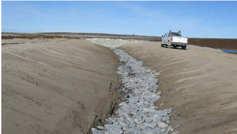
Dam 3: Upstream slope looking northwest at area of last year's ditch regrading leading to reconstructed spillway. Ditch invert lined with riprap (no geotextile observed). – 2010
