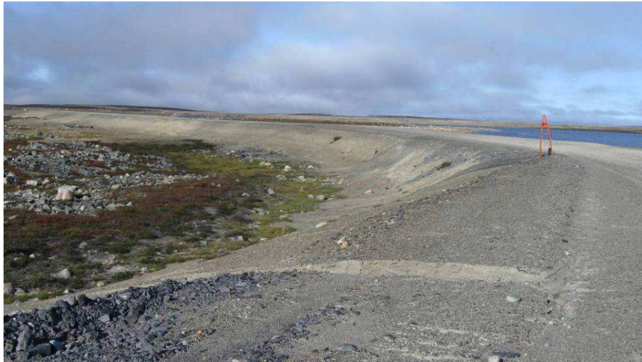
Dam 4: Downstream slope, east of cofferdam (looking west). Extensive erosion gullies – 2010
