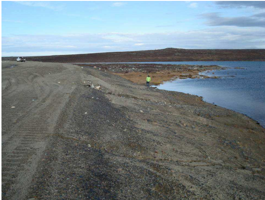
Erosion Gullies on Downstream Slope – 2011
