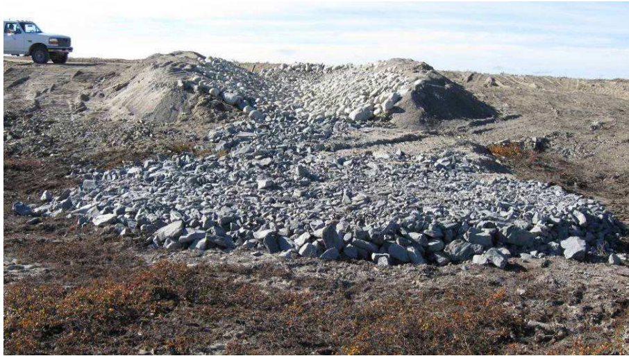
Dam 3: Downstream side of spillway (splash pad) constructed last year. Spillway side slope constructed at about 2.5H:1V (steeper than 3H:1V specified). Slopes on the outside of the spillway channel are also steeper than specified. – 2010
