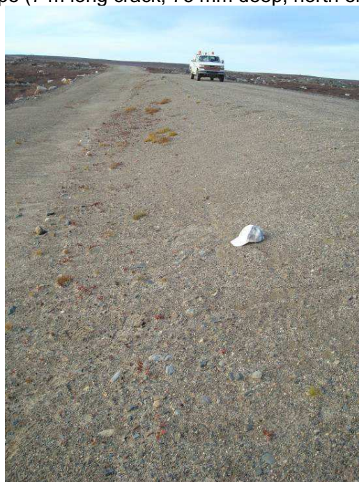
Downstream Slope (crack now in-filled) – 2011
