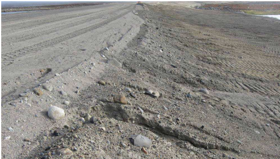
Dam 4: Downstream slope. Loose surface and erosion gullies on new infill. – 2010
