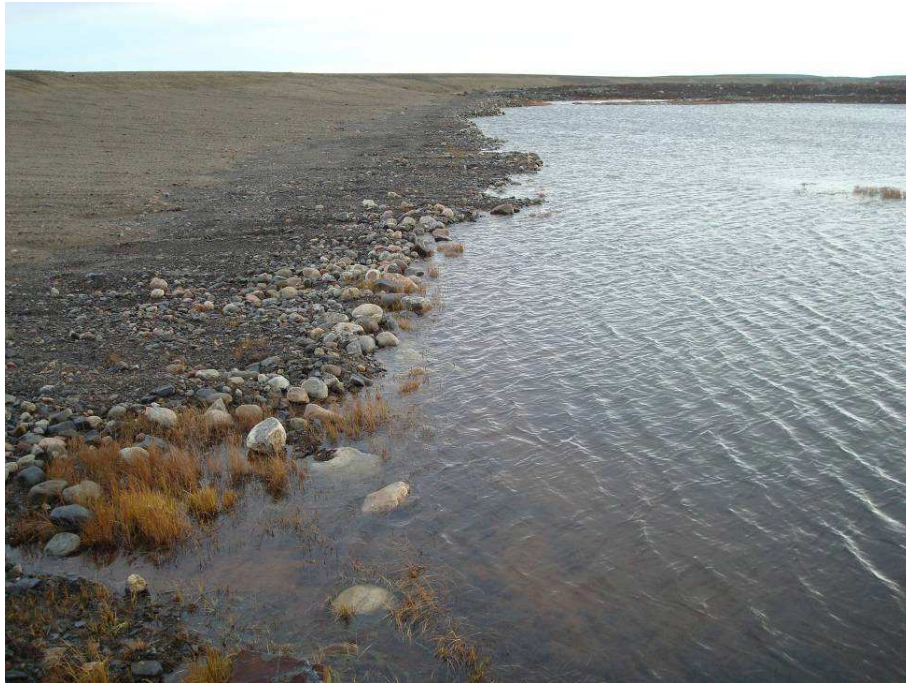
Dam 4: Downstream slope in area of old coffer dam (cobble stone). Note slightly higher downstream lake level. – 2011
