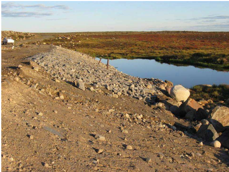
Dam 1A: Downstream Access Road Toe Berm Looking South – 2010
