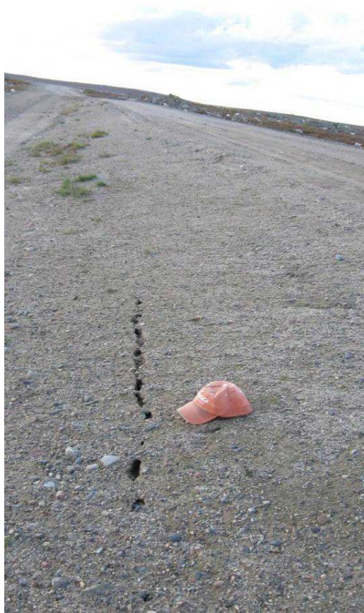
Downstream Slope (7 m long crack, 75 mm deep, north end of dam) – 2010
