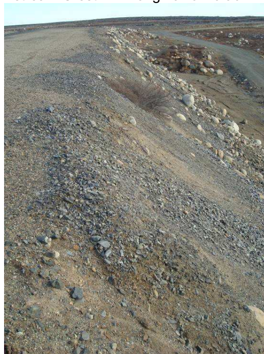
Downstream Crest: 1 m long narrow crack now in filled – 2011
