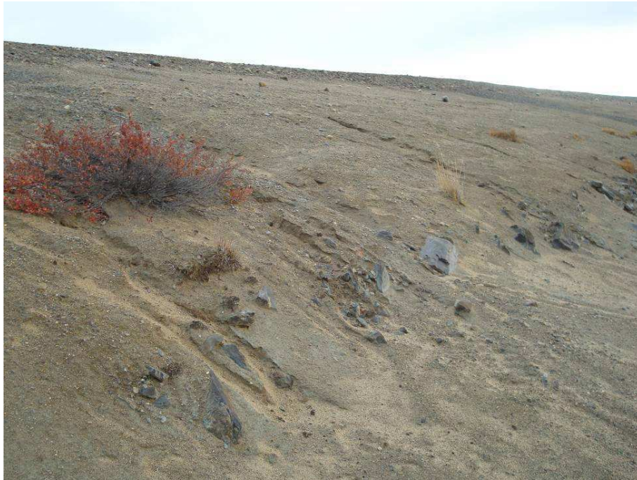
Dam 4: Downstream slope, east of cofferdam. Extensive erosion gullies (now partially in-filled) – 2011
