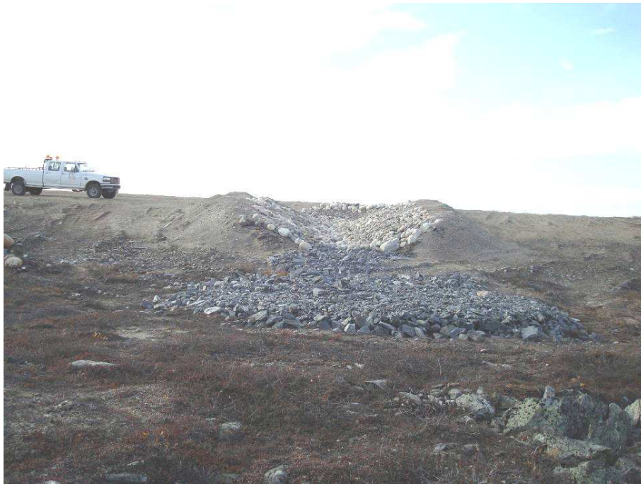
Dam 3: Downstream side of spillway (splash pad) – 2011
