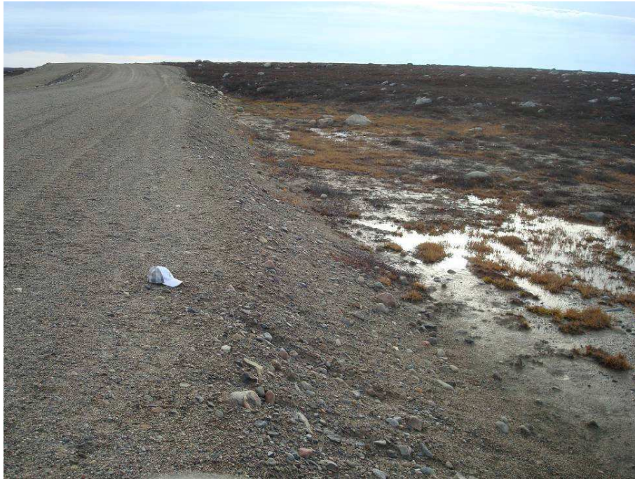
Dam 5: Downstream. Erosion gullies (partially in-filled). – 2011
