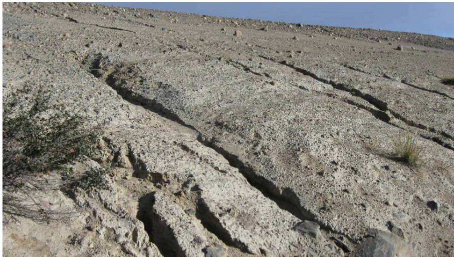
Dam 4: Downstream slope, east of cofferdam. Extensive erosion gullies – 2010
