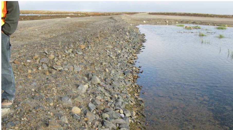
Dam 6: Upstream. Riprap in area of small pond. – 2010
