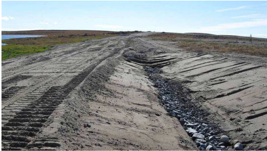
DAM 3: Upstream crest looking southeast. Loose fill on crest. End of ditch regrading. Ditching upstream of ditch regrading treatment contains some sediment. – 2010
