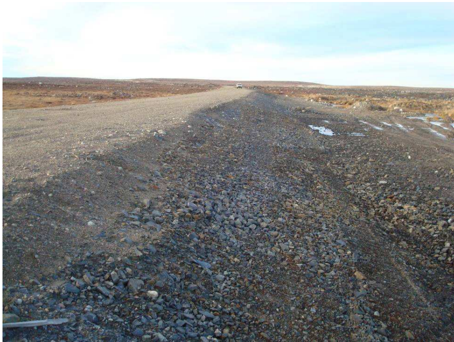
Dam 1C: Upstream (Minor Erosion Gullies on Shoulder of Granular Surfacing) – 2011
