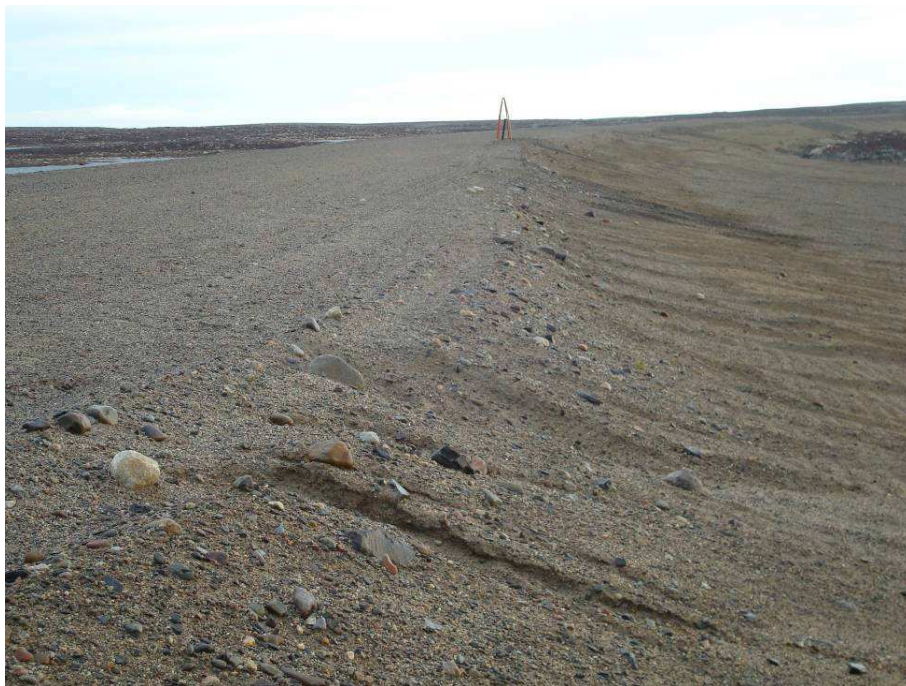
Dam 4: Downstream slope. Loose surface and erosion gullies (partially in-filled) on new infill. – 2011
