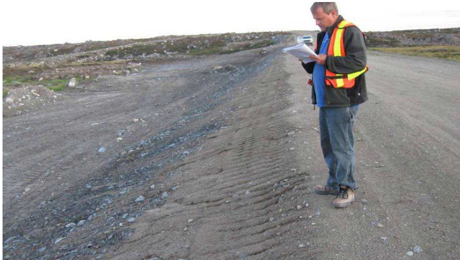
Dam 1C: Upstream (Minor Erosion Gullies on Shoulder of Granular Surfacing) Southern 2/3 of Upstream Slope Has Been Regraded/Extended with a Mixture of Rip Rap and Esker Material – 2010
