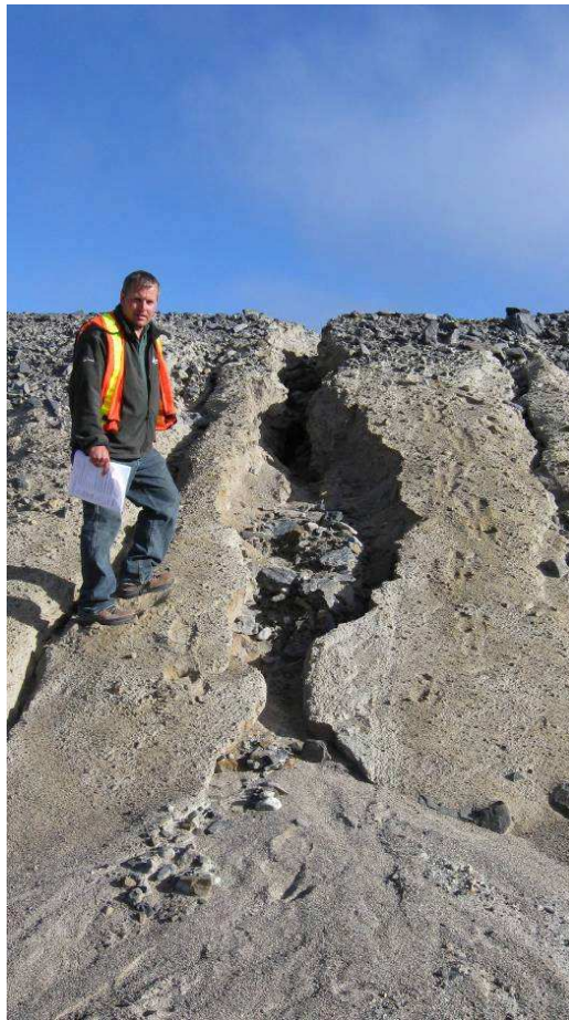
Dam 4: Downstream slope, east of cofferdam. Extensive erosion gullies - 2010
