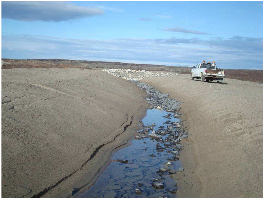
Dam 3: Upstream slope looking northwest at area of last year's ditch regrading leading. Some scour and standing water. – 2011
