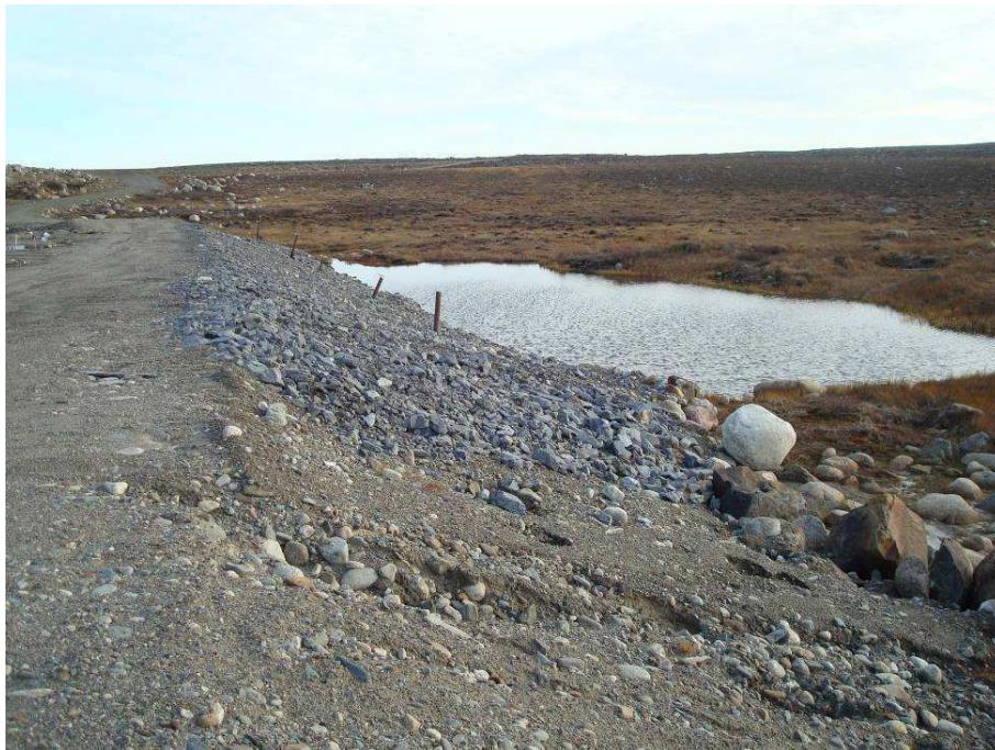
Dam 1A: Downstream Access Road Toe Berm Looking South – 2011
