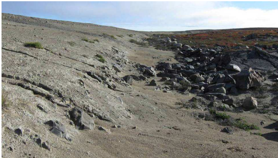
Dam 4: Downstream slope, east of cofferdam. Extensive erosion gullies (exposed geogrid). – 2010
