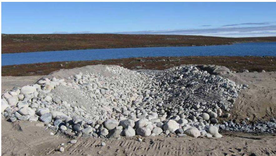
Dam 3: Spillway crossing dam at end of upstream ditch. Re-constructed last year with a grade of about 20H:1V (was specified at 30H:1V through the dam and 7H:1V along downstream slope). Through the dam crest, the new spillway has a channel base width of 2 m, not the specified 4 m. The spillway is lined with riprap and geotextile. – 2010
