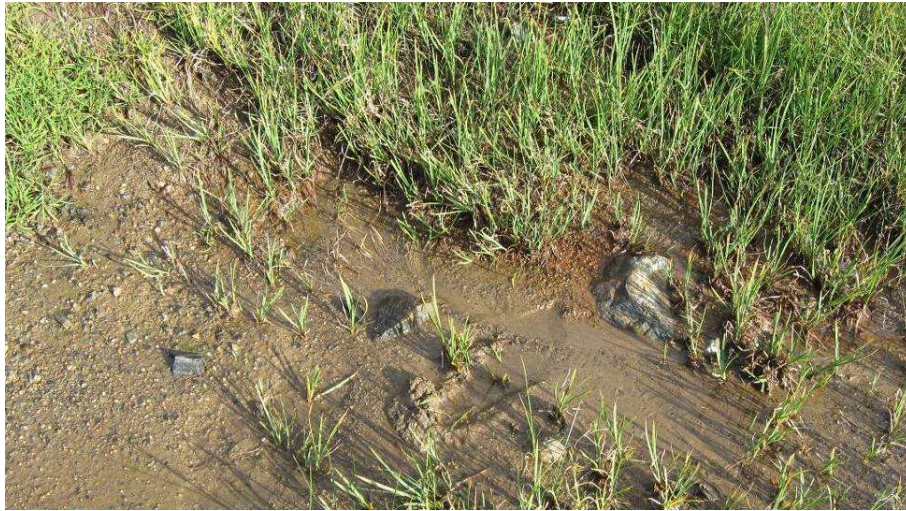
Dam 2: Downstream Toe (approx. 20 m South of D2-00-02) Clear Seepage at a Rate of Approx. 2 litres/min. – 2010
