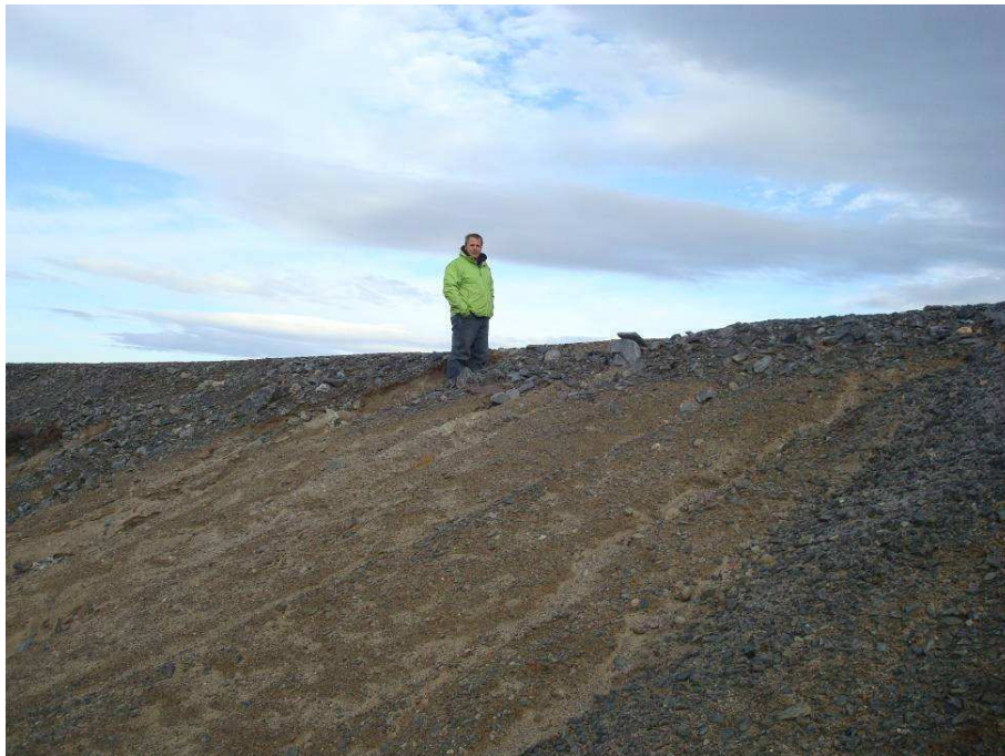
Dam 4: Downstream slope, east of cofferdam. Extensive erosion gullies – 2011
