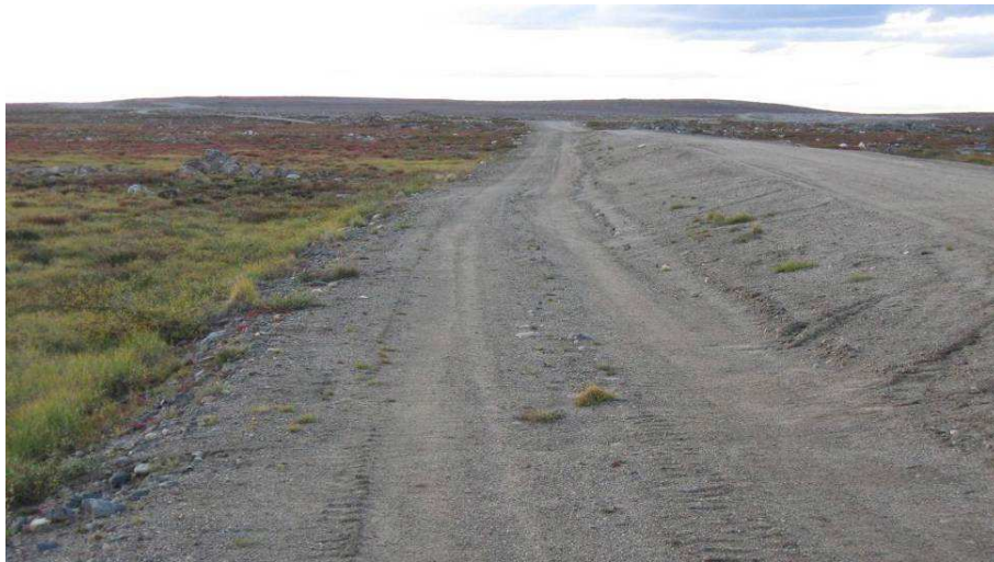
Dam 1C: Downstream Slope (Some Minor Erosion Gullies) – 2010
