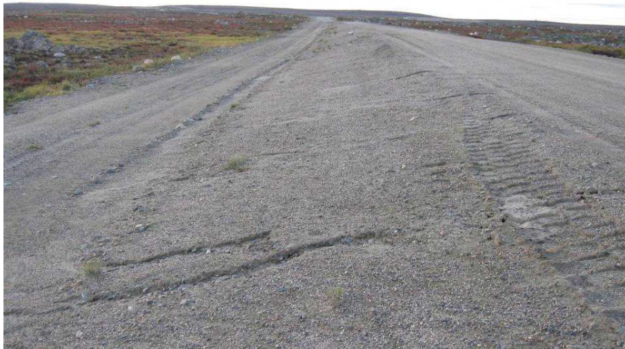
Dam 1C: Downstream Slope (Some Minor Erosion Gullies) – 2010
