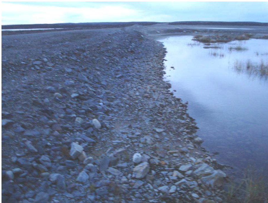
Dam 6: Upstream. Riprap in area of small pond. – 2011
