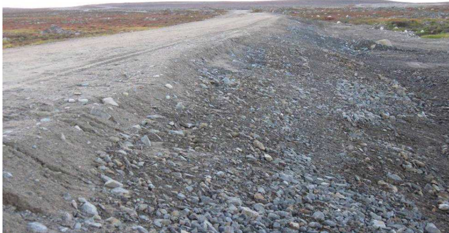
Dam 1C: Upstream (Minor Erosion Gullies on Shoulder of Granular Surfacing) – 2010
