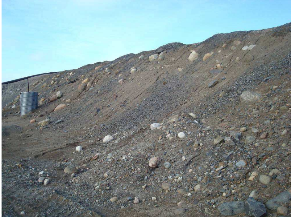
Dam 1A – Downstream Slope (south side of Siphons) Erosion Gullies – 2011
