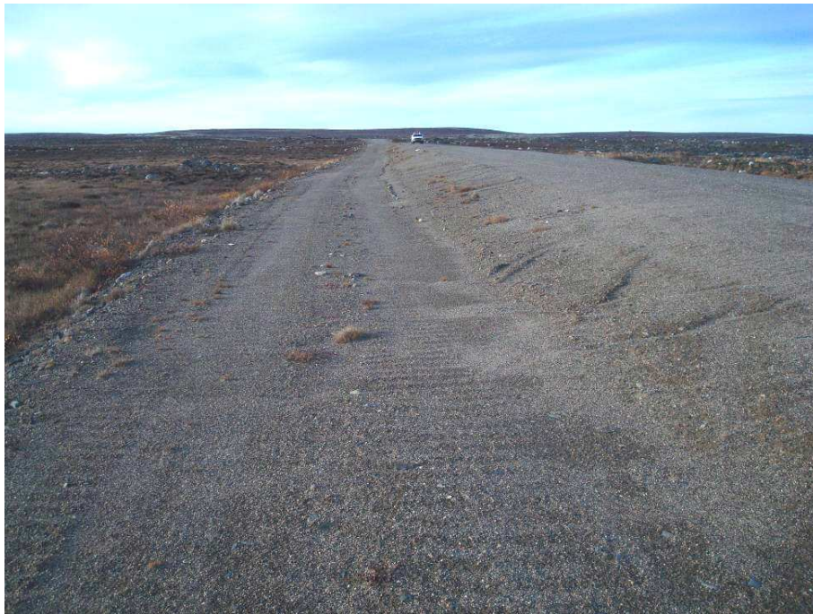
Dam 1C: Downstream Slope (Some Minor Erosion Gullies) – 2011
