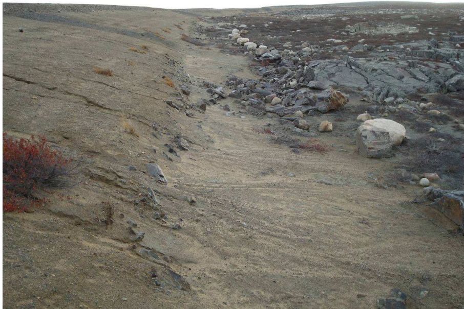
Dam 4: Downstream slope, east of cofferdam. Extensive erosion gullies (now partially in-filled). – 2011
