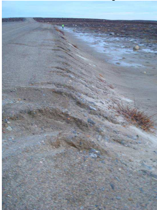
Dam 6: Down stream erosion gullies – 2011
