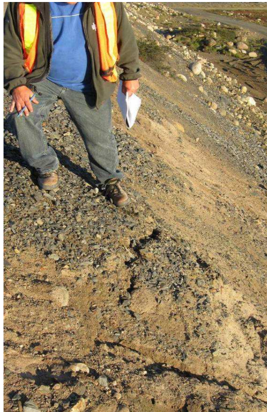
Downstream Crest: 1 m long narrow crack – 2010
