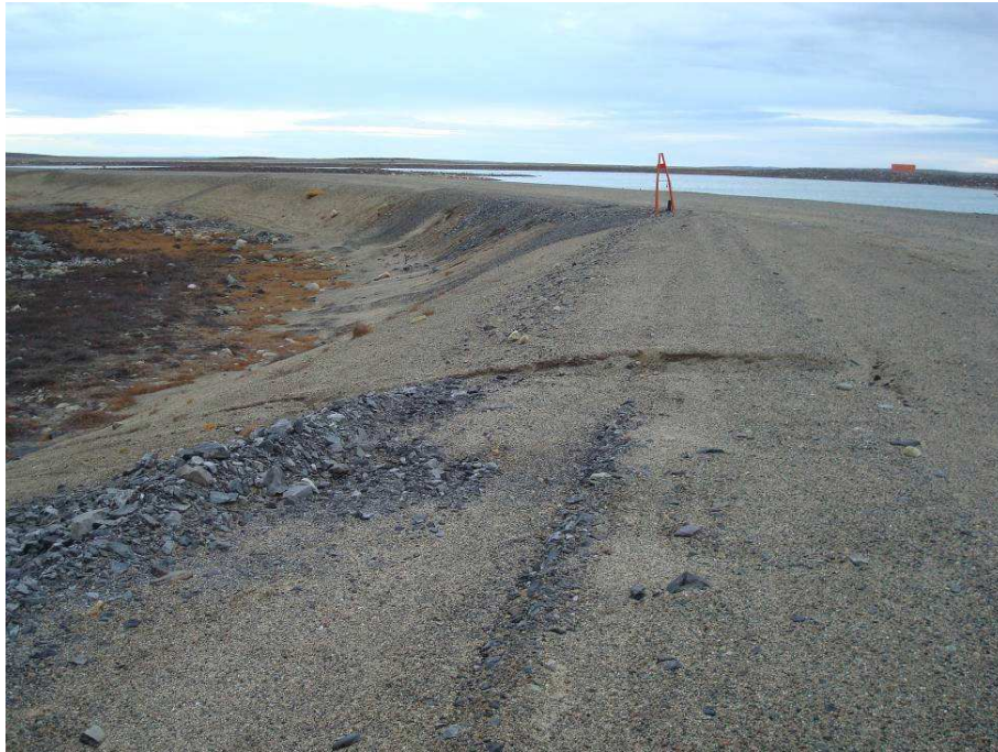
Dam 4: Downstream slope, east of cofferdam (looking west). Extensive erosion gullies – 2011
