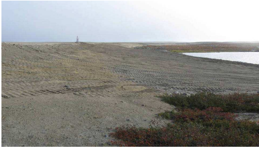
Dam 4: Downstream side, west end of dam. Area between Dam and downstream coffer dam infilled (last year) with esker material to mitigate seepage conditions. – 2010
