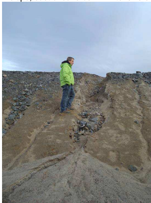
Dam 4: Downstream slope, east of cofferdam. Extensive erosion gullies - 2011
