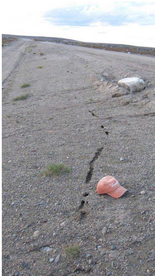
Downstream Slope (12 m long crack, middle of dam, 150 mm deep) – 2010
