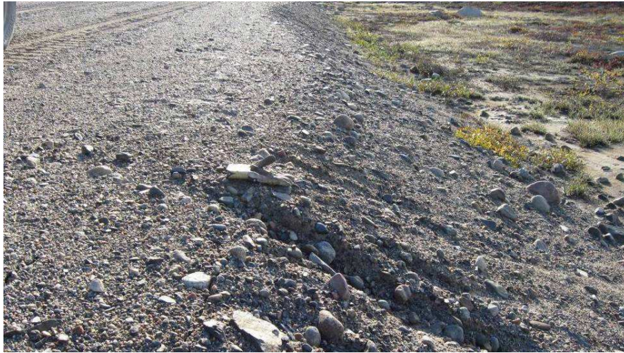
Dam 5: Downstream. Erosion gullies. – 2010
