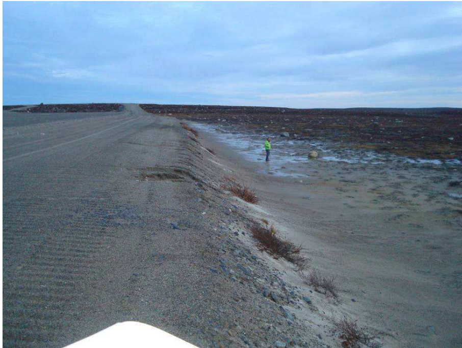
Dam 6: Downstream. Erosion gullies and Standing Water Near Toe. – 2011
