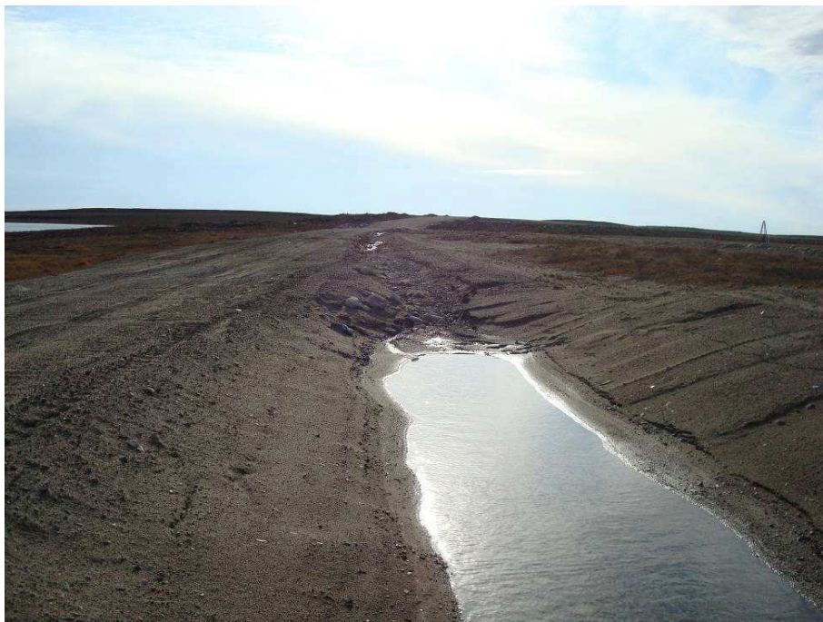
DAM 3: Upstream crest looking southeast. Loose fill on crest. End of ditch regrading. Standing water. Ditching upstream of ditch regrading treatment contains some sediment. – 2011
