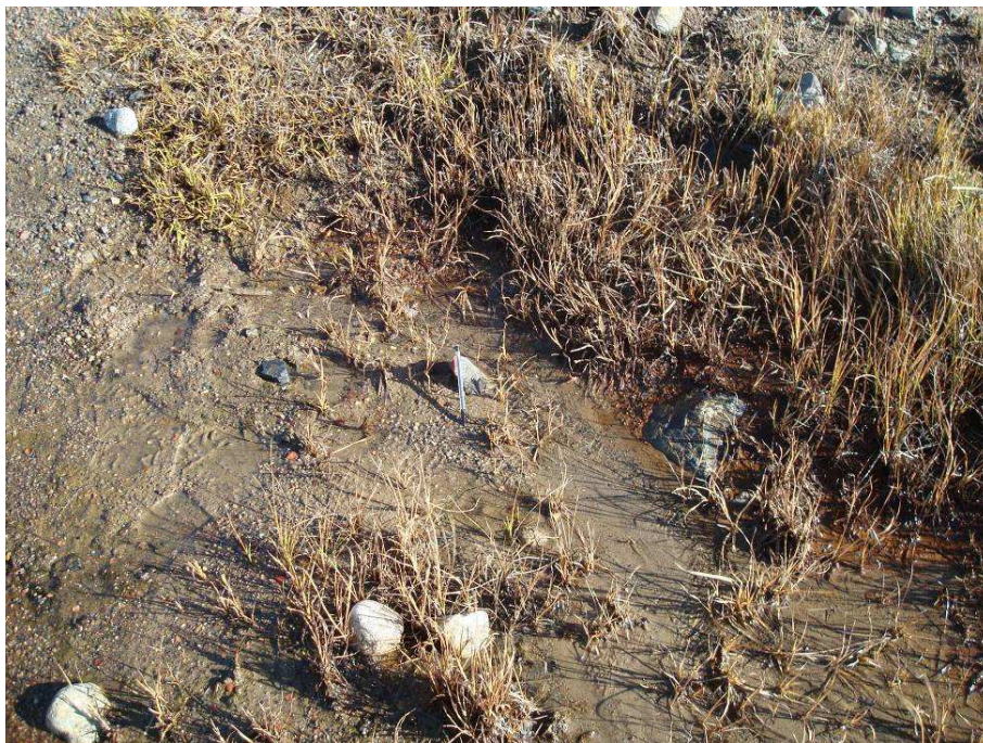
Dam 2: Downstream Toe (approx. 20 m South of D2-00-02) Clear Seepage at a Rate of Approx. 4 litres/min. – Th2011
