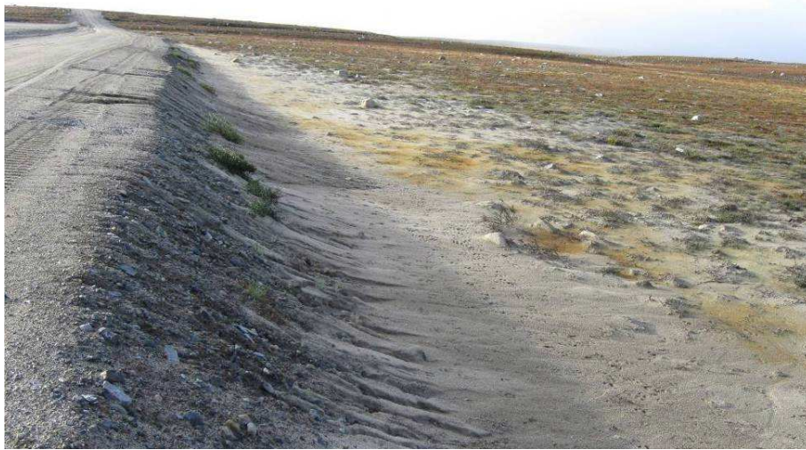
Dam 6: Downstream. Erosion gullies. – 2010
