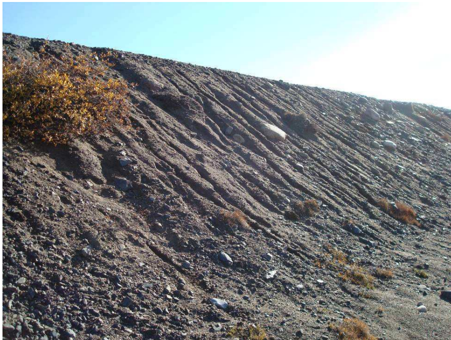
Dam 2: Downstream Slope Erosion Gullies and Rills – 2011
