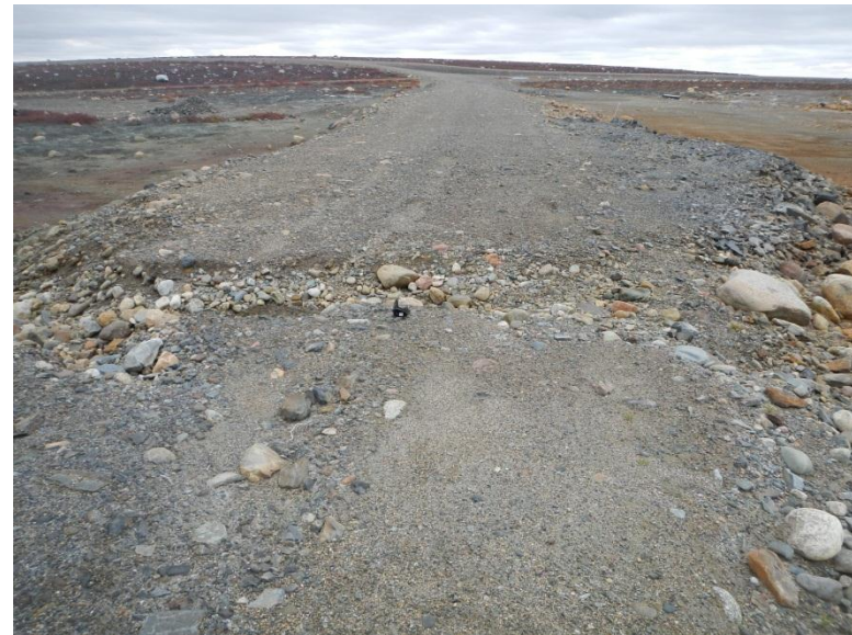
Lupin Dam L erosion channel
