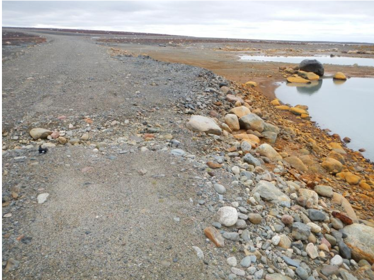
Lupin Dam L erosion channel, Cell 3 view
