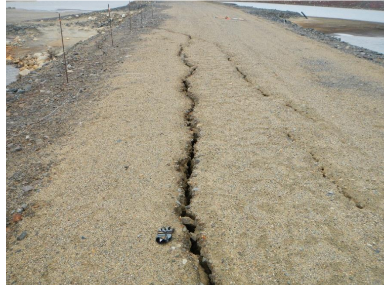
Lupin Dam M tension crack
