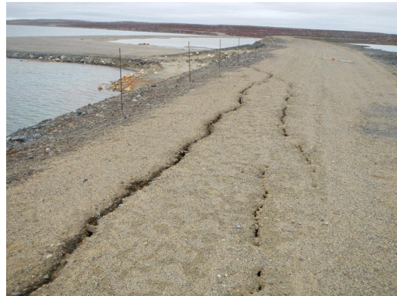
Lupin Dam M tension crack
