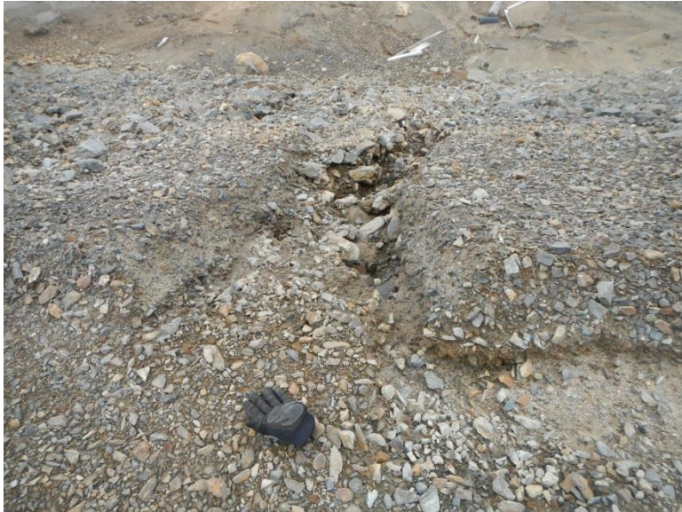
Lupin Dam L crest erosion
