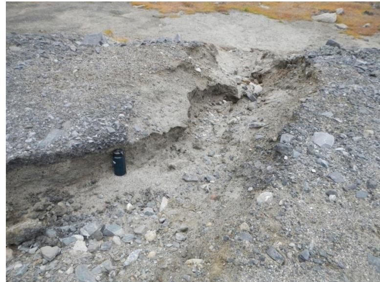
Lupin Dam 4 eastern DS slope erosion
