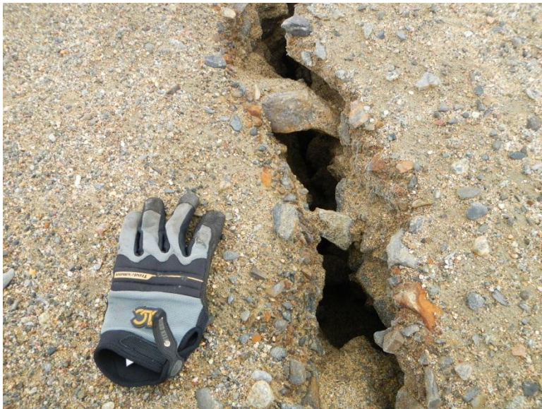
Lupin Dam M tension crack
