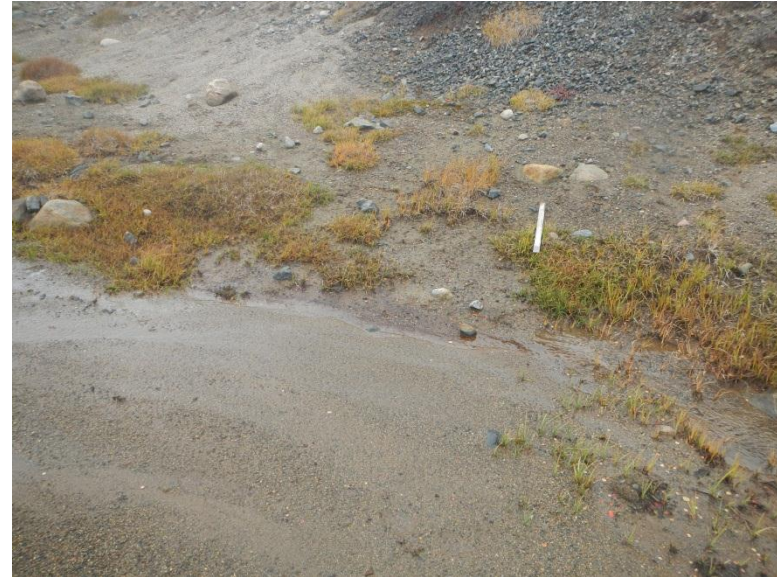
Lupin Dam 2 North abutment seepage
