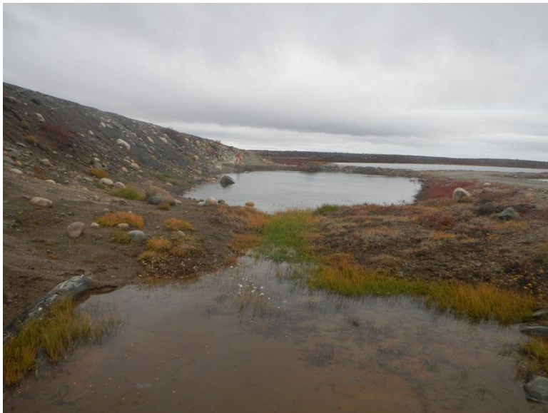
Lupin Dam 2 North abutment seepage
