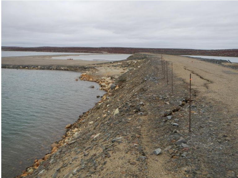
Lupin Dam M tension crack
