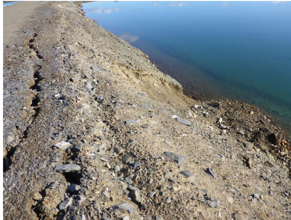
Photo 32: Close up view of the new tension cracks observed in 2014, in face of the dam toward Pond 1.
