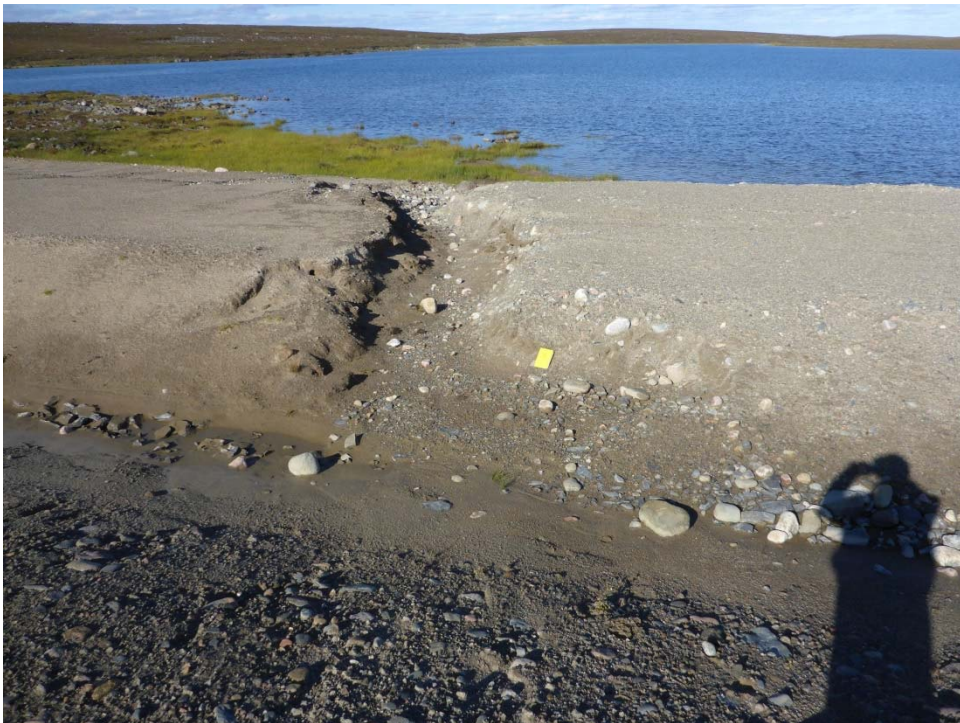
Photo 22: looking north at the erosion damage on crest of Dam 3.
