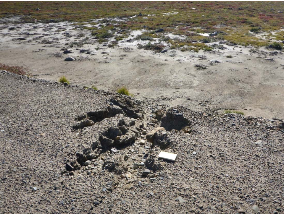
Photo 14: Close up look at one of the large erosion gully in Dam 6.
