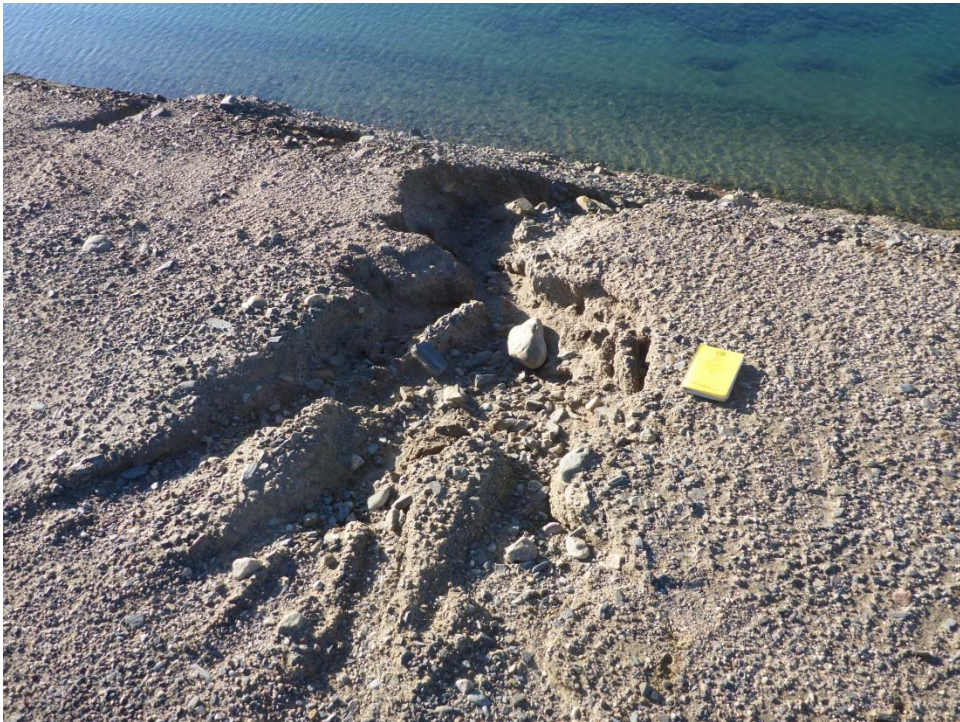
Photo 41: Close up view of erosion gully in Dam K facing pond 2.
