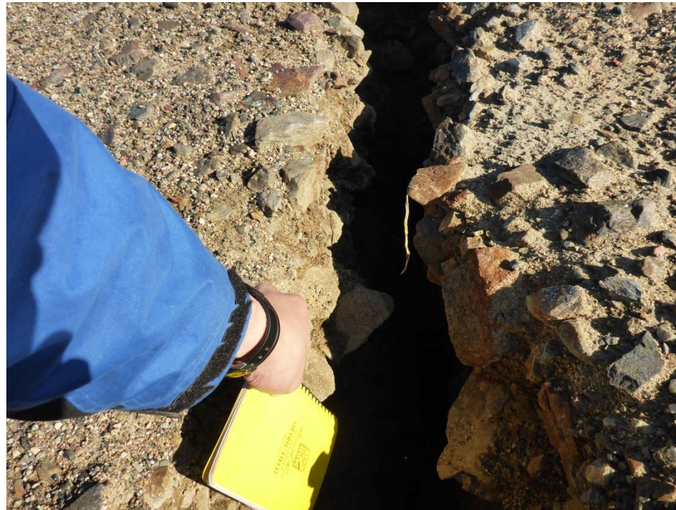
Photo 35: Close up view of the new tension cracks observed in 2014, in face of the dam toward Pond 1.
