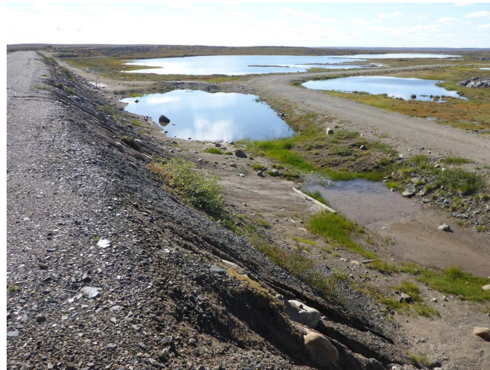
Photo 2: Looking south at the seepage collection ponds at toe of Dam 2.
