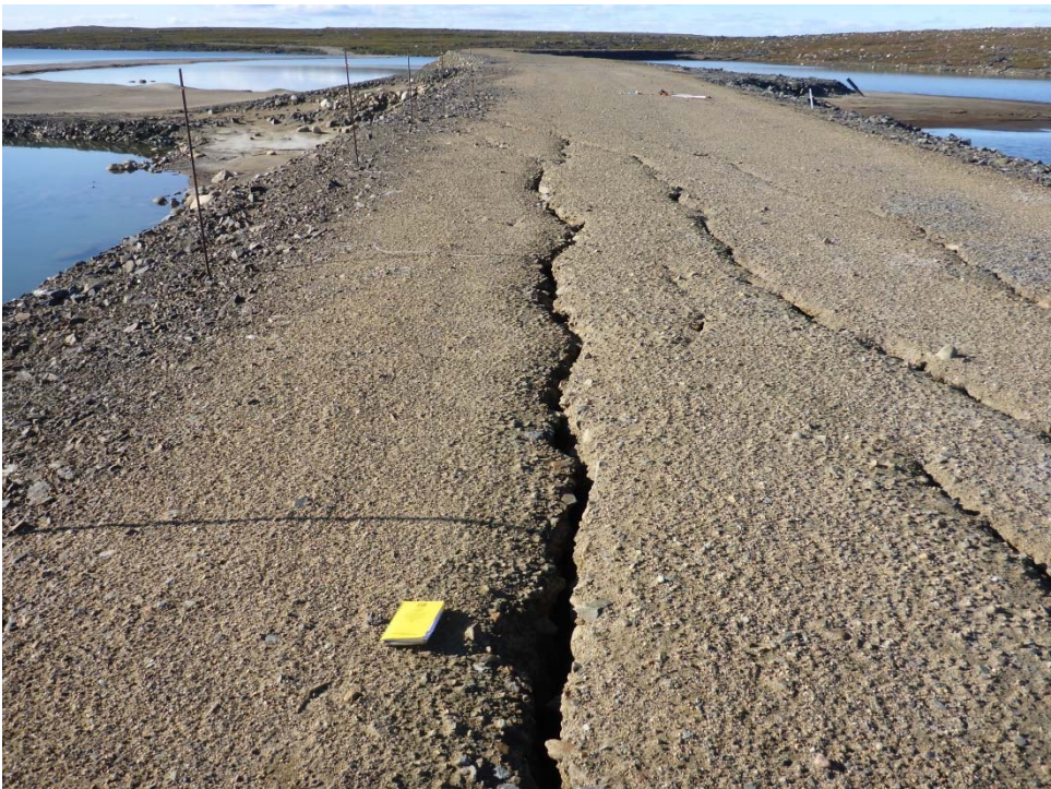
Photo 29: Close up view of the original tension cracks on Dam M.
