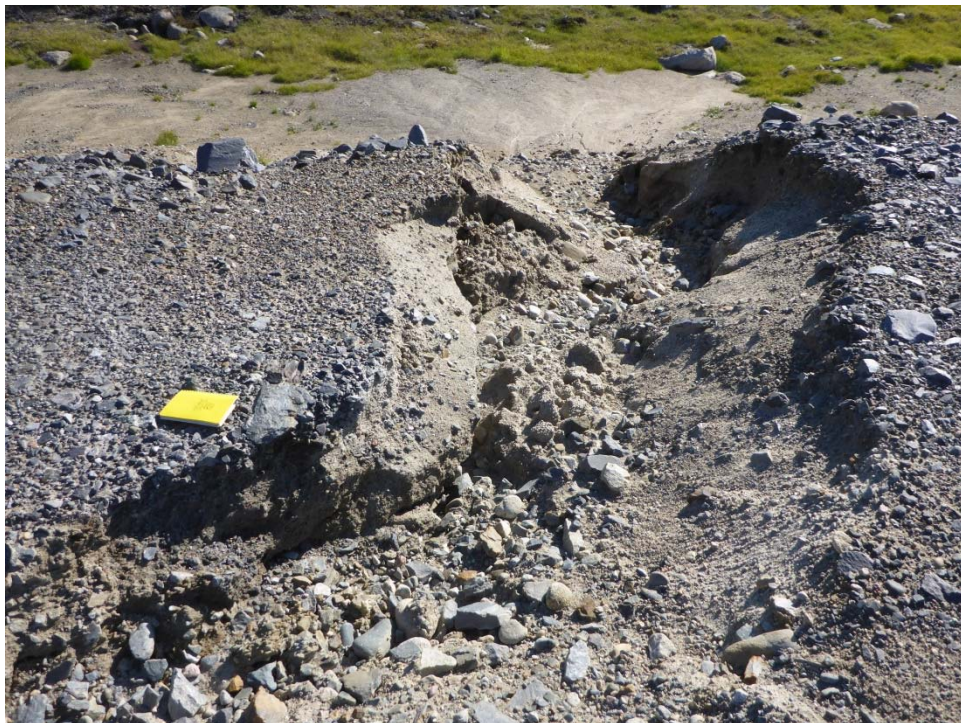
Photo 21: Close up of erosion gully in Dam 4.
