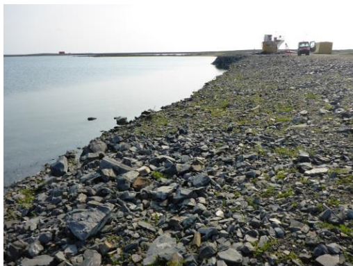
Photo 4: Looking south at Dam 1A upstream face.
