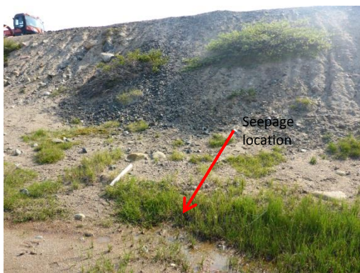
Photo 1: Seepage in the north abutment of Dam 2 and surface erosion
