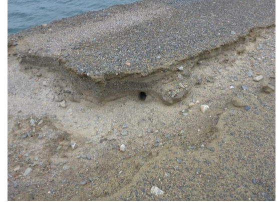
Photo 21: Close up of erosion gully in Dam 4, the burrow from ground animal.
