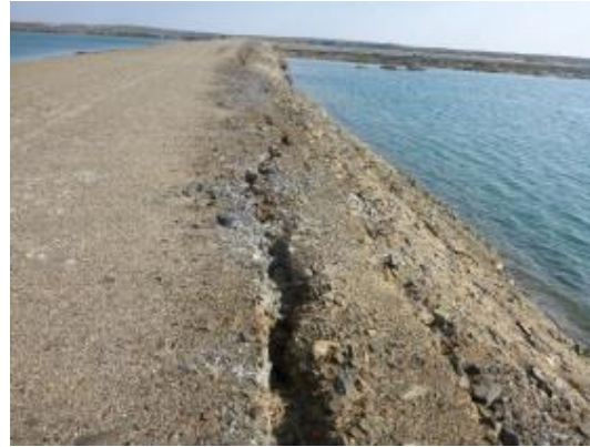
Photo 32: Close up eastern view of Dam M at the new tension cracks observed in 2014, in face of the dam toward Pond 1.
