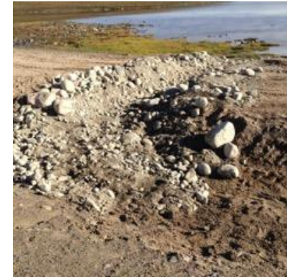
Photo 24: Looking north at the repair work completed over the eroded gully in Dam 3, including geotextile and riprap armoring.
