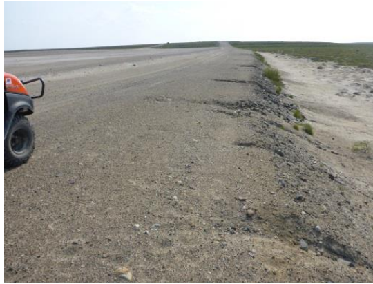
Photo 14: Close up look at one of the large erosion gully in Dam 6.
