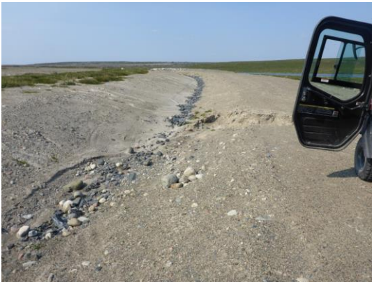
Photo 22: looking northwest at the storm ditch and erosion damage on crest of Dam 3.
