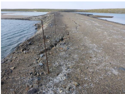
Photo 28: Looking northwest at original tension cracks on Dam M, with Dam N and Pond 2 to the left.
