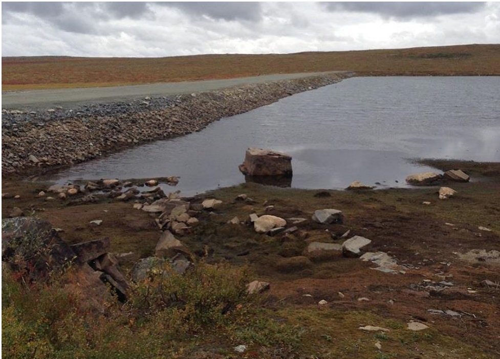
Photo 3: Look south from the Lower Sewage Dam North abutment on the repaired upstream slope and crest. Note the 1.3 meter freeboard available at the time of the photo.
