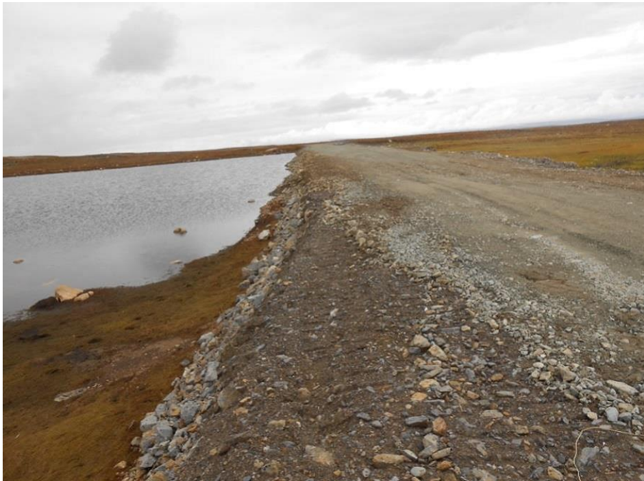
Photo 1: Looking north from the Lower Sewage Dam south abutment on the repaired crest and upstream face.
