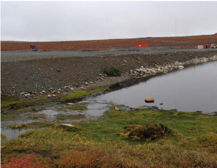
Photo 5: Looking at repaired upstream face and crest of the Upper Sewage Dam. Note the 1.8 meter freeboard available at the time of the photo.
