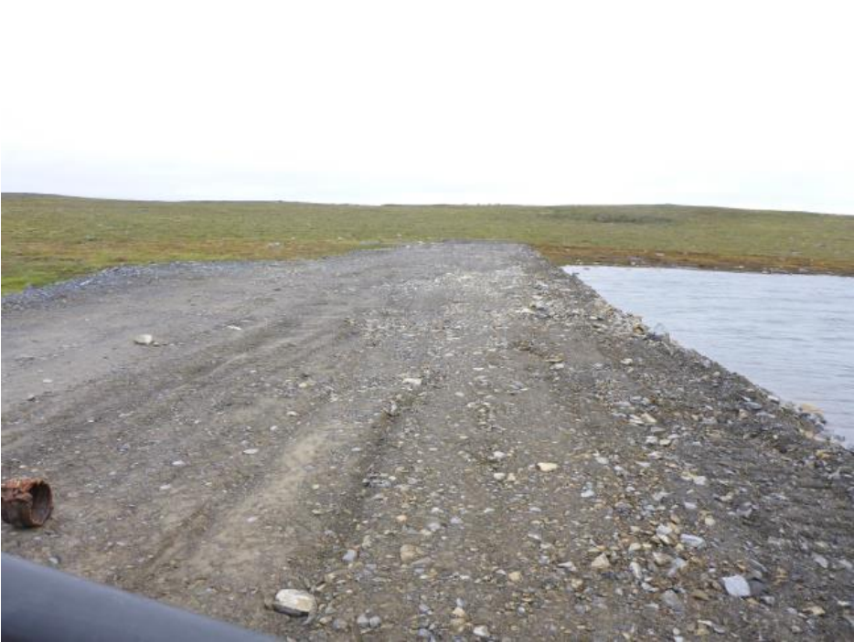
Photo 2: Looking south at the Lower Sewage Dam southern abutment on the additional fill placed to raise the elevation.
