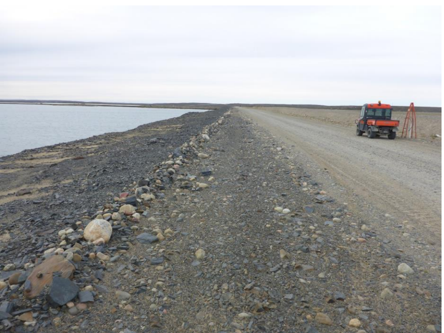
Photo 40: Looking east at the crest from thermistor D3D-1, with the Cell 1 cover to the right and mine rock buttress to the left.
