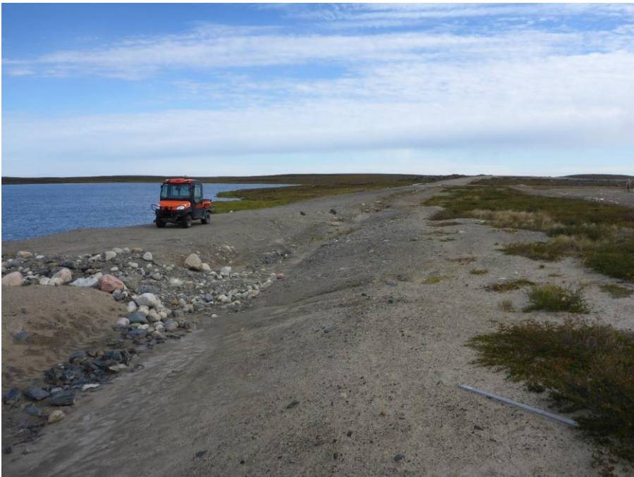
Photo 23: Looking east at the crest and storm drain, with the repaired erosion gully to the left.
