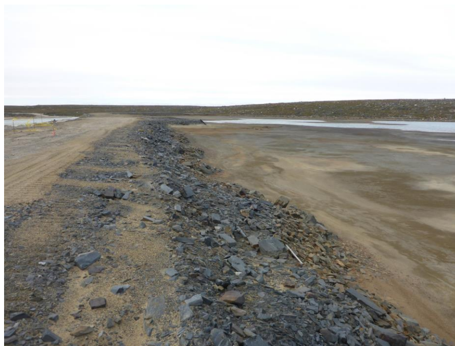
Photo 59: Looking northwest at the upstream slope (facing Cell 5). Note the lowered water level and exposed tailings beach.
