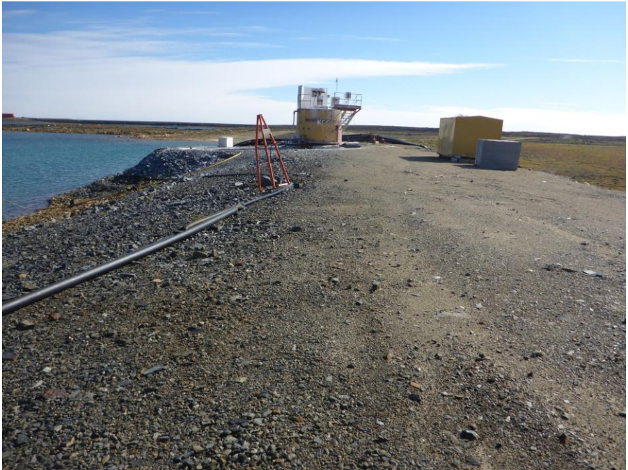
Photo 2: Looking east along the crest. Note the water treatment equipment and work pad extending over the upstream slope
