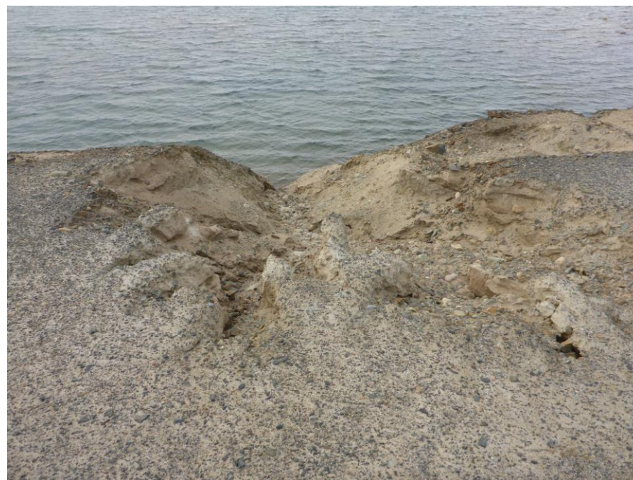
Photo 57: Close up look at an erosion gully over the downstream crest south of the Cell 3 cover boundary.
