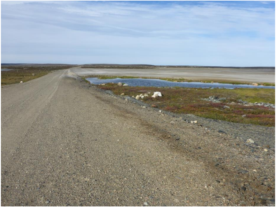
Photo 37: Looking north from the south abutment at the crest with the Cell 3 cover in the background. Note the ponding water near the south abutment.
