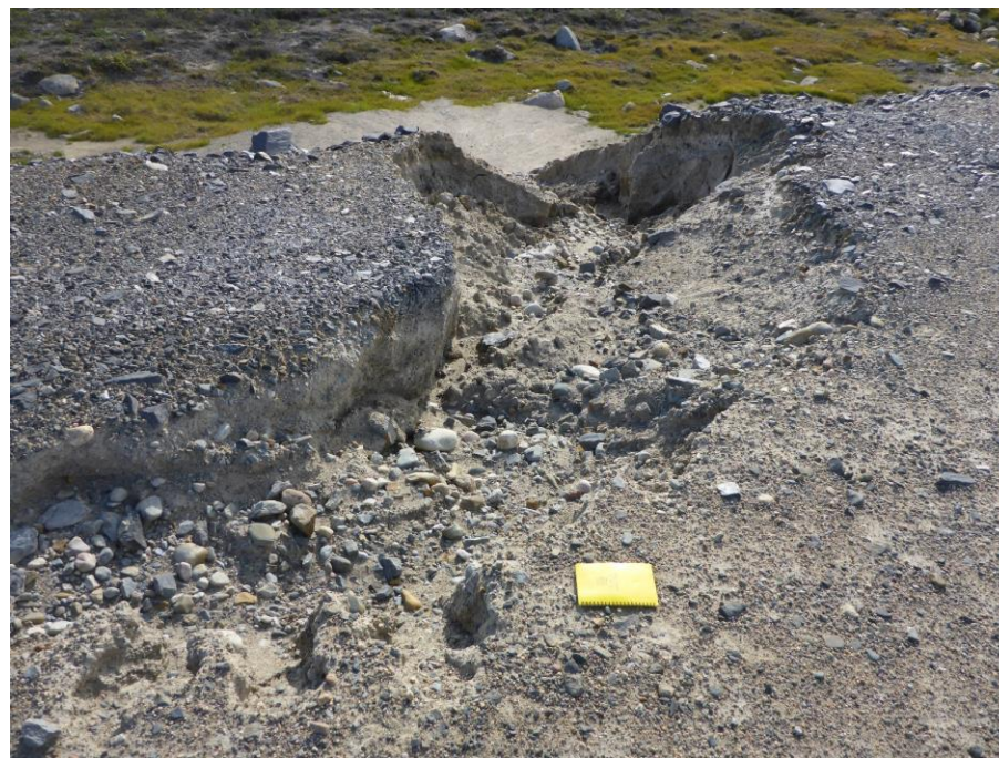
Photo 27: Looking at the erosion gully over the downstream crest at the east abutment
