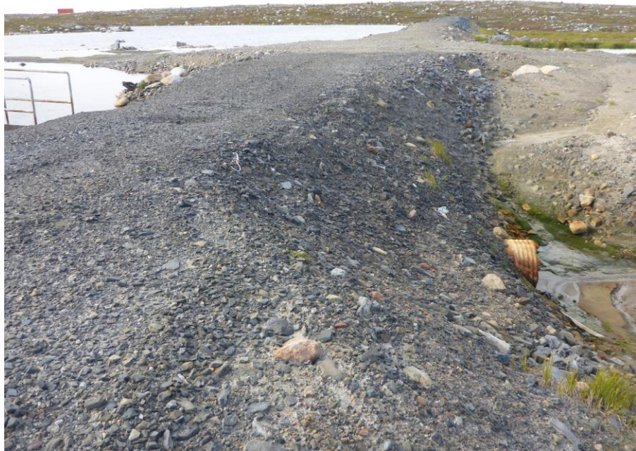
Photo 78: Looking south at the downstream slope of the North Divider Dyke. Note the flow control culvert at the toe of the dyke.
