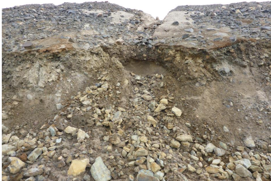
Photo 51: Close up look at an erosion gully over the downstream crest at mid-point of the dam. Note the sloughing at the toe.
