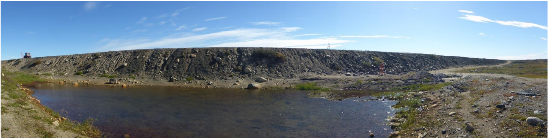
Photo 18: Panoramic view of the downstream slope at the seepage collection pond. Note the erosion gullies.
