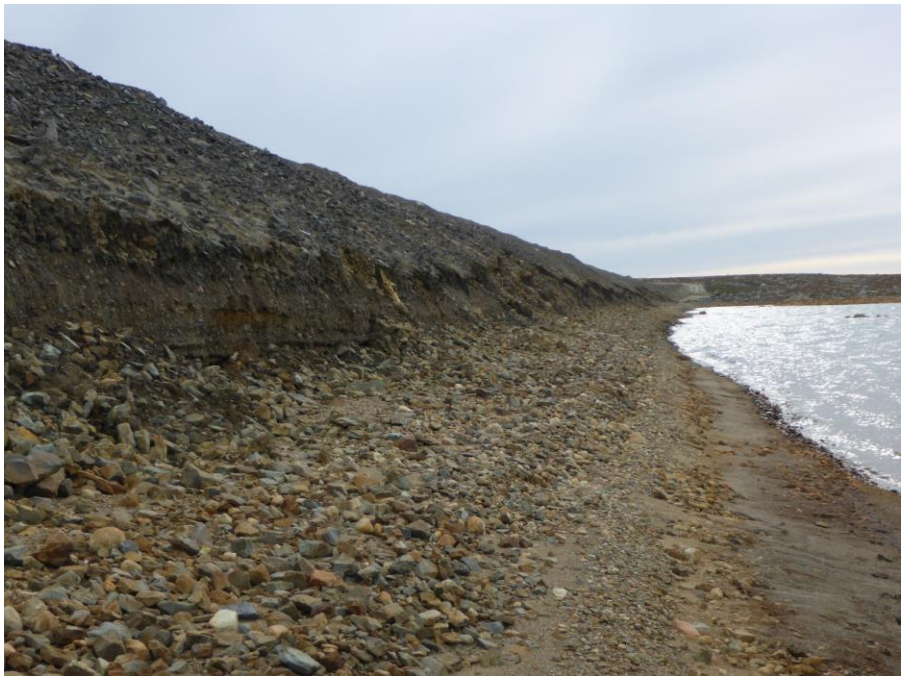
Photo 49: Looking west at the downstream slope from the toe of the dam. Note the near vertical eroded slope.
