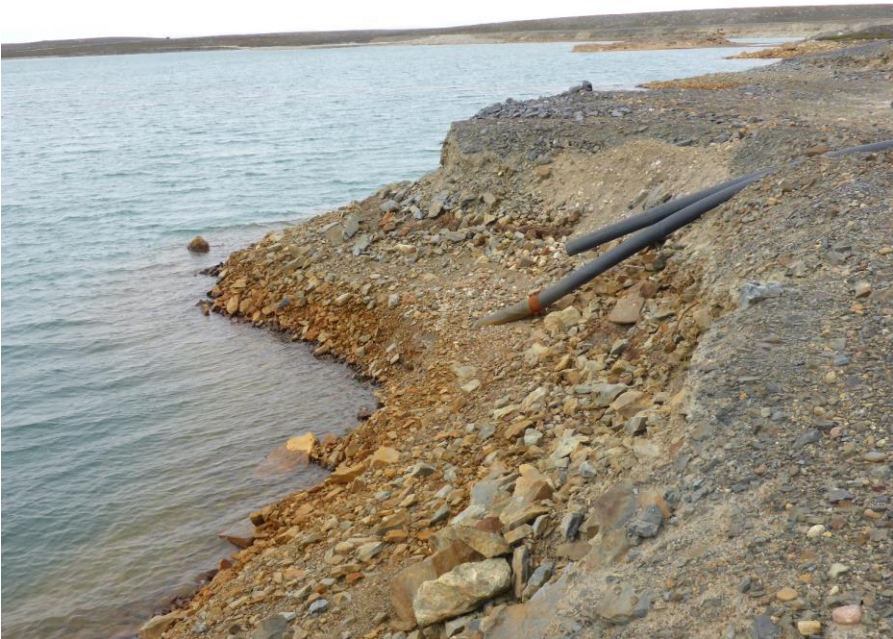
Photo 47: Close up looking north at the downstream slope (facing Pond 2). Note the undercut has caused sloughing and reduce crest width.
