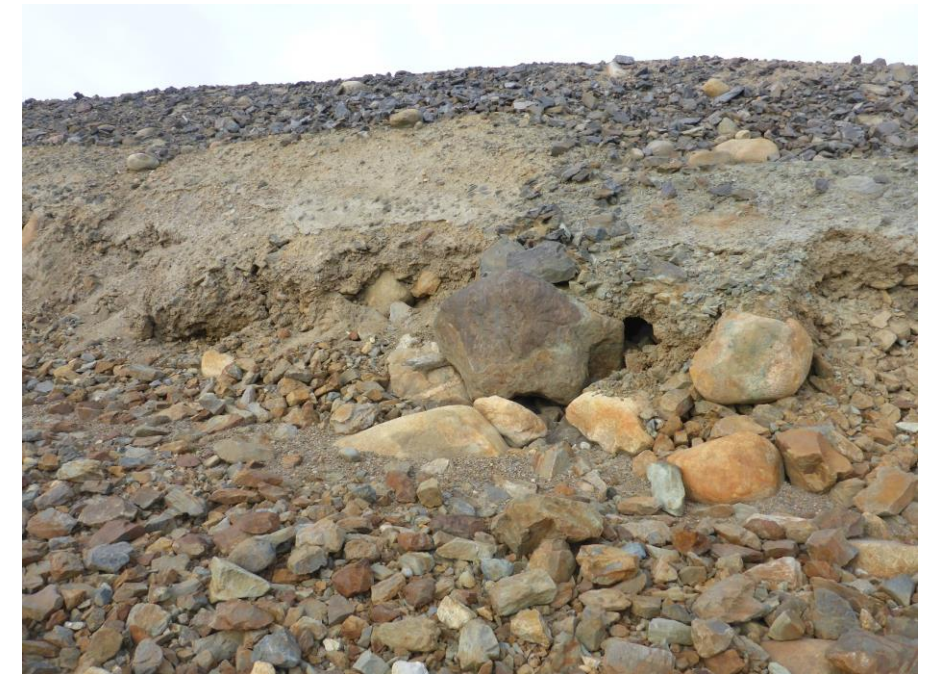
Photo 68: The significant undercut in the downstream slope at 1/3 way down from the Dam J abutment.
