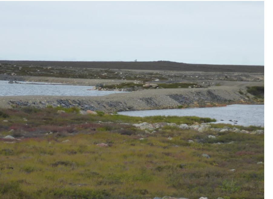
Photo 80: Looking west at the downstream slope of the South Divider Dyke. Note the low spot in the middle of the dyke.
