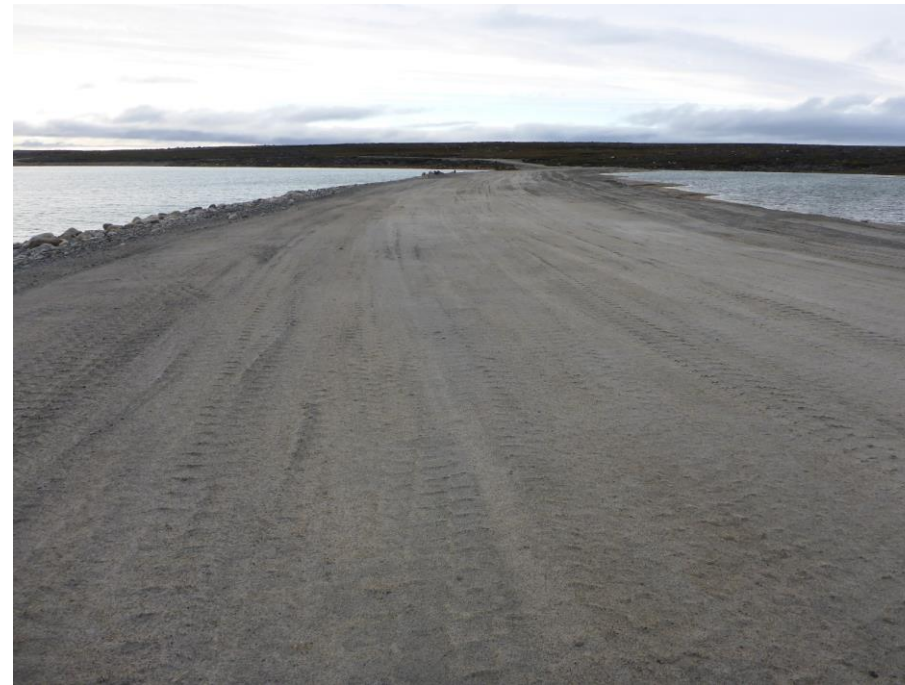
Photo 72: Looking northwest at the crest toward the north abutment. Note the water behind the dam (right) is approximately 0.5m below the crest.
