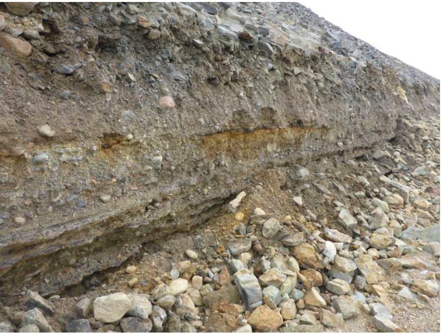
Photo 50: Close up look at the undercut erosion and the near vertical slope.
