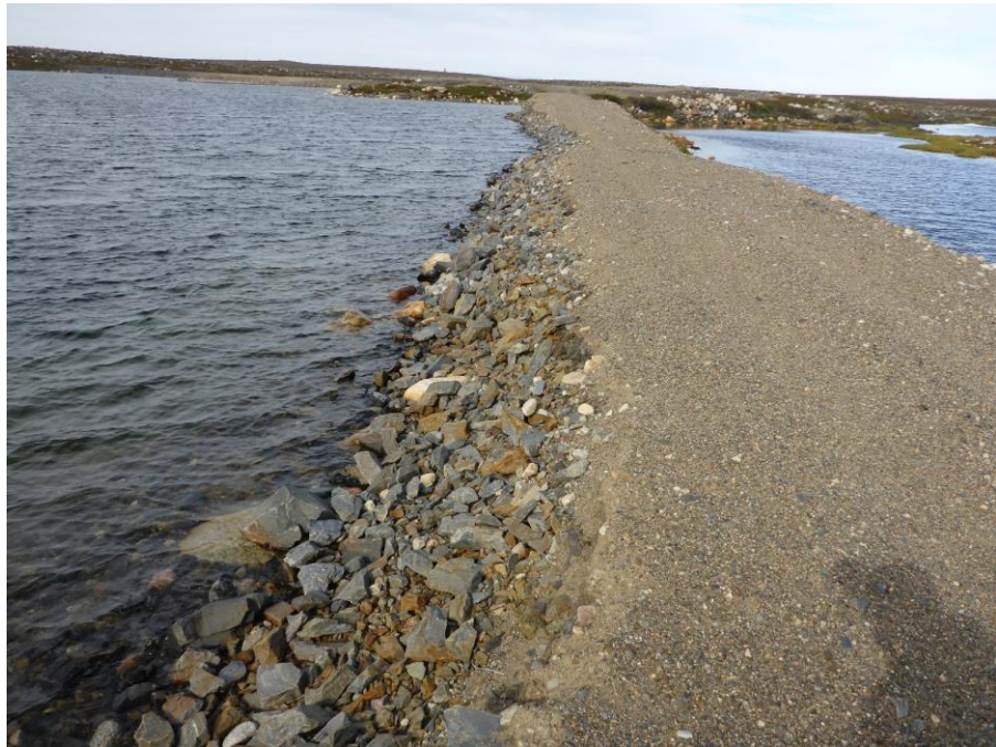
Photo 75: Looking north at the upstream slope of the South Divider Dyke. Note the erosion at the HWM.
