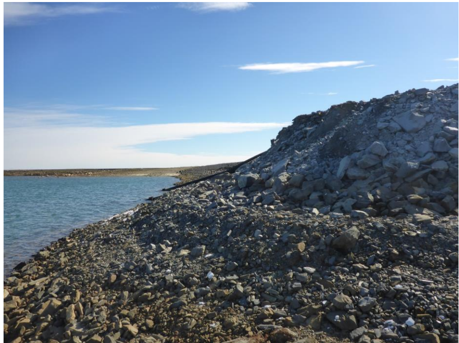
Photo 4: Looking east at the upstream slope at the over steepened work pad extension.
