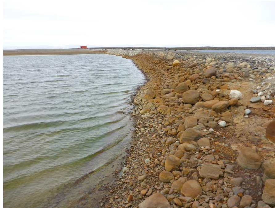
Photo 54: Looking north at the upstream slope (facing Cell 3). Note the erosion at the HWM.
