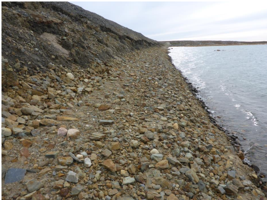
Photo 52: Close up look at the sloughing near the mid-point of the dam from the toe.
