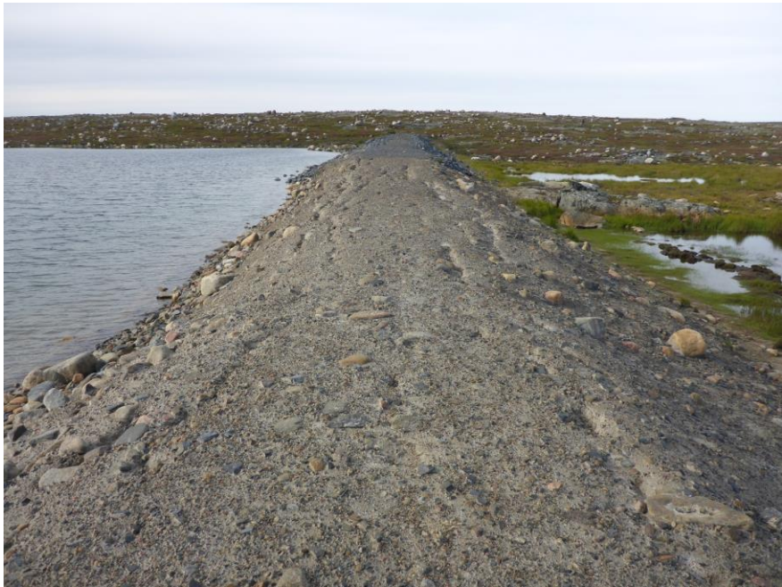
Photo 79: Looking north from value control at the crest of the North Divider Dyke. Note the sloughing, cracks and reduced width of the crest.
