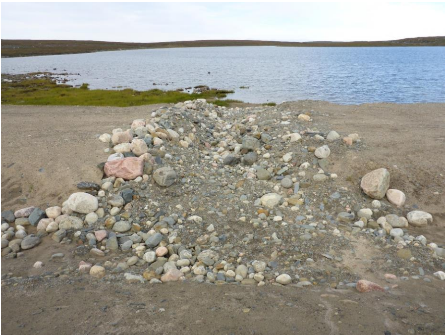
Photo 21: Looking north at the repair erosion gully with boulder armoring. Boomerang Lake is in the background.
