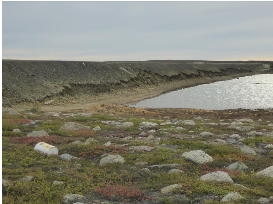
Photo 48: Looking south at the downstream slope (facing Pond 2) from north abutment of Dam J. Note the undercut erosion at the HWM.
