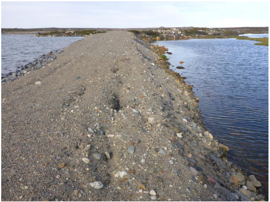
Photo 76: Looking north at the downstream slope of the South Divider Dyke. Note the sloughing and cracks.
