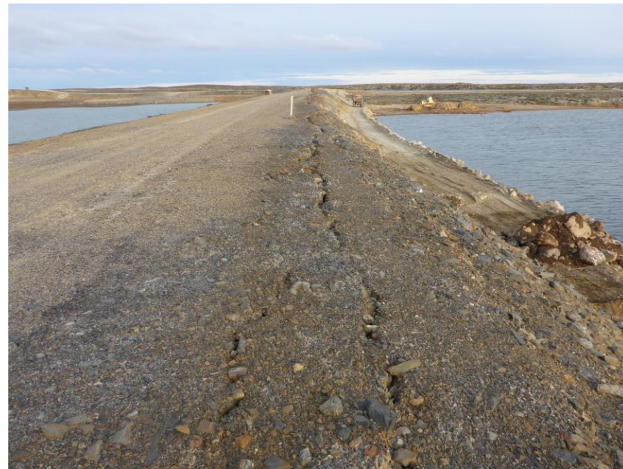
Photo 70: Looking southeast at cracks along the downstream crest near Dam J abutment, above the eastern buttress.
