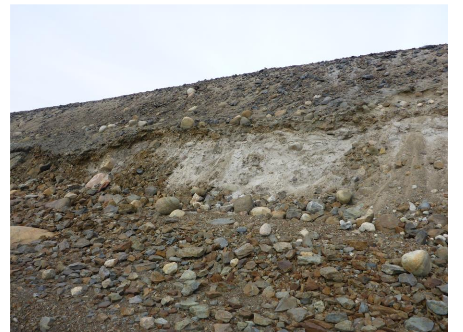
Photo 63: Looking at the undercut and sloughed downstream toe near the mid-point of the dam. Note the exposed loose poorly graded fine sand foundation.
