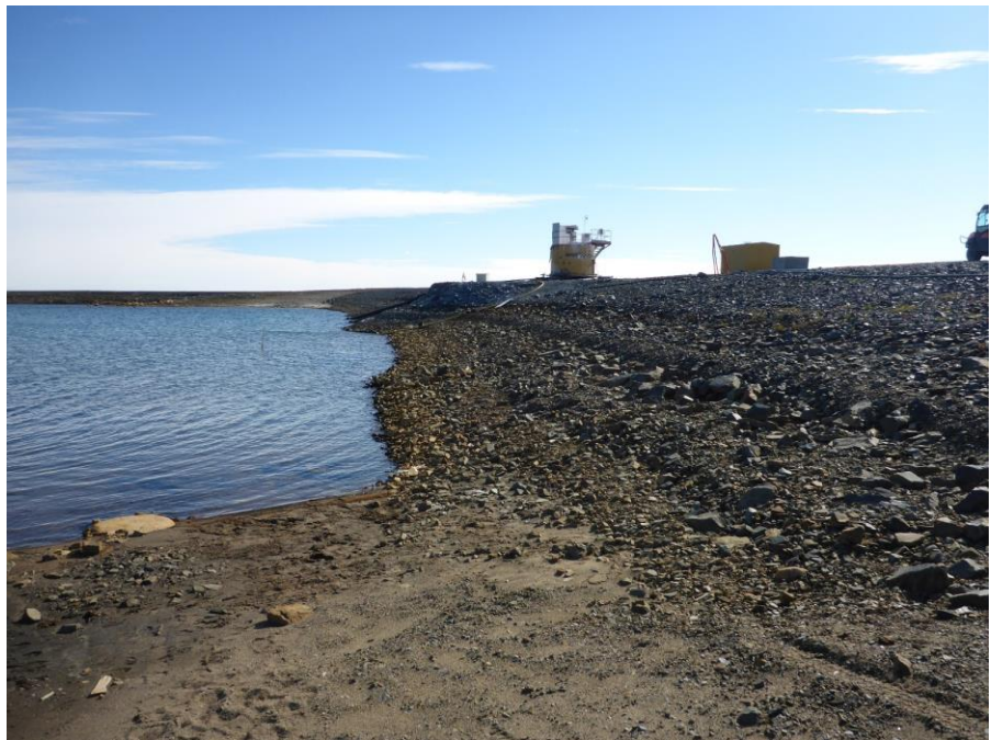
Photo 1: Looking east along the upstream slope. Note the erosion at the HWM.
