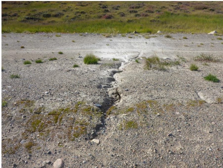
Photo 13: Looking at the erosion gully about 1/3 way past the north abutment.
