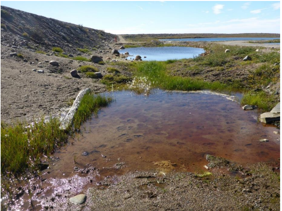
Photo 16: Looking south at the seepage collection pond at northern buttress.
