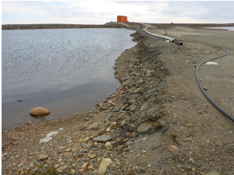
Photo 43: Looking south at the upstream slope (facing Pond 1). Note the erosion at the HWM.
