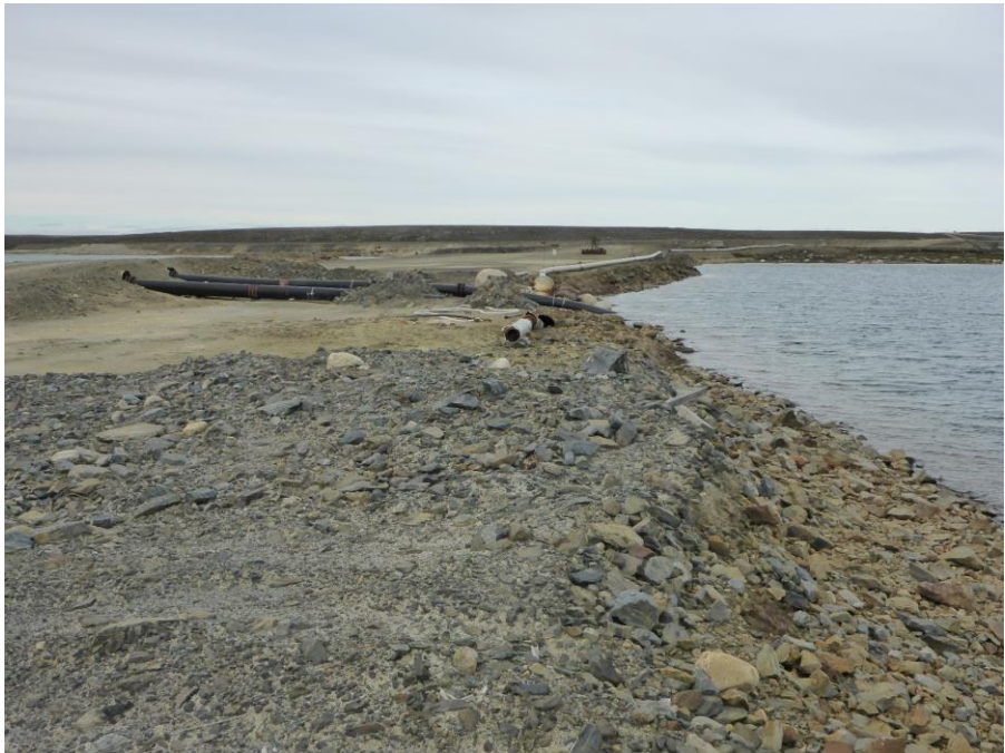
Photo 44: Looking north at the upstream slope (facing Pond 1). Note the erosion at the HWM.
