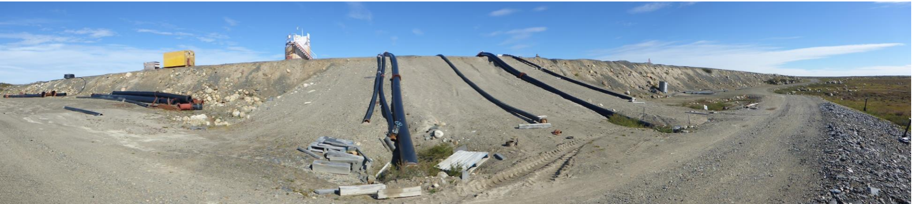
Photo 5: Panoramic view of the downstream slope at the siphon. Note the erosion gullies.
