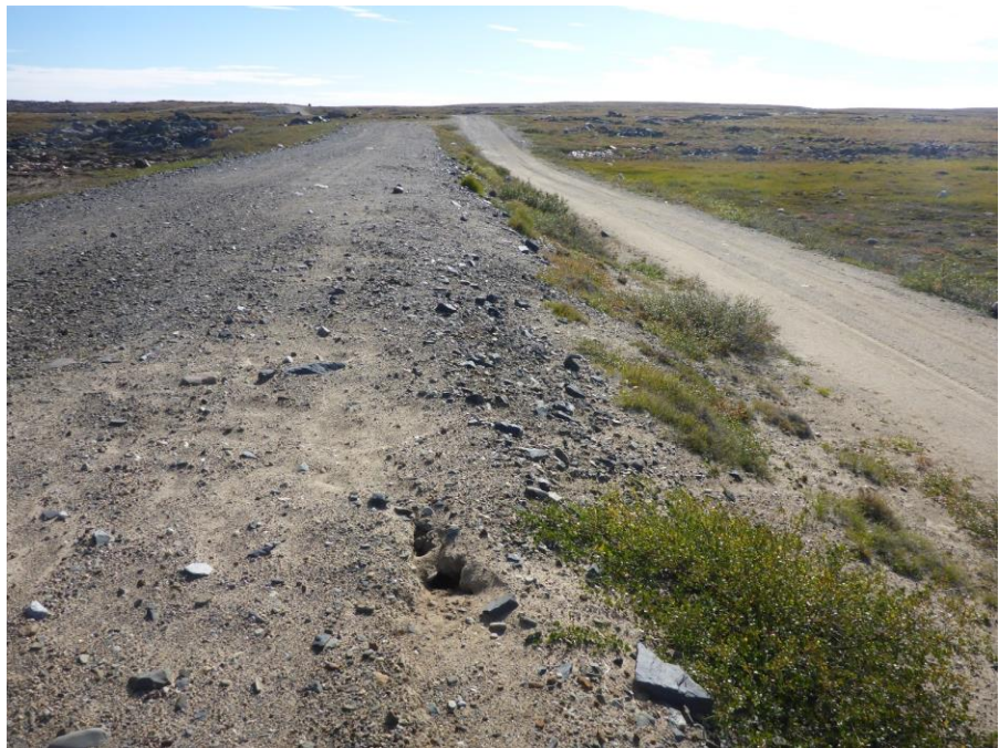
Photo 9: Looking south at the mid-point of the dam at the downstream crest. Note the animal burrow.
