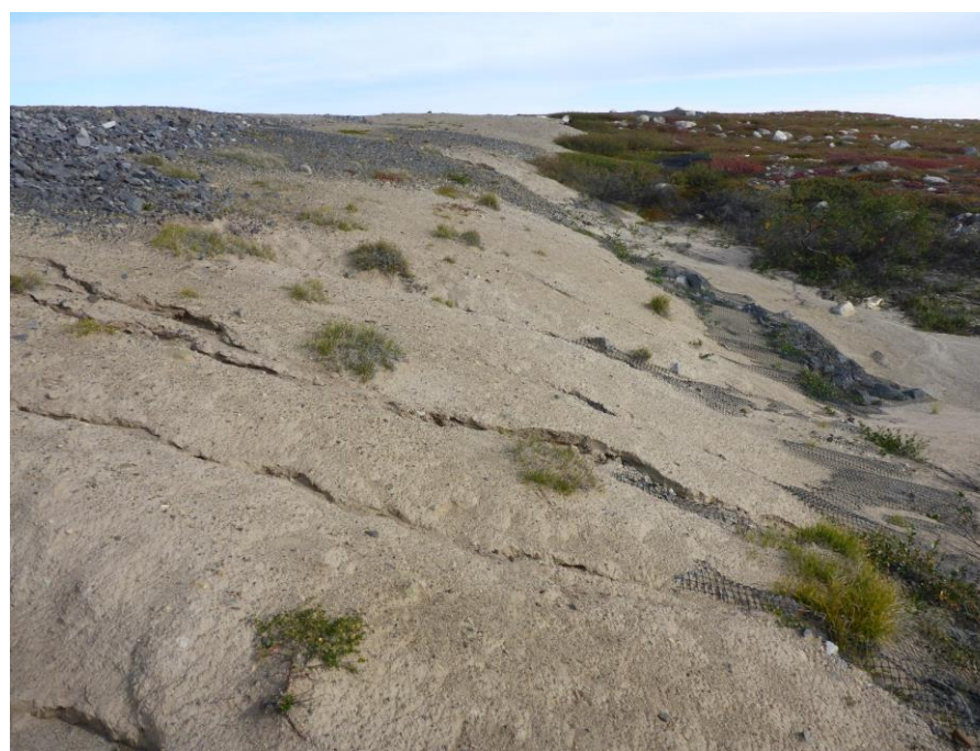
Photo 28: Looking east at the downstream slope at the east abutment. Note the erosion gullies and exposed geogrid.
