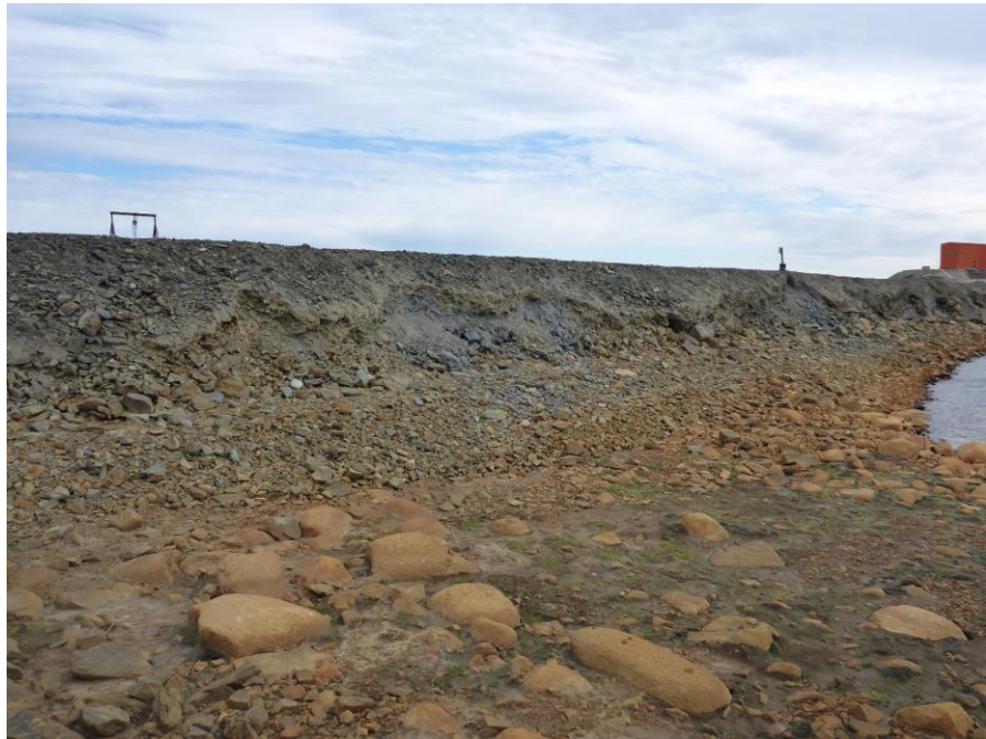
Photo 46: Looking south at the downstream slope (facing Pond 2). Note the undercut and erosion at the HWM.
