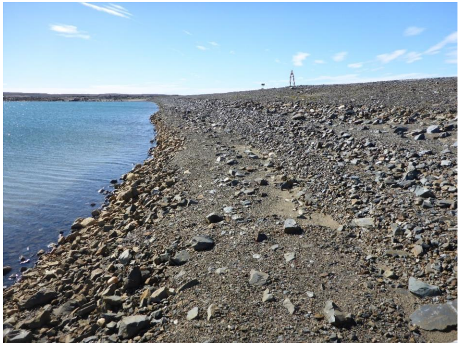
Photo 14: Looking south along the upstream slope. Note the erosion at the HWM.
