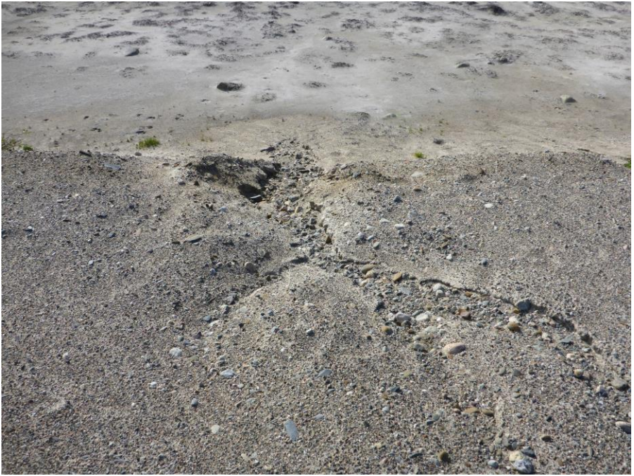
Photo 36: Looking south at the erosion gully over the downstream crest at the mid-point of the dam.
