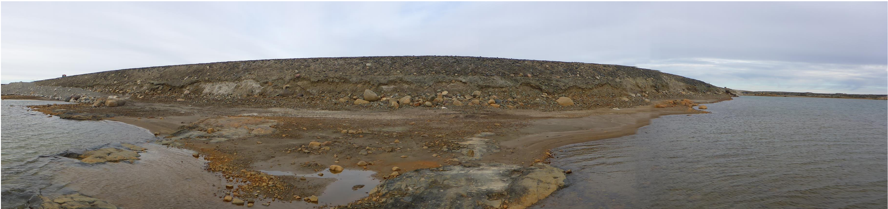
Photo 64: Panoramic view of the downstream slope from the mid-point of the dam. Note the undercut erosion and sloughing material. The loose fine sand foundation can be seen beyond the western buttress at the left.
