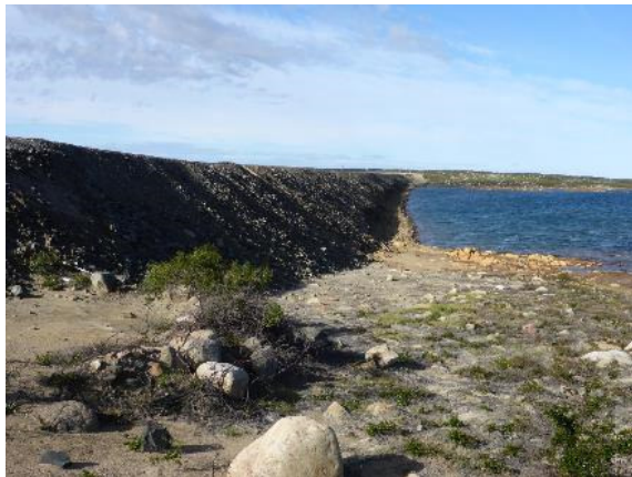
Photo 30: Looking south at the Dam K downstream slope (facing Pond 2) from north abutment of Dam J. Note the undercut erosion at the HWM.
