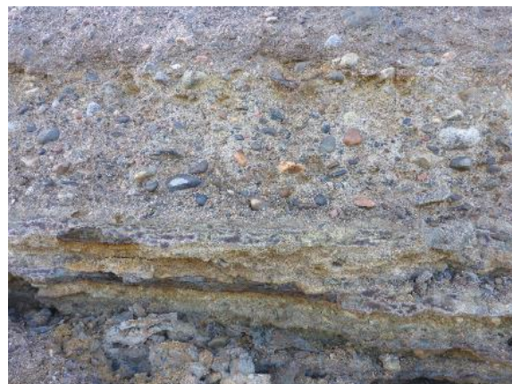
Photo 31: Close up look at the Dam K undercut erosion and the near vertical slope.
