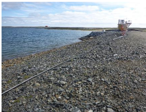
Photo 2: Looking east along the Dam 1A crest. Note the water treatment equipment and work pad extending over the upstream slope
