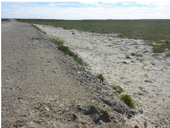
Photo 24: Looking south from the Dam 6 north abutment at the crest and downstream toe. Note the erosion at the bottom of the photo.
