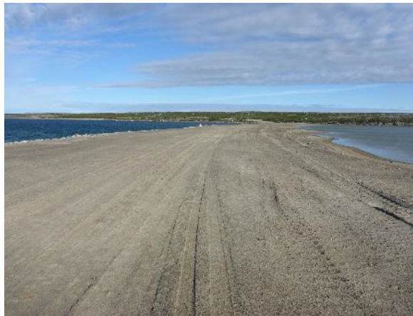
Photo 40: Looking northwest at the Dam N crest toward the north abutment. Note the water behind the dam (right) is approximately 0.8m below the crest.
