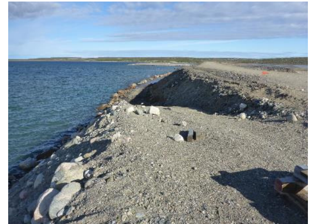
Photo 38: Looking west at the repair buttress at Dam M with armor at the toe.
