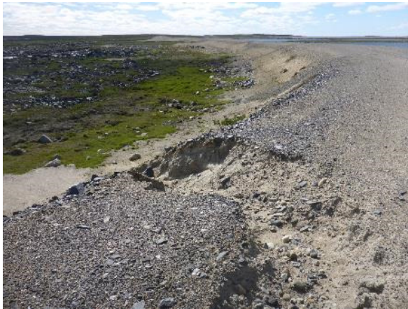
Photo 21: Looking at the erosion gully over the downstream crest at the east abutment
