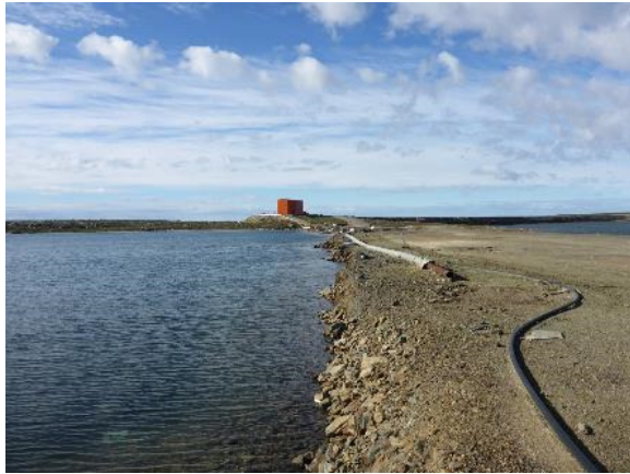
Photo 27: Looking south at the Dam J upstream slope (facing Pond 1). Note the erosion at the HWM.
