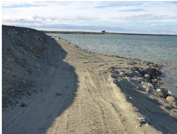
Photo 37: Close up look toward the east at the repair buttress at Dam M with armor at the toe.
