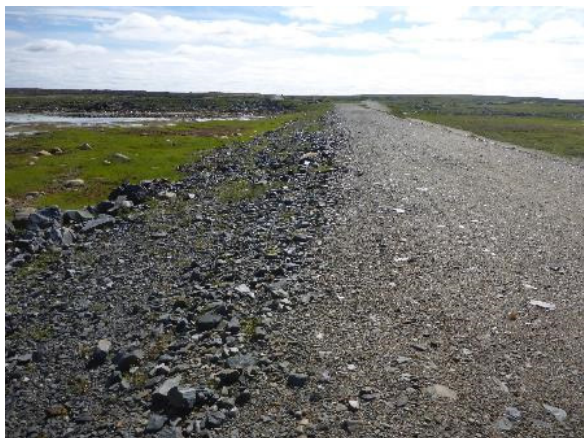
Photo 4: Looking south along the Dam 1B upstream slope. Note there is no adjacent water.
