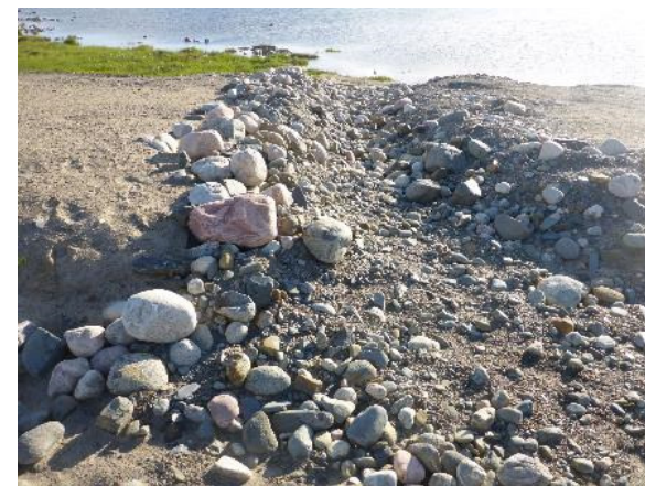
Photo 14: Looking north at the Dam 3 drainage with boulder armoring. Boomerang Lake is in the background.
