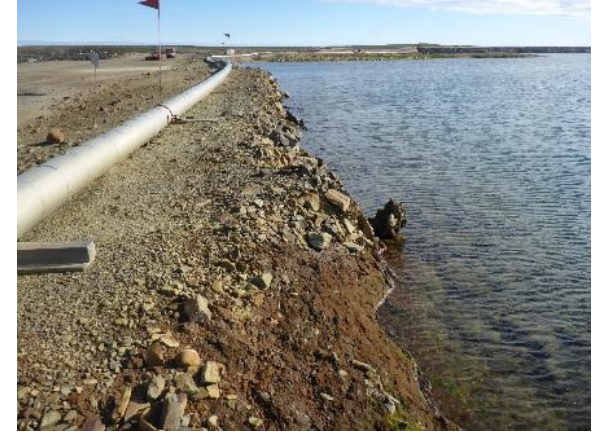
Photo 29: Close up looking north at the Dam J downstream slope (facing Pond 1). Note the undercut has caused sloughing and reduce crest width.
