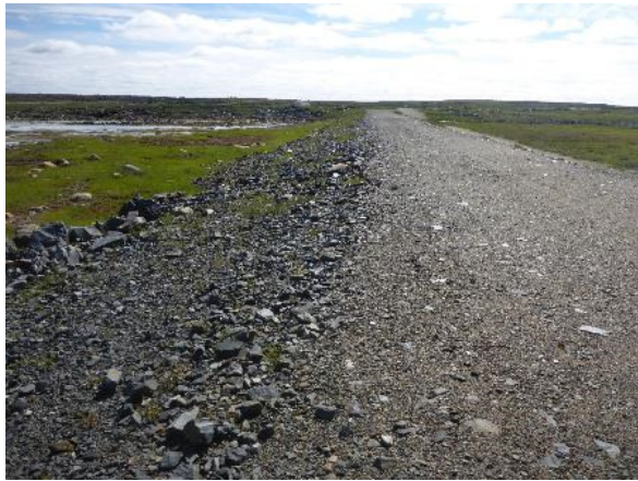
Photo 6: Looking south along the Dam 1C upstream slope. Note there is no adjacent water.
