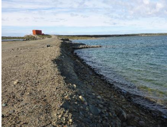
Photo 28: Looking north at the Dam J upstream slope (facing Pond 1). Note the erosion at the HWM.
