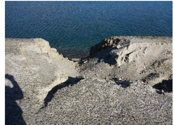
Photo 32: Close up look at the Dam K undercut erosion and the near vertical slope.
