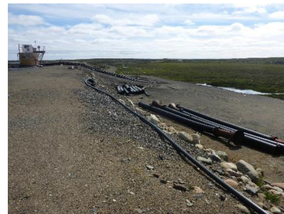
Photo 3: Looking east along the Dam 1A downstream slope. Note discharge siphons.
