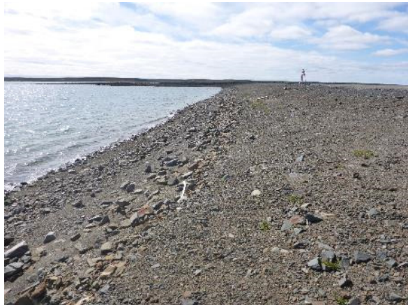
Photo 9: Looking south along the Dam 2 upstream slope. Note the erosion at the HWM.
