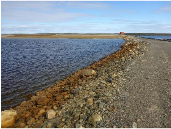
Photo 33: Looking north at the Dam L upstream slope (facing Cell 3) and the crest from the south abutment. Note the Cell 3 cover in the left horizon.
