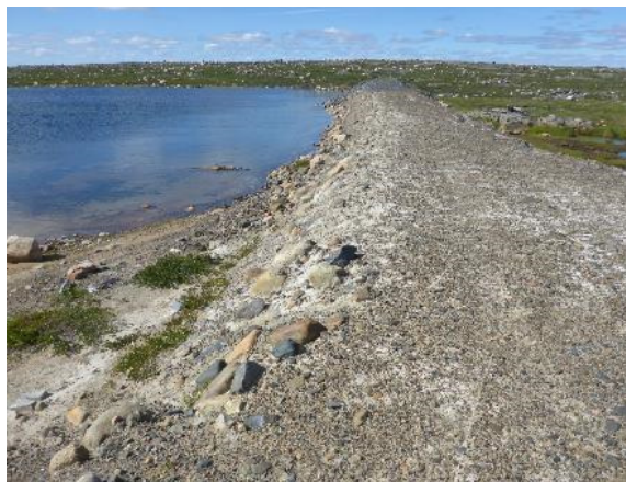
Photo 43: Looking north at the northern portion of the Divider Dyke. Note the reduced crest width and sloughing and cracks.
