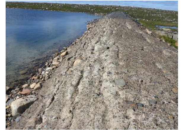
Photo 44: Close up look of the sloughing and cracks on the northern section of the Divider Dyke.
