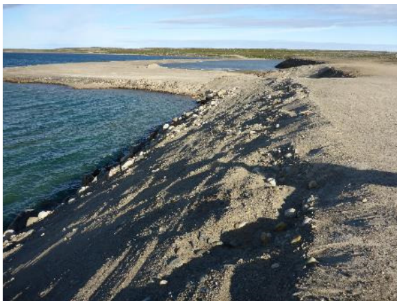
Photo 36: Looking west at the Dam M repaired buttress and armor at the toe, with Dam N and Pond 2 to the left.
