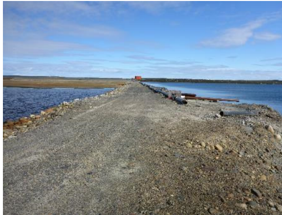
Photo 34: Looking north along the Dam L centerline. Note the reduction in crest width near the end.
