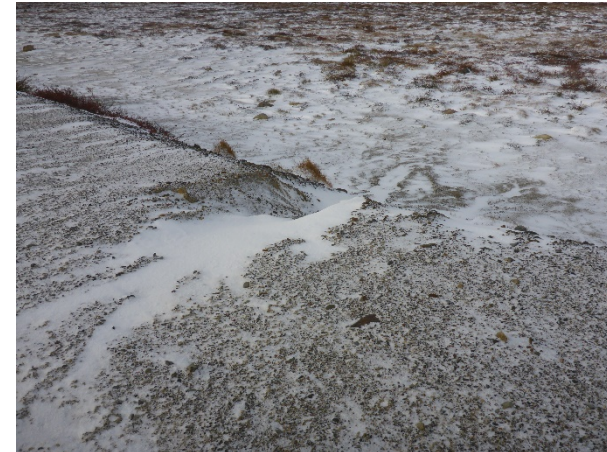
Photo 22: Looking southwest at one of the erosion gullies at the downstream crest of Dam 5.
