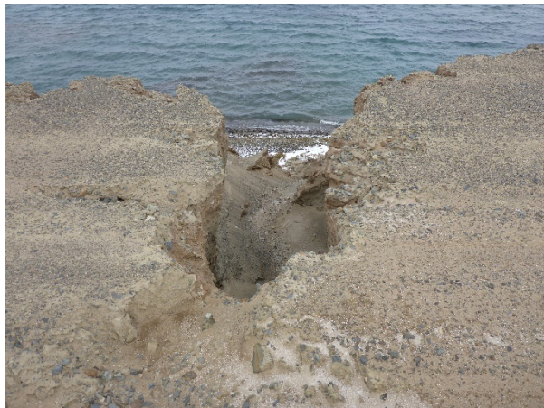
Photo 33: Looking northwest at another one of the five erosion gullies along the upstream crest of Dam K
