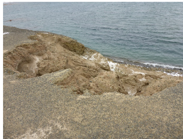
Photo 31: Looking northwest at one of the five erosion gullies along the upstream crest of Dam K
