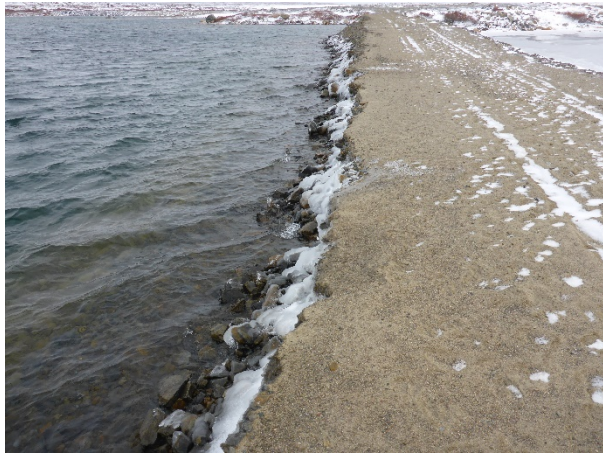
Photo 47: Looking north at the repaired upstream slope and crest of the southern divider dyke.
