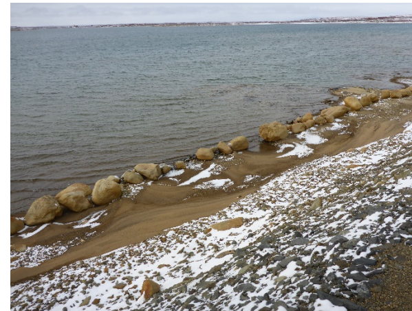
Photo 43: Looking southwest at the riprap armor at the toe of reinforcement buttress.
