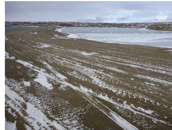
Photo 46: Looking north at the crest of Dam N and ponding water with less than 1m freeboard.
