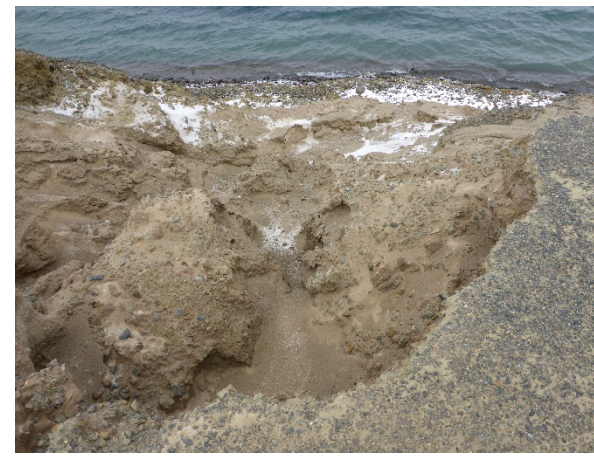
Photo 32: Looking northwest, down toward the toe at one of the five erosion gullies along the upstream crest of Dam K
