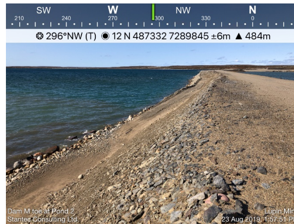
Photo 45: Looking west at the reinforcement buttress of Dam M.
