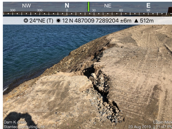
Photo 35: Looking north down toward the toe at one repaired but sloughed gullies along the downstream crest of Dam K
