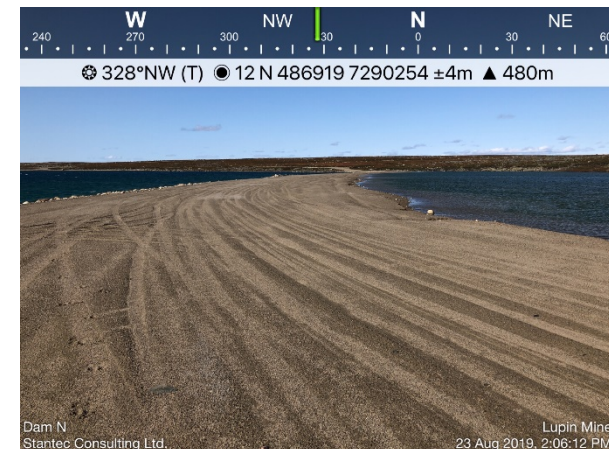
Photo 49: Looking north at the crest of Dam N and ponding water with less than 1m freeboard.
