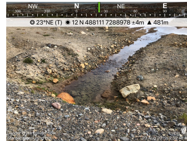
Photo 52: Looking north at the culvert discharge at the malfunctioning gate valve.
