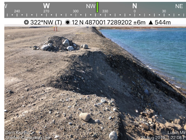
Photo 36: Looking north down toward the toe at one repaired but sloughed gullies along the downstream crest of Dam K
