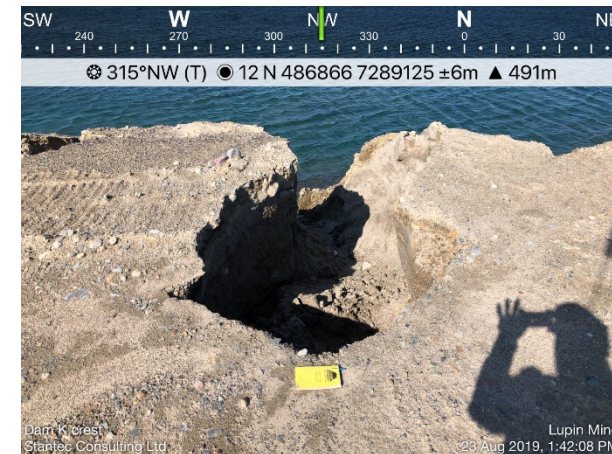
Photo 37: Looking northwest down toward the toe at one repaired but sloughed gullies along the downstream crest of Dam K
