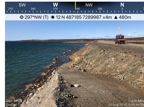
Photo 6 Looking west at the sloughed and submerged toe of reinforcement buttress.
