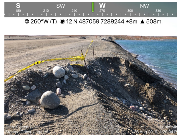
Photo 33: Looking west at one of the repaired but sloughed gullies along the downstream crest of Dam K
