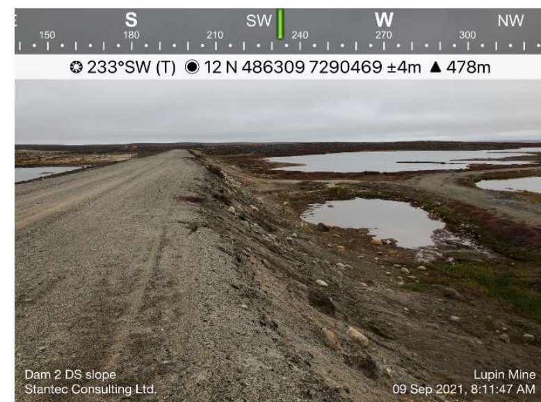
Photo 11: Looking southwest at the downstream slope of Dam 2 with the seepage collection pond.
