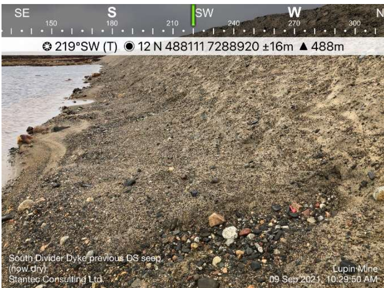
Photo 52: Looking southwest at one of the old seepage zones at the toe and no seepage is observed.
