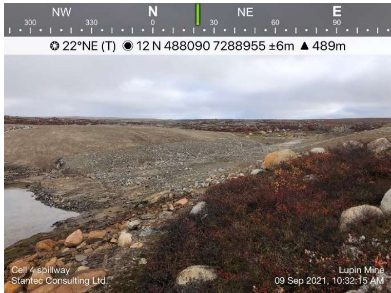
Photo 53: the newly constructed Cell 4 spillway through the Divider Dyke.
