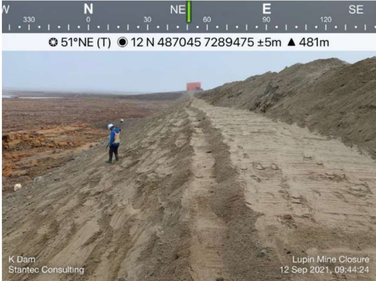
Photo 34: Looking northeast at the reslope with thin layered compaction being carried out by the excavator.
