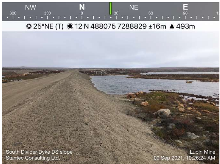
Photo 51: Looking northeast at the downstream slope and the old seepage zones at the toe of the divider dyke. No seepage was observed.
