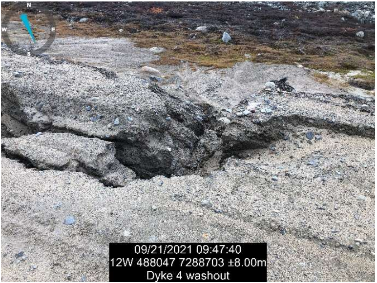
Photo 18: View of the erosion at the D/S crest of Dam 4 near the east abutment
