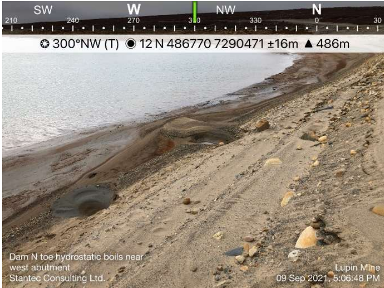
Photo 49: The tailings boils observed near the north abutment of Dam N
