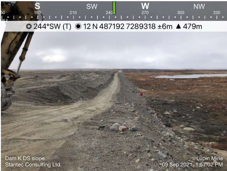
Photo 32: Looking southwest on the ongoing resloping work over the compacted buttress.
