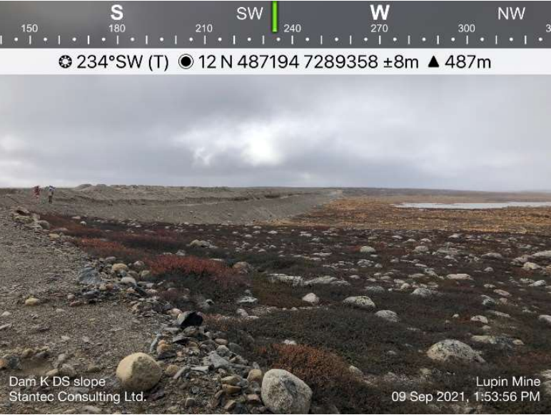
Photo 31: Looking southwest at the resloping being constructed over the buttress at Dam K.
