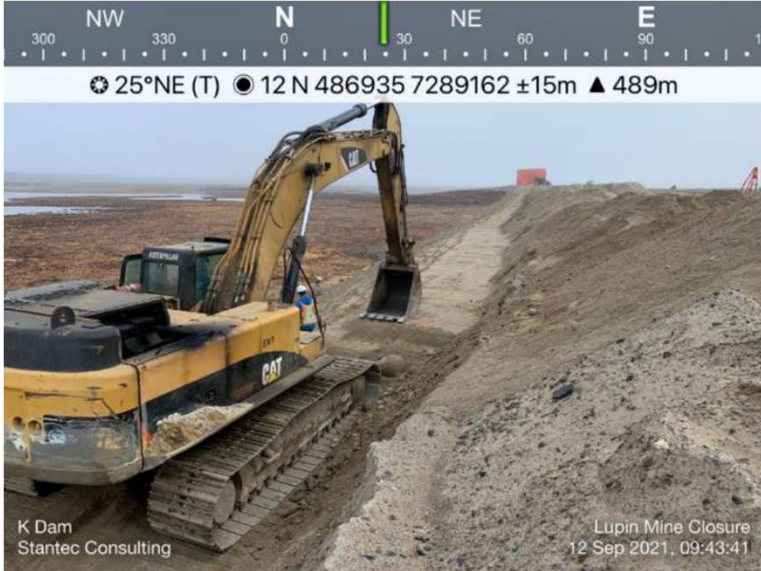
Photo 35: Looking northeast at the reslope with thin layered compaction being carried out by the excavator.
