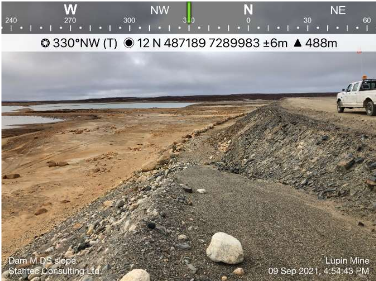
Photo 45: Looking northwest at the reinforcement buttress of Dam M at the toe of the dam.
