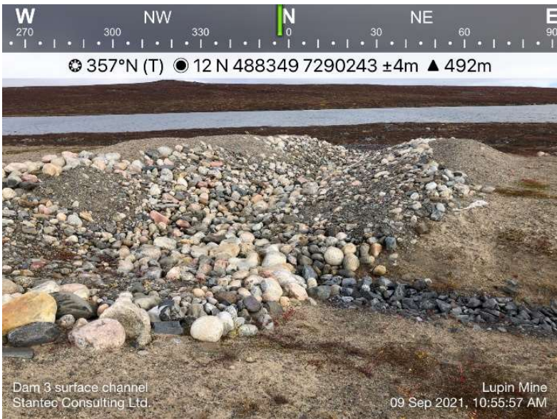
Photo 15: Looking north at the surface ditch spillway on Dam 3.
