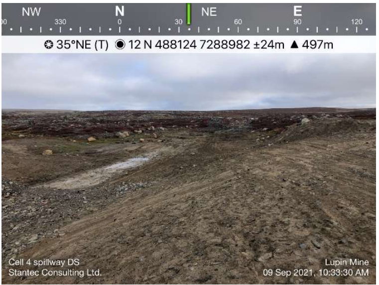
Photo 55: the outlet of Cell 4 spillway through the Divider Dyke into the Chain Lake area.
