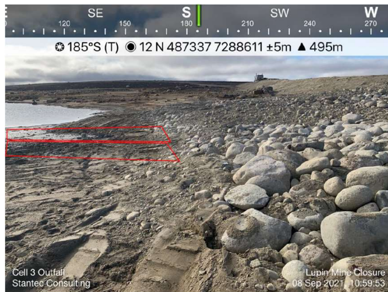
Photo 41: Cell 3 outlet that need to be field extended for transition into the shoreline.
