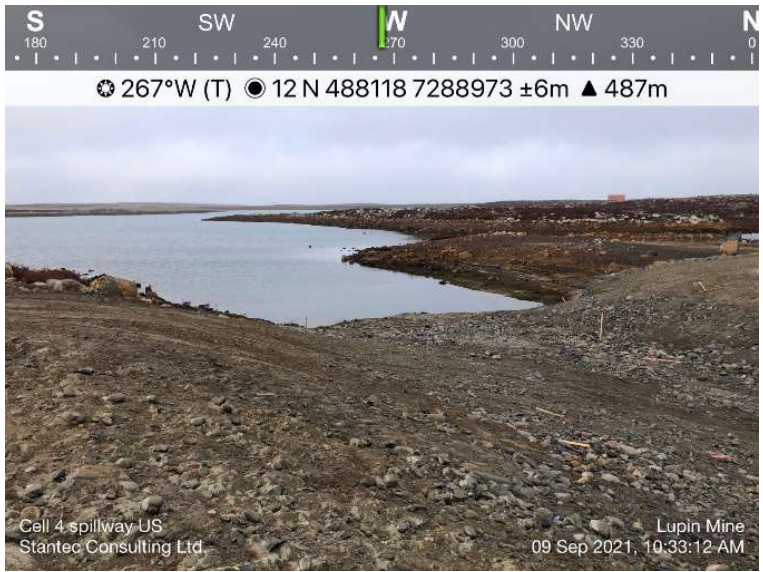
Photo 54: the inlet of Cell 4 spillway through the Divider Dyke.
