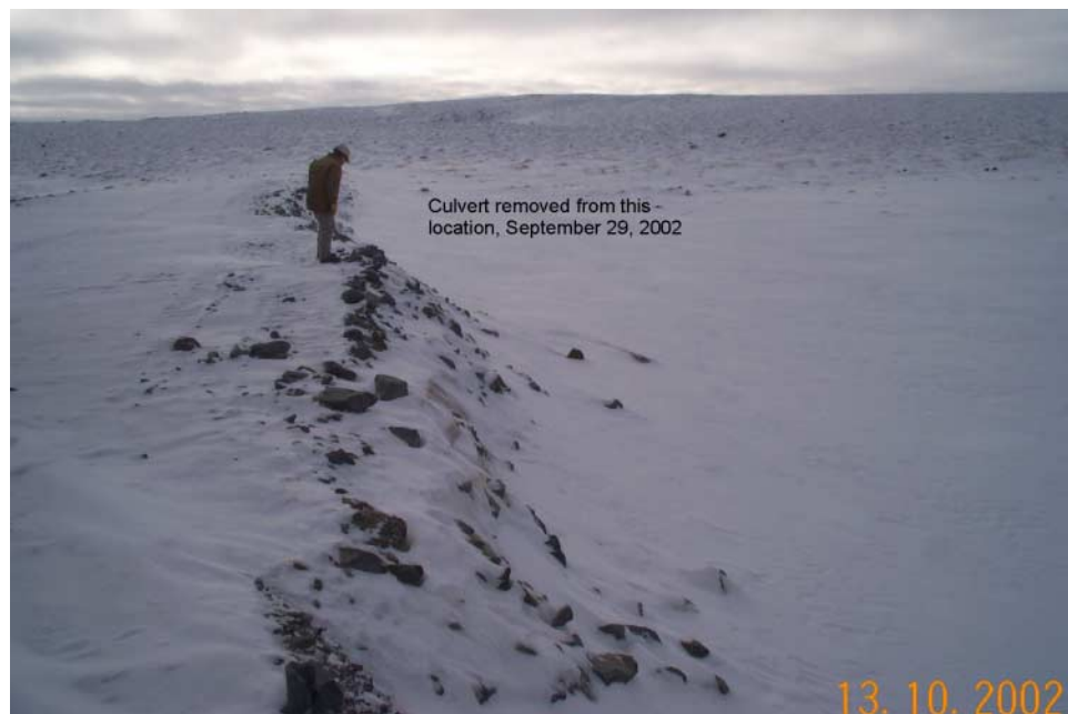
Photo 1 - Sewage Lake No.2 upstream embankment showing culvert removed.
