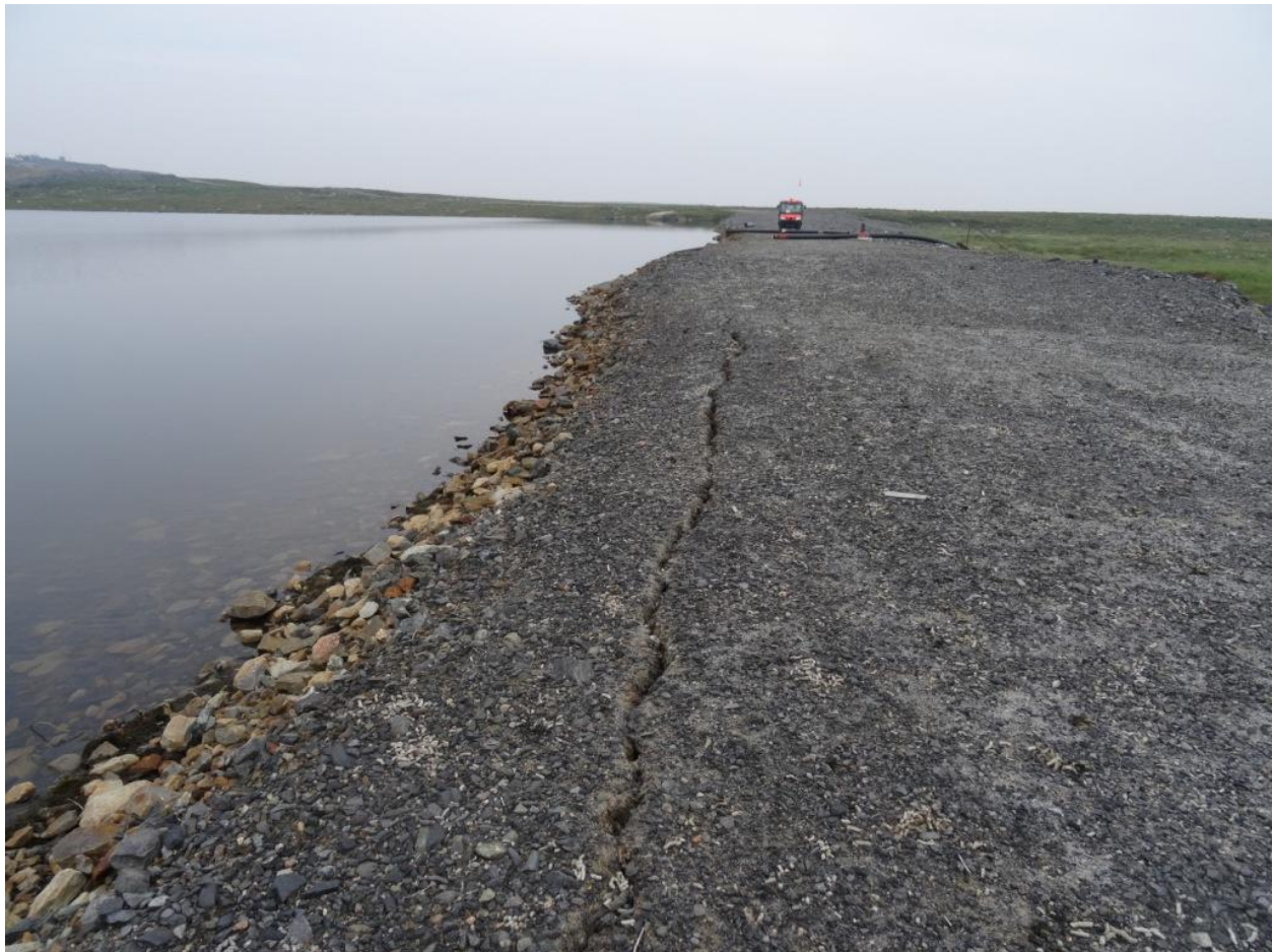
Figure 3. Crack in the dam at LSL.
