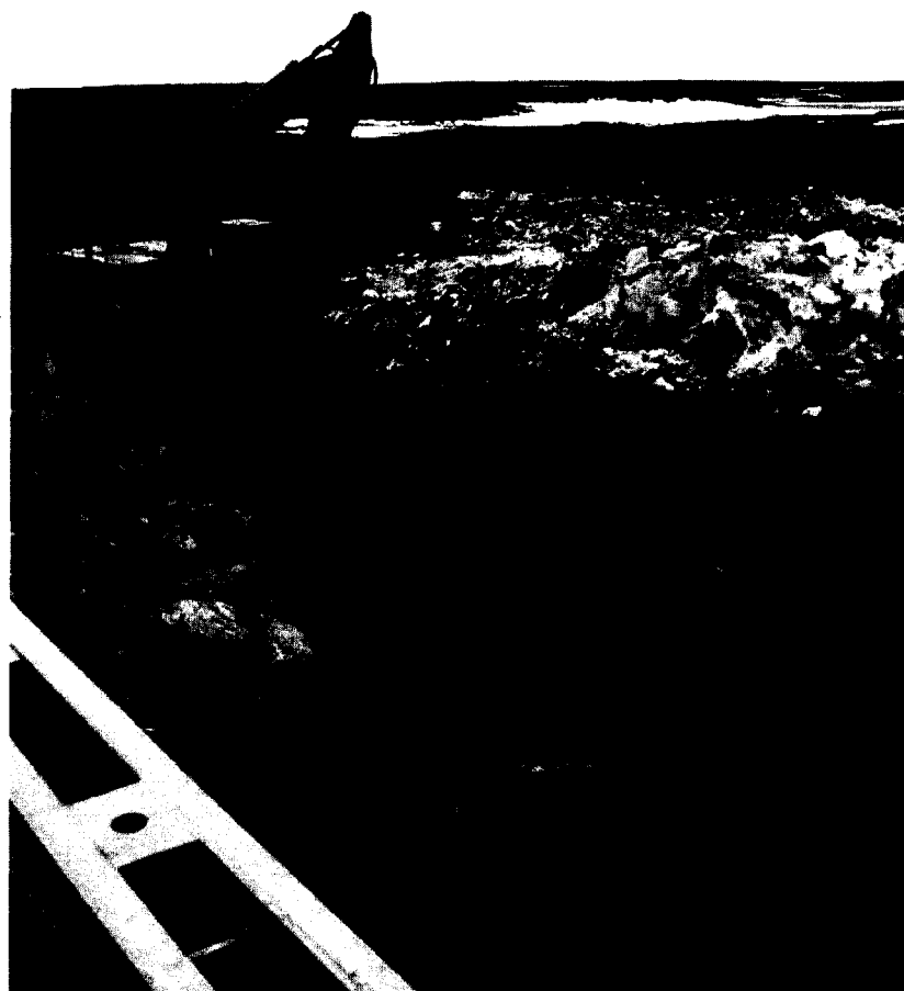
Photo 9. R02 – Adding boulders to stabilize unstable bank area (U/S S side) (17Jun07)
