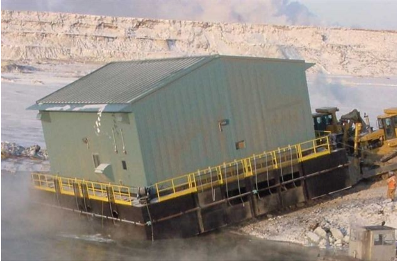
Barge being moved into the water – Intake screen location is visible on the end of the hull
