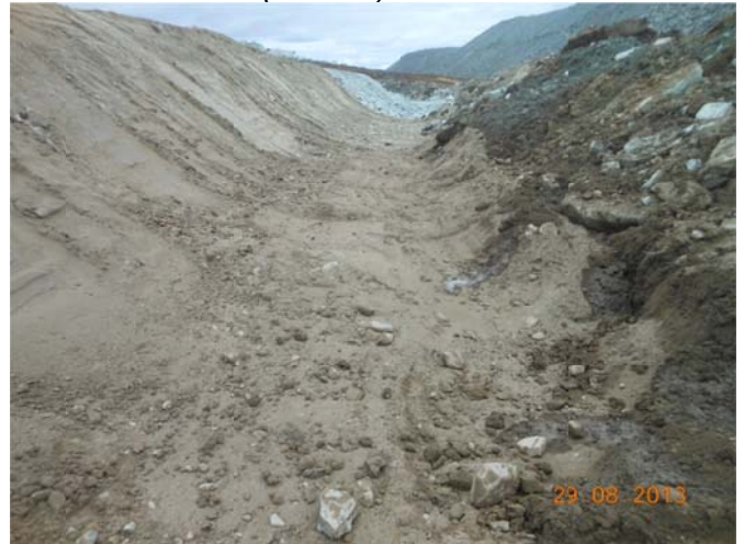
Figure 5: final till placement over an entire section after 1 day of work. The till is flattened and compacted before any rockfill placement.
