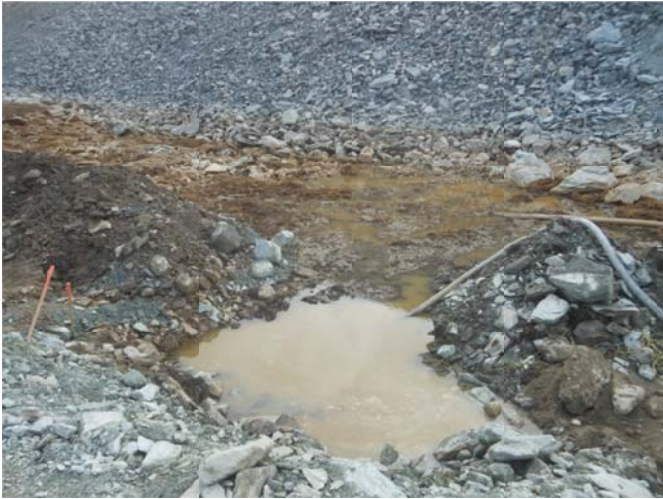
Figure 7: water accumulation along the side of the road before works begin. View of the eastern channel.
