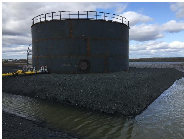
Photo 48: Whale Tail Pit Fuel Tank Farm Facility
