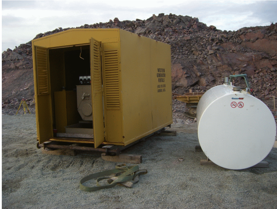
Photo 3: Diesel generator inside shack, fuel tank to the right.
