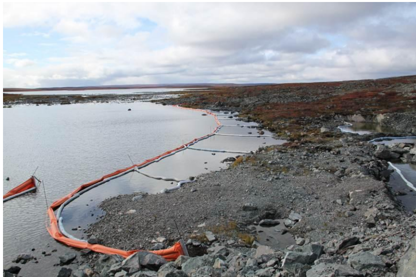
Photo 17: Booms and screens in place at HADD bridge to prevent any fuel from entering stream
