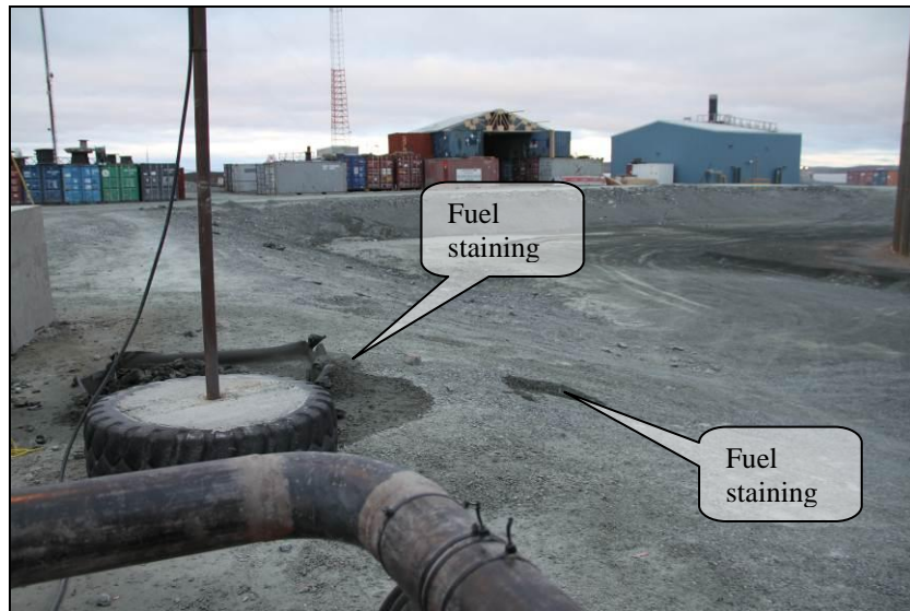
Photo 26: Staining observed at the Meadowbank on-site fuel tank farm
