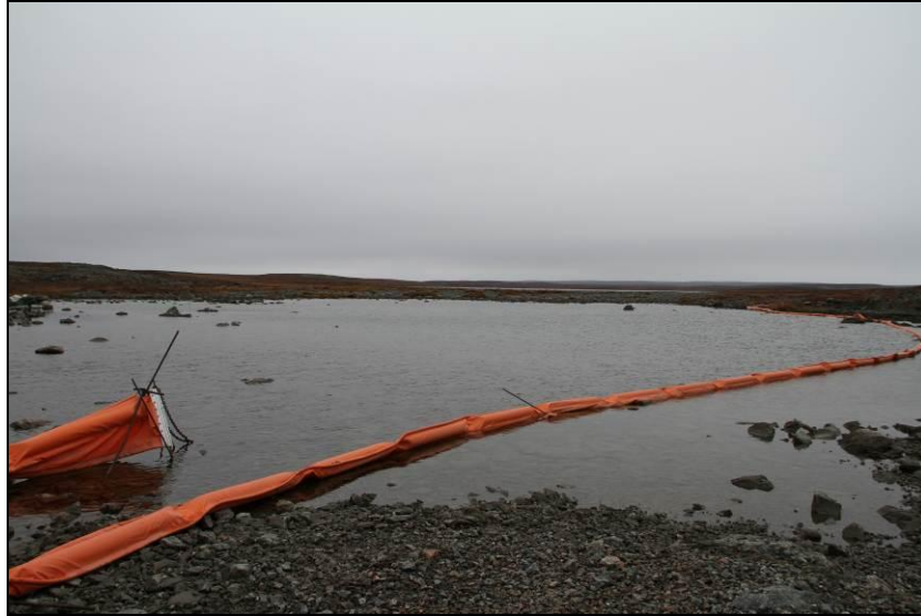
Photo 22: Booms and screens in place at bridge near kilometre 22
