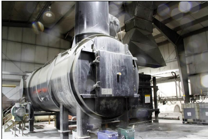
Photo 19: Dual chamber forced air incinerator at the Meadowbank site
