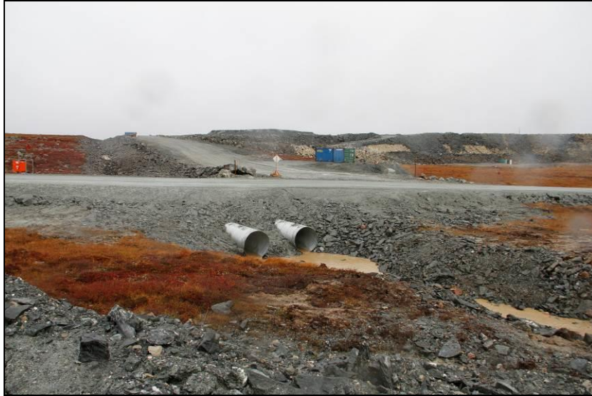
Photo 12: Diversion ditch around tailings facility
