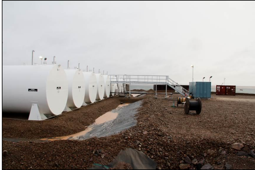
Photo 25: Jet-A pad at Baker Lake storage facility
