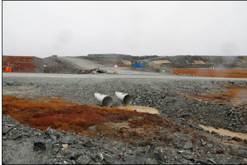
Photo 12: Diversion ditch around tailings facility
