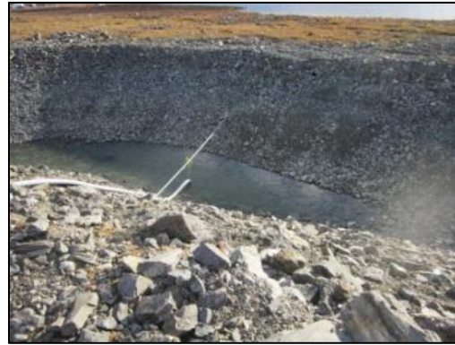
Photo 43: Point of seepage through the road at the Assay lab, located to the bottom right of Photo 42.
