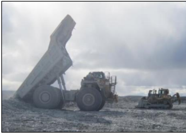
Photo 18: Dumping of waste rock to build the steps in the Vault pit waste rock storage facility.
