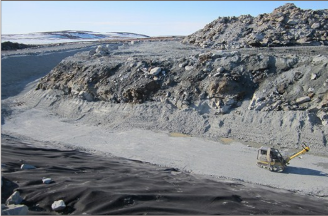
Photo 15: East End of Interception Trench Facing Northwest Bentonite Material on Upstream Slope Below Bedrock Contact
