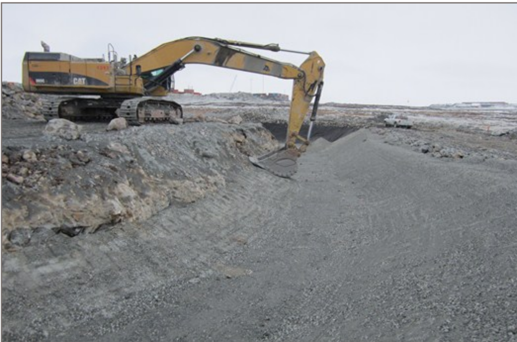
Photo 14: West End of Interception Trench Facing Southeast CAT 365 Excavator Bucket Compacting Upstream Bentonite Material Slope Below the Bedrock Contact
