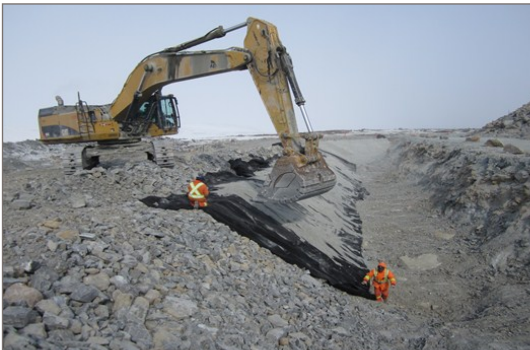
Photo 10: West End of Interception Trench Facing Northwest Trench Bottom after Cleaning. Contractors Laying Geotextile on Downstream Slope
