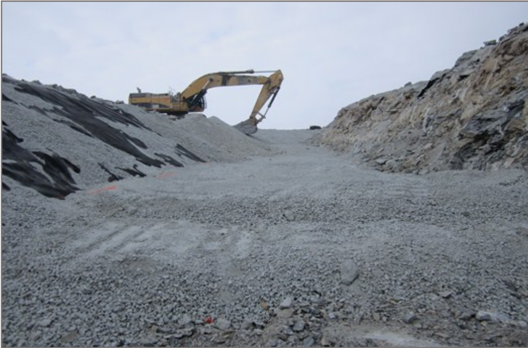
Photo 13: West End of Interception Trench Facing Northwest Background: CAT 365 Excavator Bucket Compacting Two Lifts of Bentonite Material on Downstream Slope. Foreground: Two Lifts of Bentonite Material Visible
