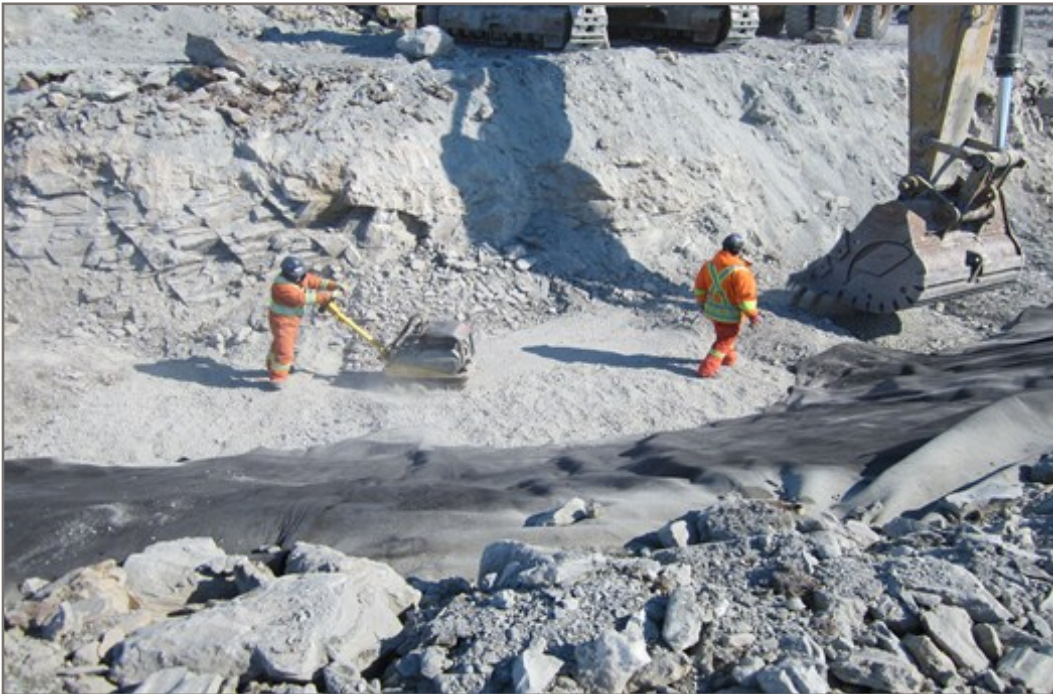
Photo 12: West End of Interception Trench Facing North Contractor Filling in and Compacting Low Areas
