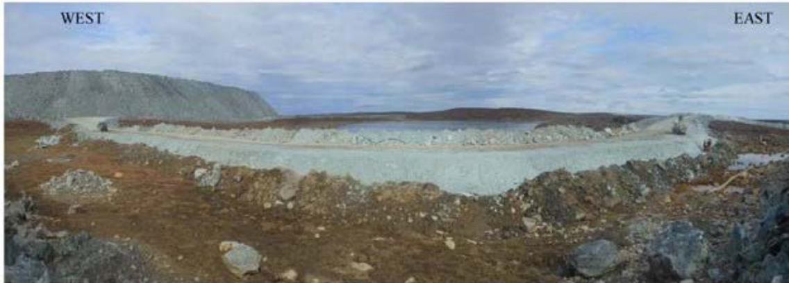
Figure 10: photo of the final result of the entire till plug from West to East. The actual pumping station and the 2 active seepage channels are visible on the eastern abutment.
