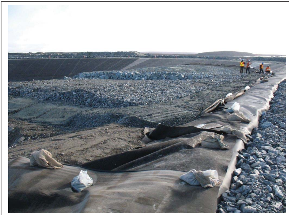
Photo no. 7 Construction of Key Trench Protection at Saddle Dam SD5
