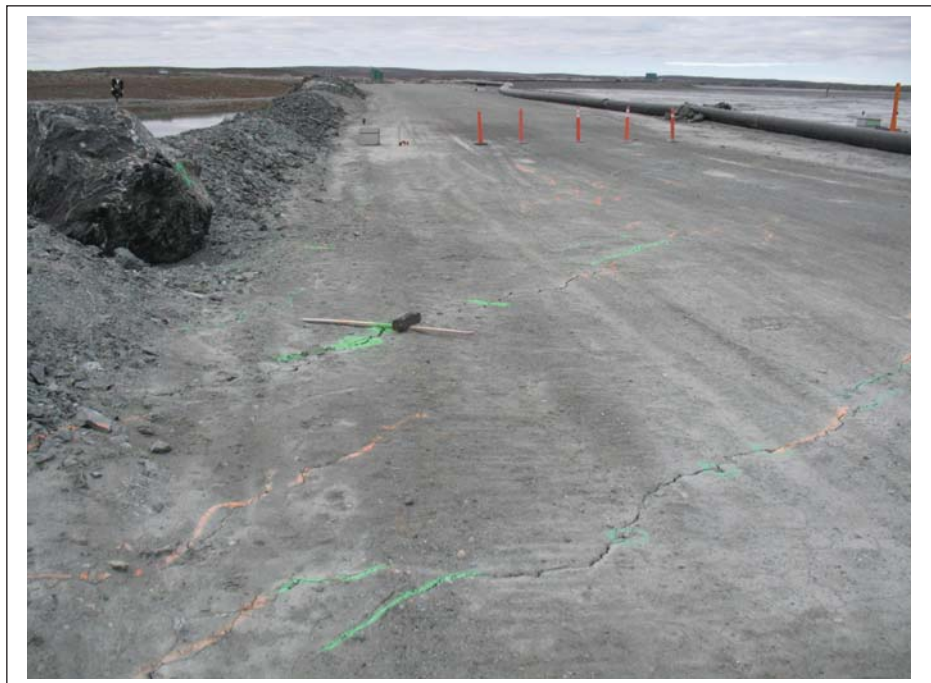
Photo #2 Location of new depression. 70cm max settlement on D/S (left)
