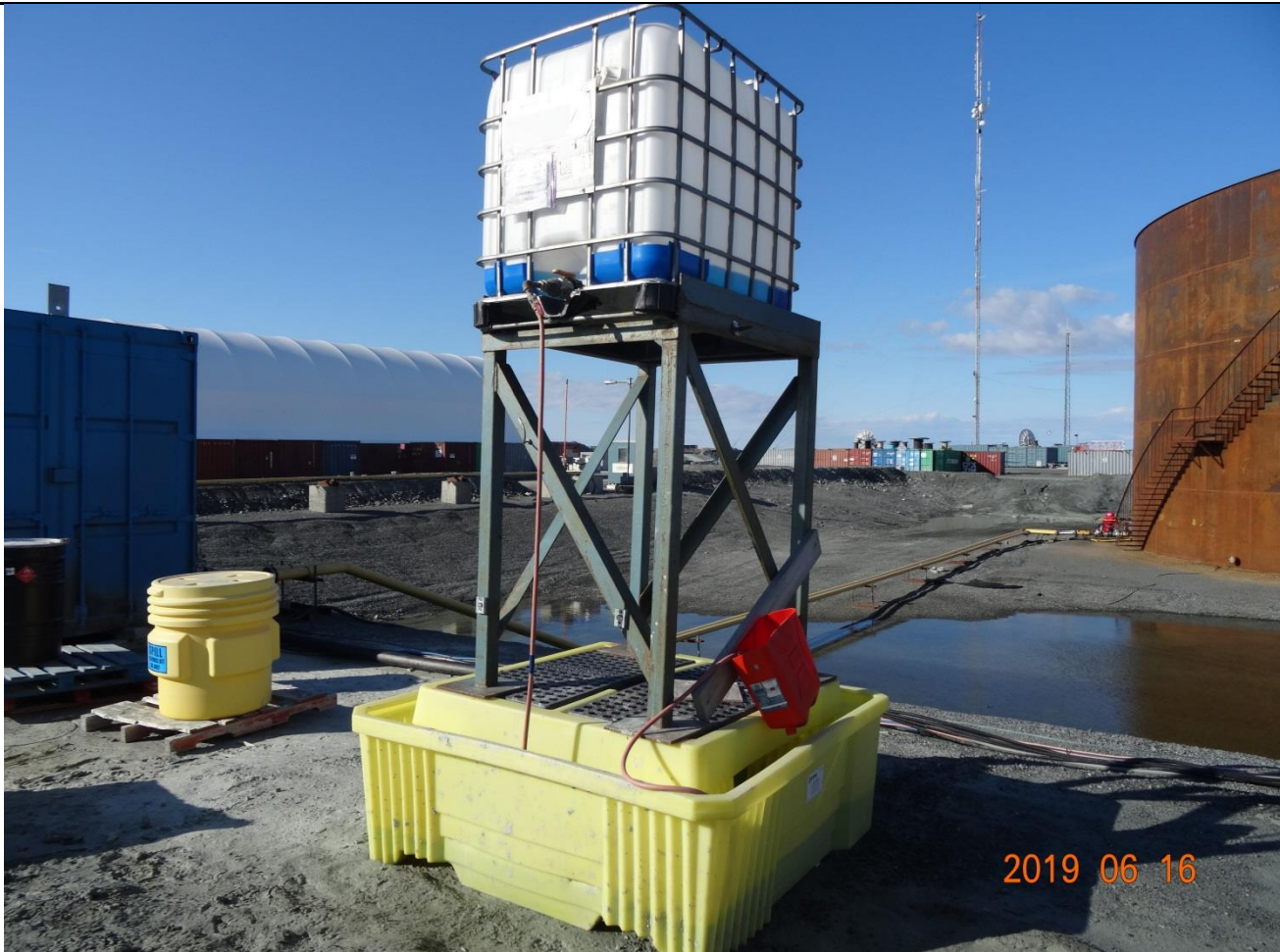
Description: Adequate secondary containment installed at fuelling station
