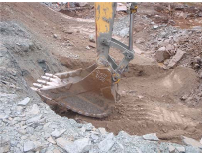
Figure 3: till placement with the excavator bucket and compaction.
