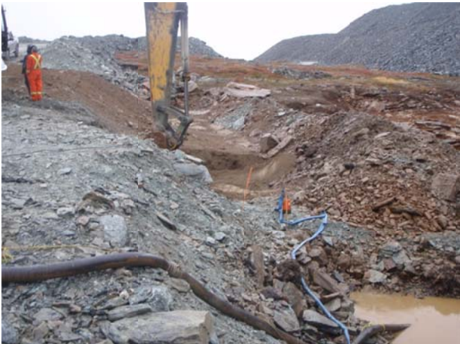
Figure 9: water control during the construction. A small 3" electric pump and a 3" diesel pumps were used.
