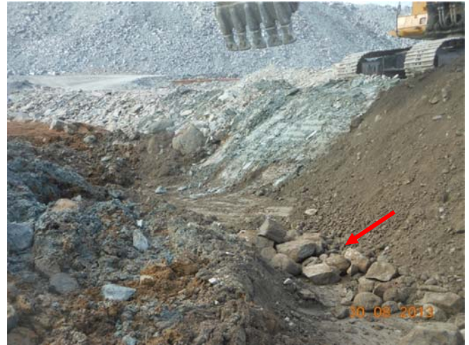
Figure 4: preparation of the transition NPAG on the roadside. Once excavation completed, soapstone was flattened and compacted before any till placement. Note the coarser material discarded from the till (red arrow).
