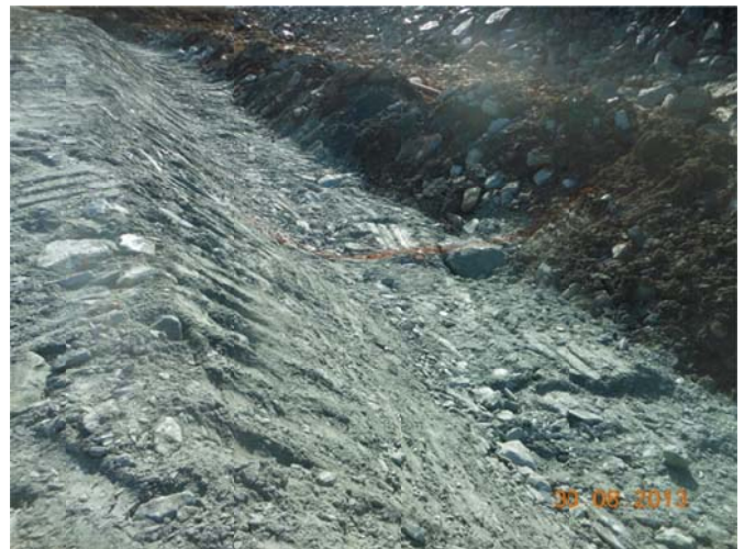
Figure 6: Final placement of soapstone rockfill protective layer (1A) over the till, once compacted.
