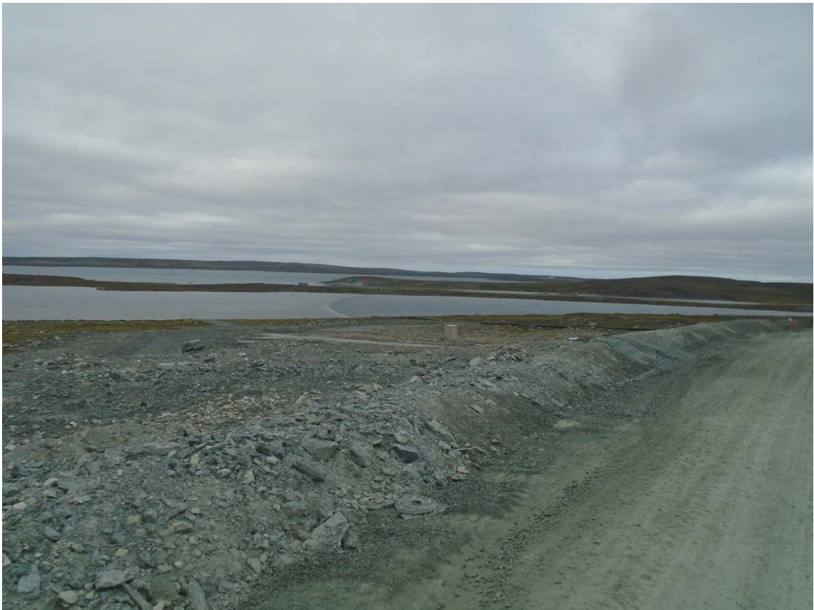
Figure 1: Concerned section of the rock barrier berm that was refilled with material
